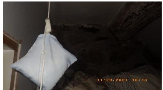
Inside Storage cupboard A
