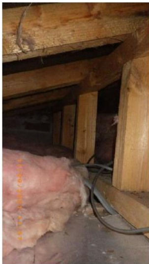
Loft above the west extension
