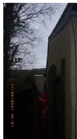
South elevation of the south extension
