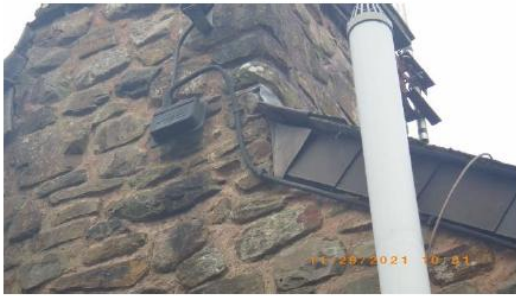
Raised hanging tiles on the south gable
