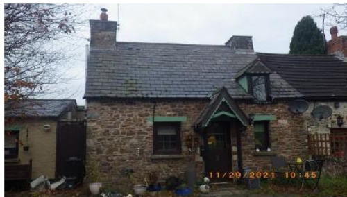
East elevation of the house
