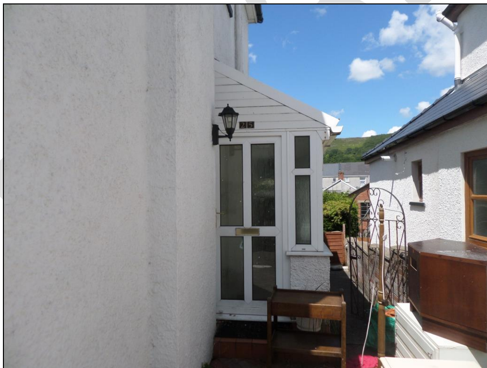
Photo 2: Access porch located on eastern elevation (view looking north).
