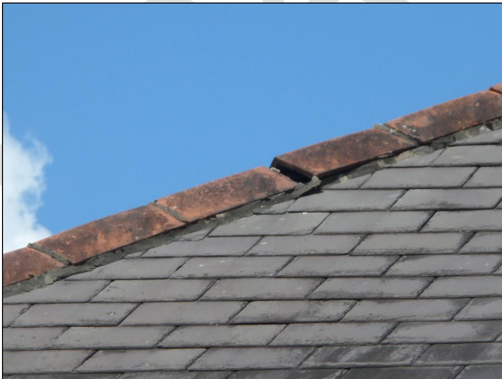
Photo 8: Missing ridge mortar on front of roof (southern elevation).
