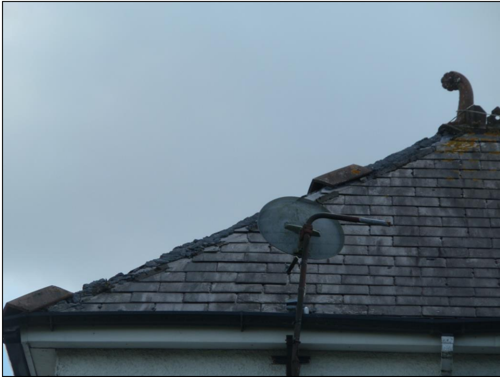
Photo 8: Missing ridge mortar on front of roof (southern elevation).
