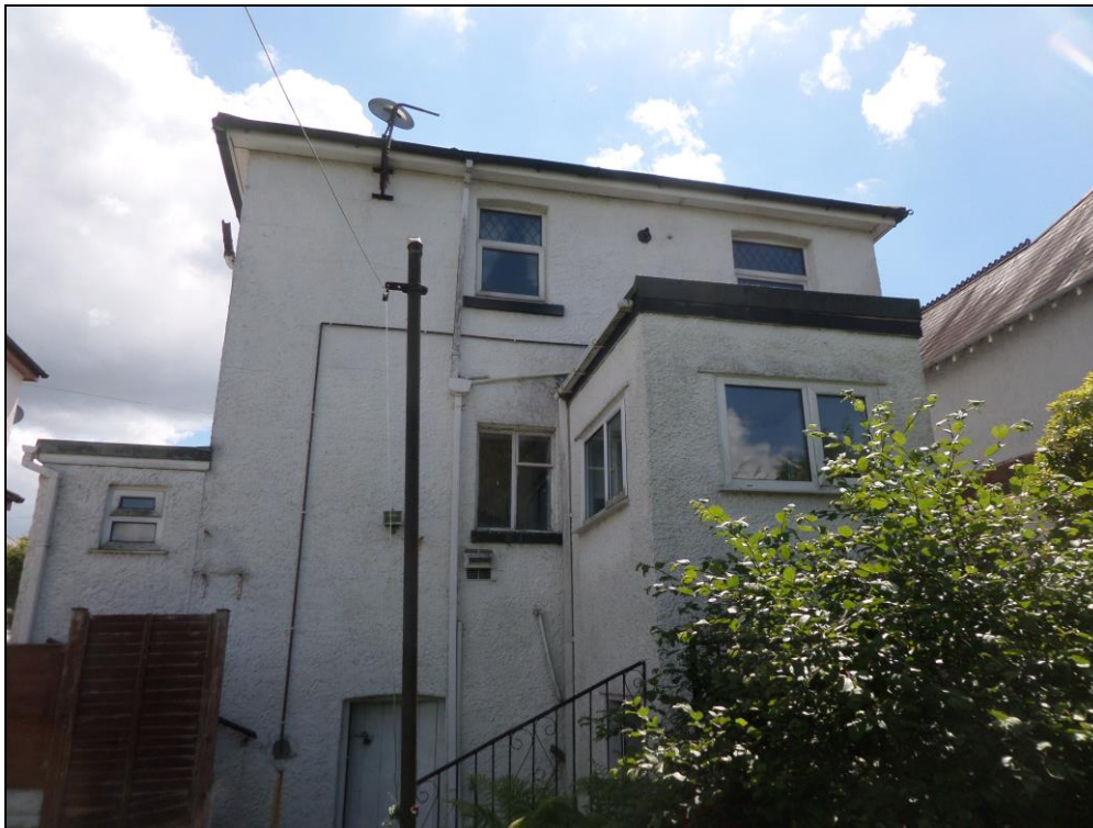
Photo 3: Three storey northern elevation (view looking south).
