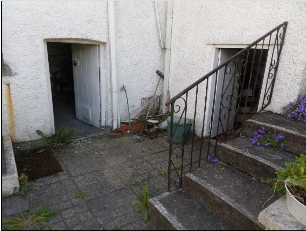
Photo 5: Two ground floor storage rooms (view looking south west).
