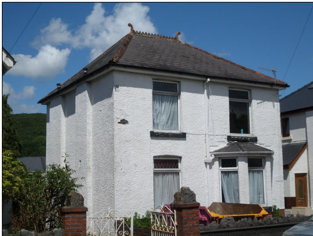
Photo 1: Southern and western elevations (view looking north east).
