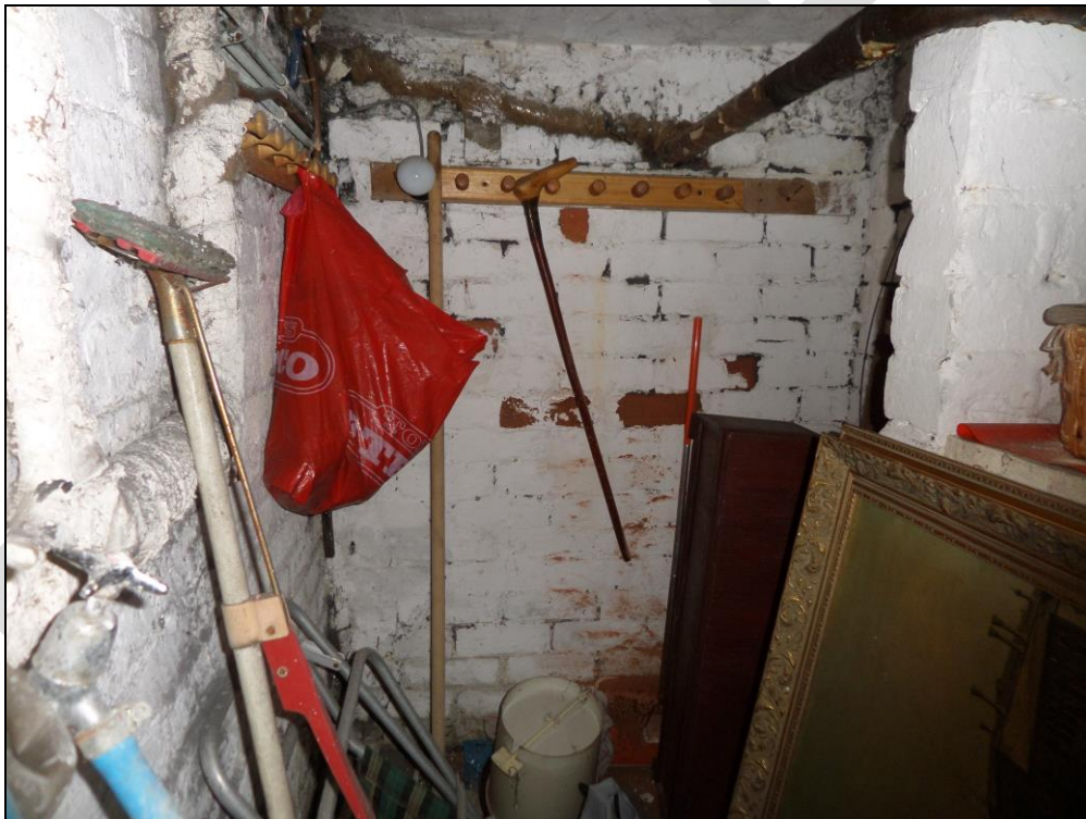
Photo 9: Internal of eastern ground level storage room.
