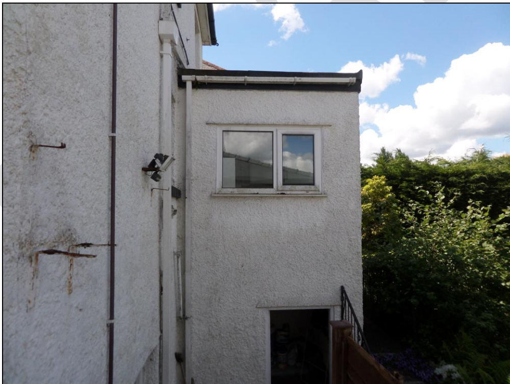
Photo 4: Two storey rear annex on northern elevation (view looking west).
