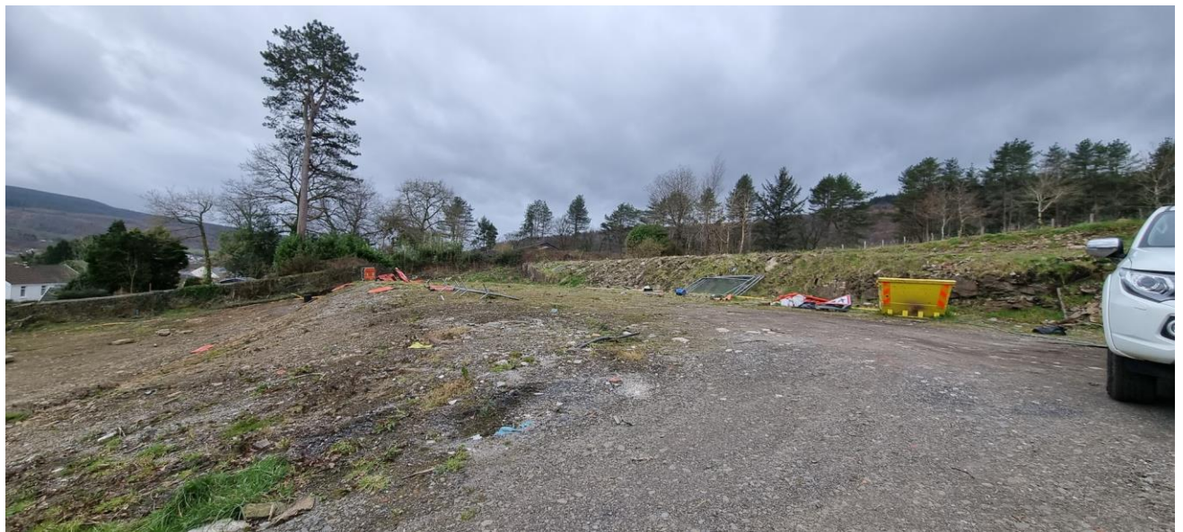
Photo 1: Study area, looking south across development footprint and terrace cutting.
