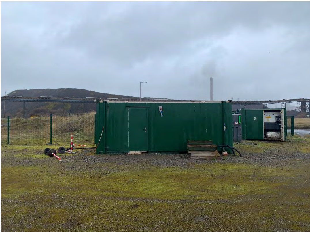
Photograph 2: General site conditions, looking north.
