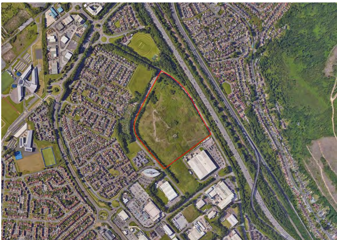
Image EDP 2.1: Aerial photography extract of the site, identified by redline boundary.
