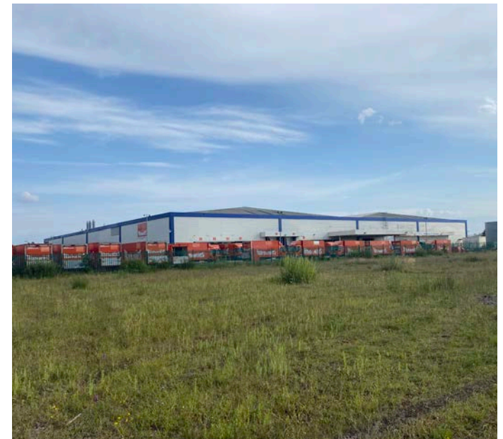
Figure 17 - Warburtons factory to the south of the site
