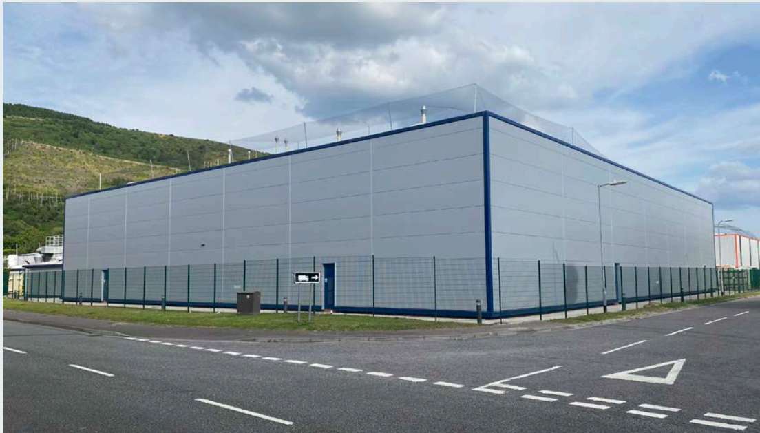
Figure 20 - Existing industrial unit at Baglan Industrial Park
