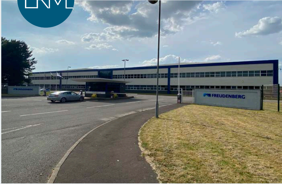
Figure 18 - Existing industrial unit at Baglan Industrial Park
