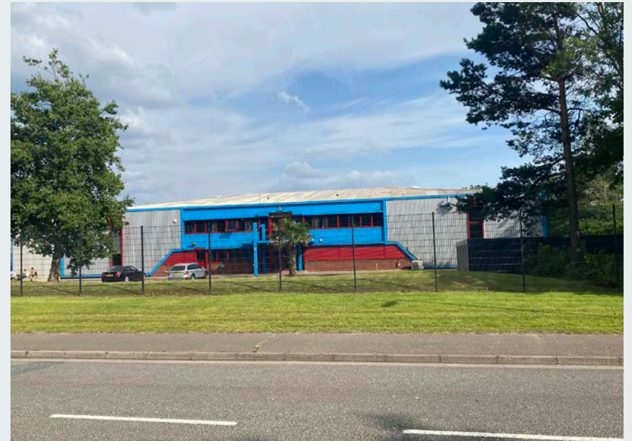
Figure 21 - Existing industrial unit at Baglan Industrial Park
