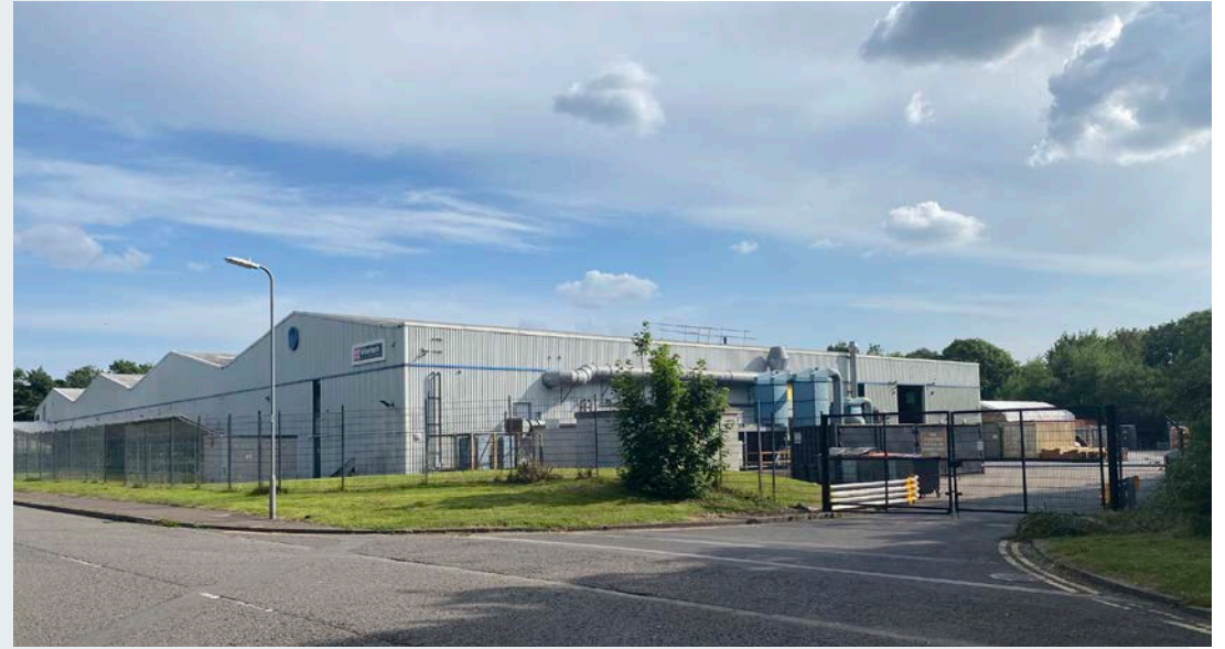
Figure 19 - Existing industrial unit at Baglan Industrial Park
