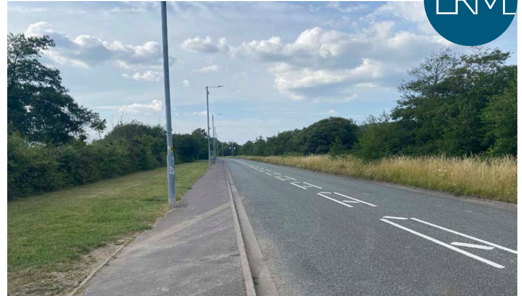
Figure 9 - Baglan Way to the north-east of the site
