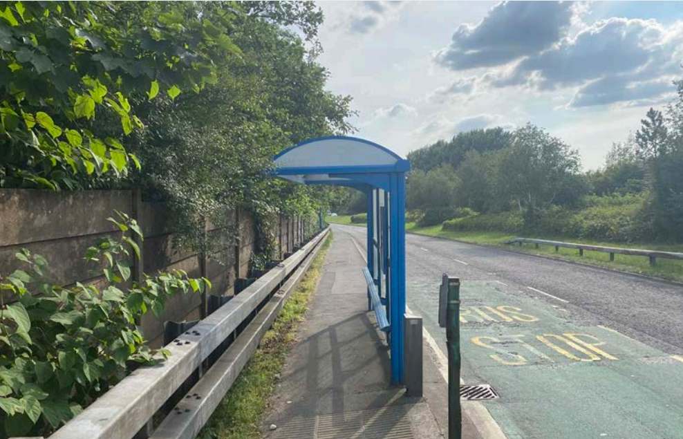
Figure 13 - Bus shelter near Baglan station on the A4241
