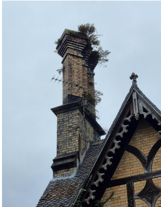
Fig.10 Chimney foliage growth (South Elev)
