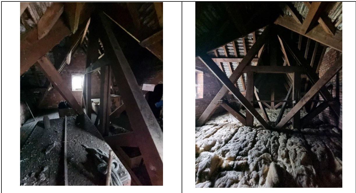
Fig.8 North attic space
