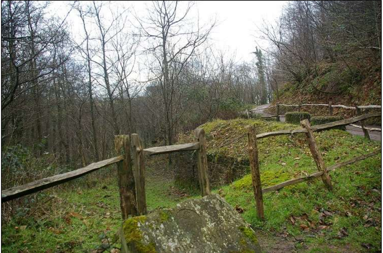
11. THE MONKS BATH, MEDIEVAL CISTERN AND BASIN, LOCATED IN THE WOODED VALLEY BEHIND THE ABBEY, LATER ADAPTED AND EXTENDED AS A FOLLY WITHIN THE REMODELLED PARKLAND; VIEWED FROM THE NORTH.
