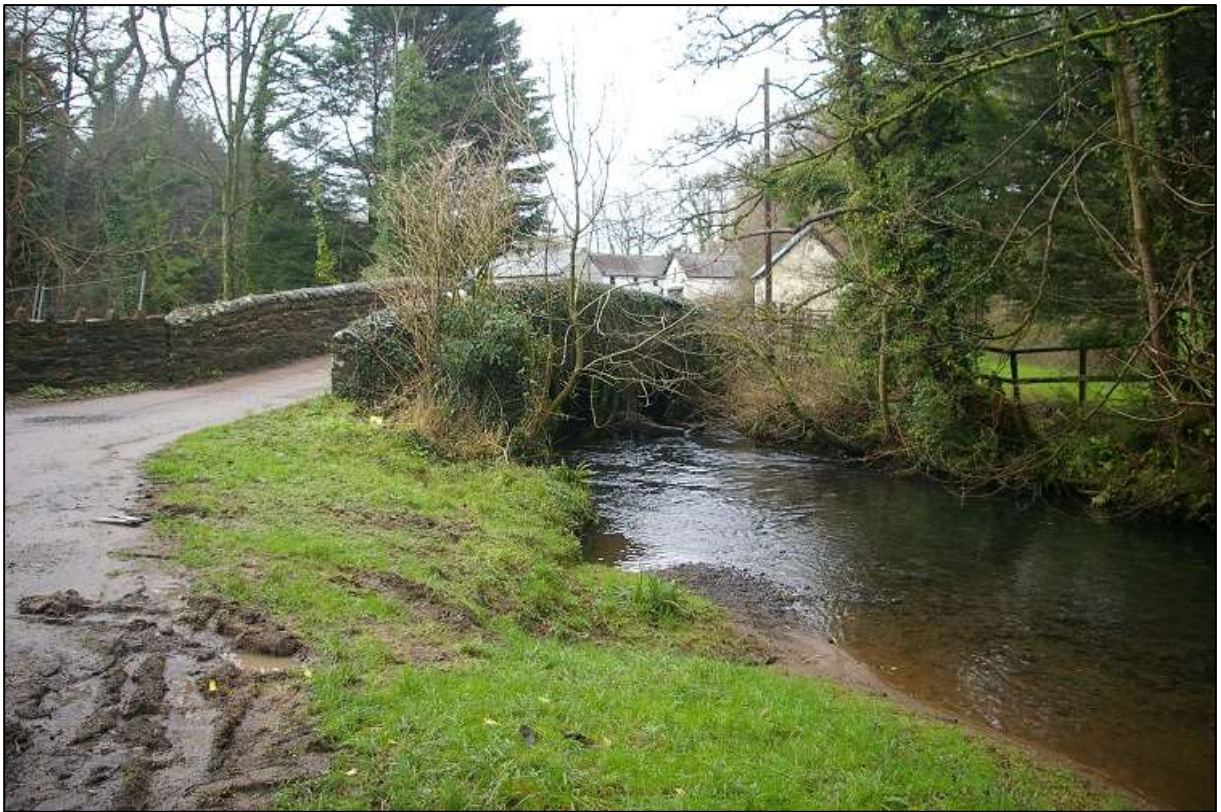
2. LLANMIHANGEL BRIDGE, LEADING TO THE MILL AND FARM; VIEWED FROM THE SOUTH-EAST.
