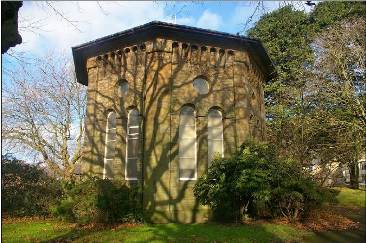
FIGURE 33: BULAH CALVINISTIC METHODIST CHAPEL IN ITS CURRENT LOCATION, A PARK IN THE MODERN SUBURBS OF PORT TALBOT; VIEWED FROM THE SSW.
