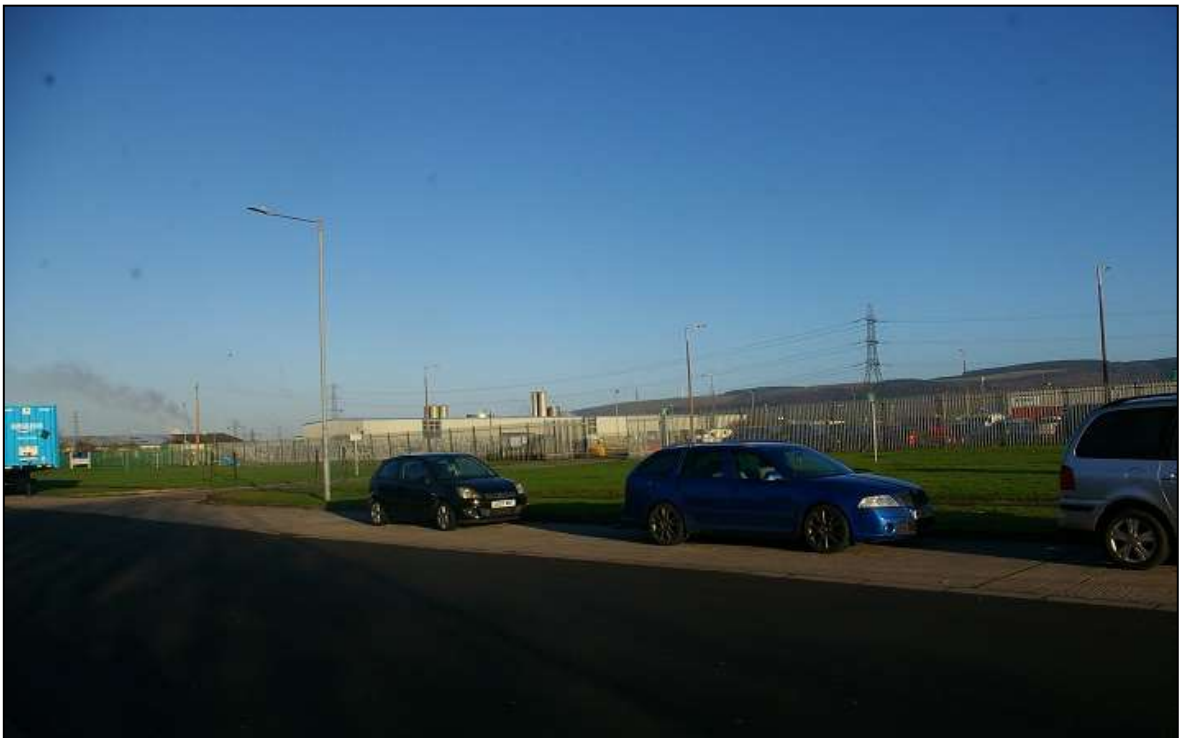
FIGURE 7: THE SITE OF THE PROPOSED TURBINE ON THE KENFIG INDUSTRIAL ESTATE; VIEWED FROM THE SOUTH-WEST.
