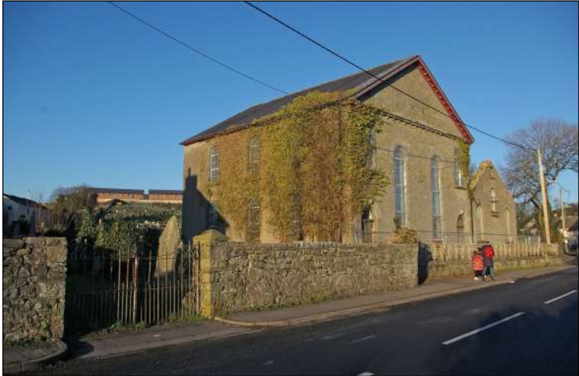
FIGURE 32: PYLE CALVINISTIC METHODIST CHAPEL; VIEWED FROM THE WSW.
