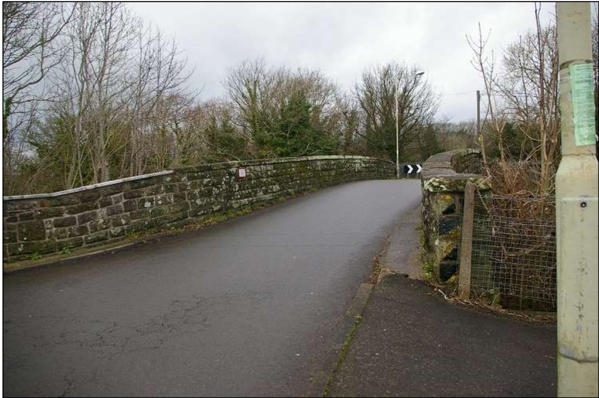
FIGURE 18: PYLE ROAD OVERBRIDGE; VIEWED FROM THE WSW.
