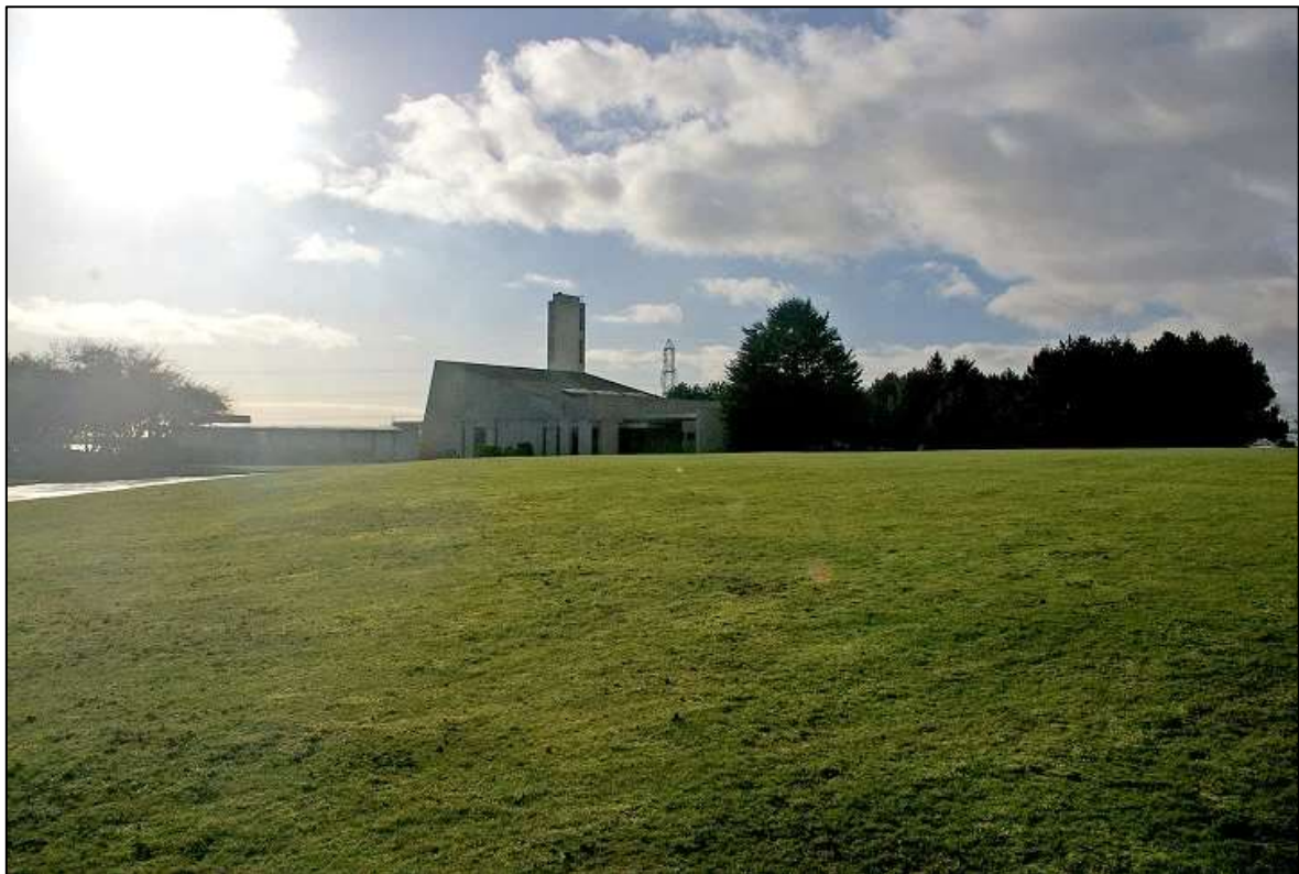
FIGURE 24: MARGAM CREMATORIUM, A STRIKING MODERNIST BUILDING CONTAINED WITHIN ITS OWN PARKLIKE SETTING, FRAMED BY TALL HEDGES; VIEWED FROM THE NORTH-EAST.
