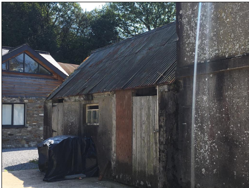
Photo 5: Northern annex elevation with gaps above doors and open window (view looking east).
