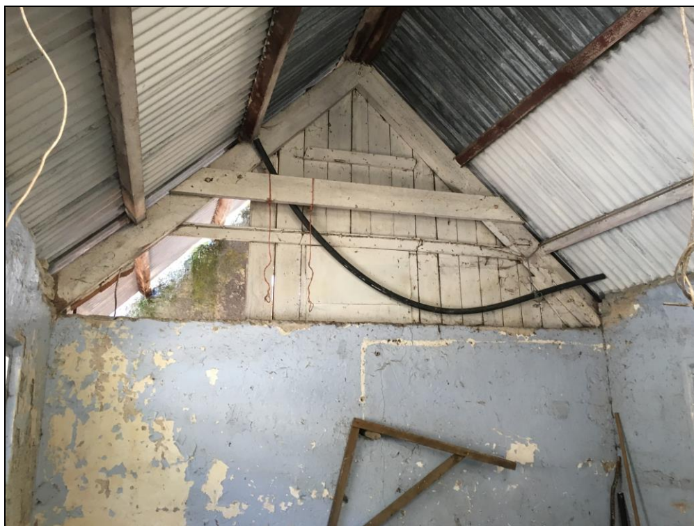
Photo 13: Interior of annex (view looking east).
