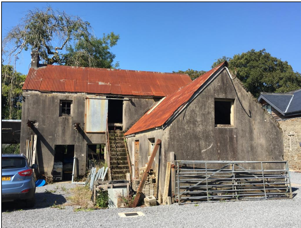
Photo 1: Main cottage structure and annex eastern elevations (view looking west).
