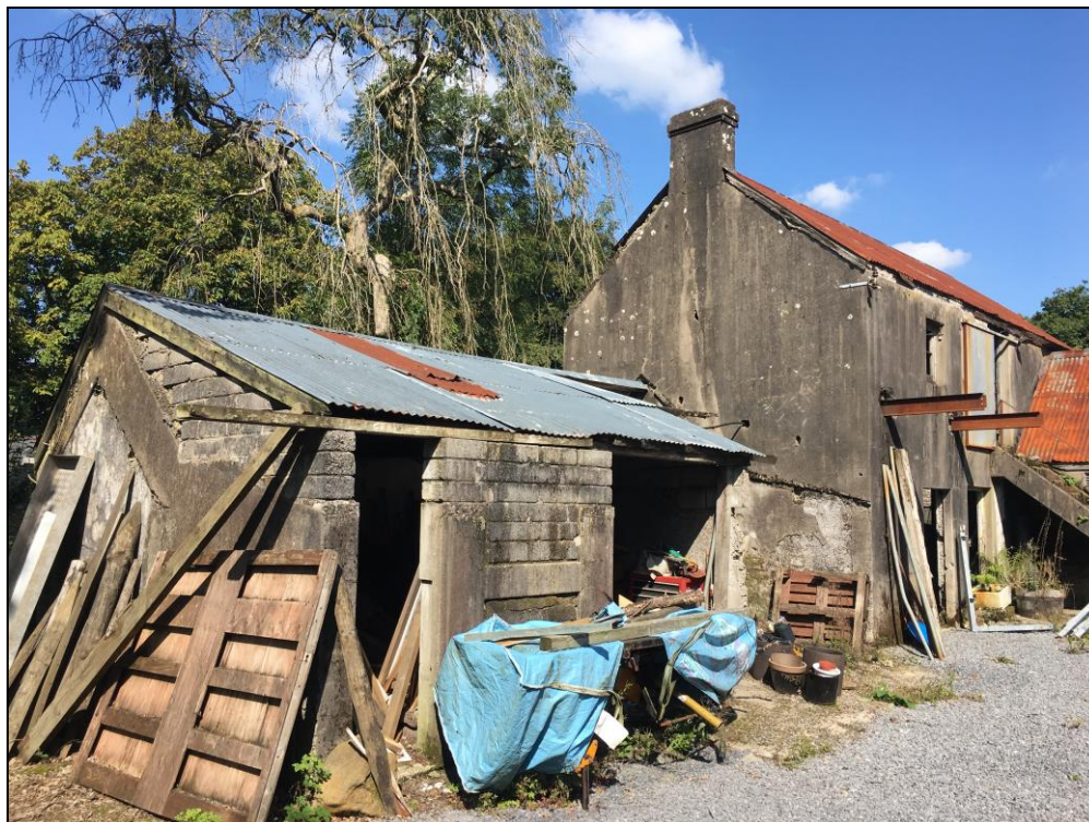
Photo 14: Storage shed (view looking west)
