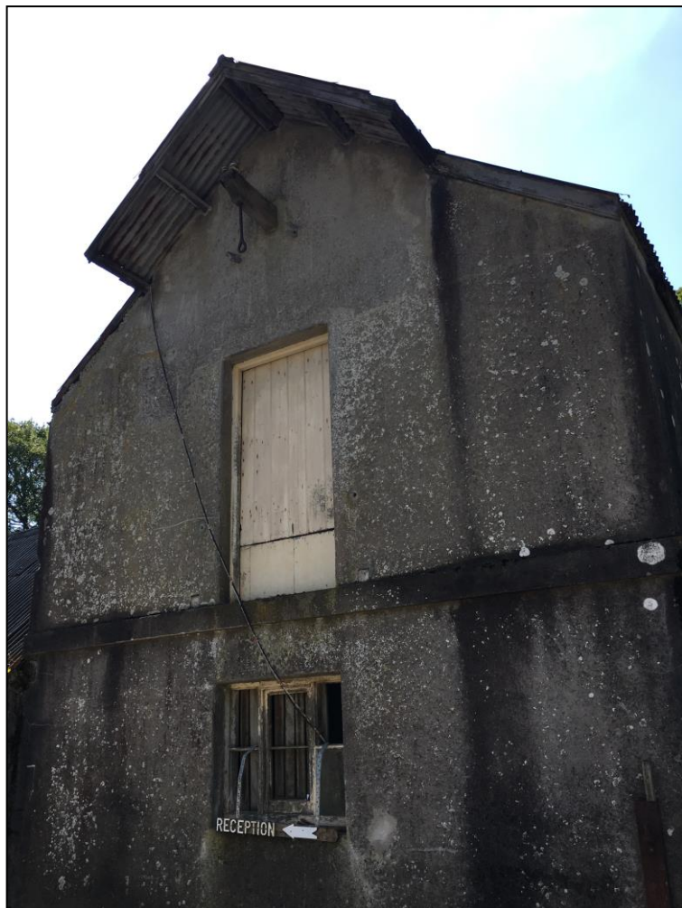
Photo 5: Northern annex elevation with gaps above doors and open window (view looking east).
