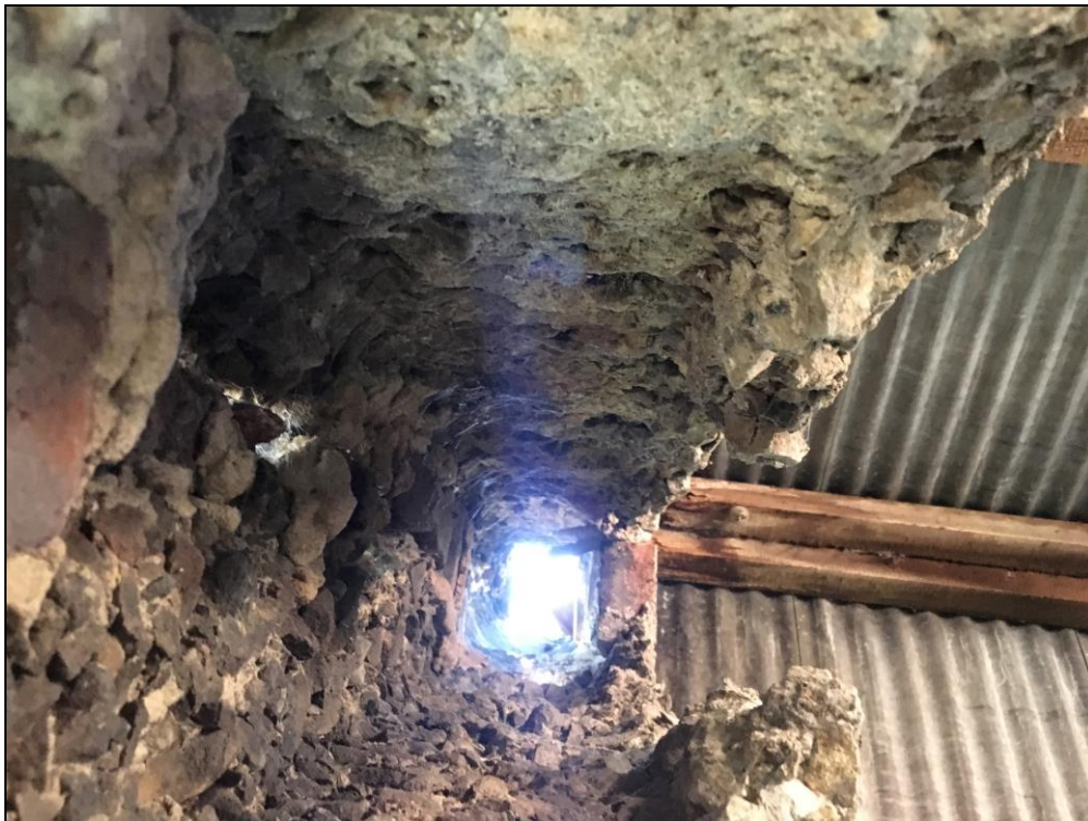
Photo 12: Interior of chimney breast through crack in wall.
