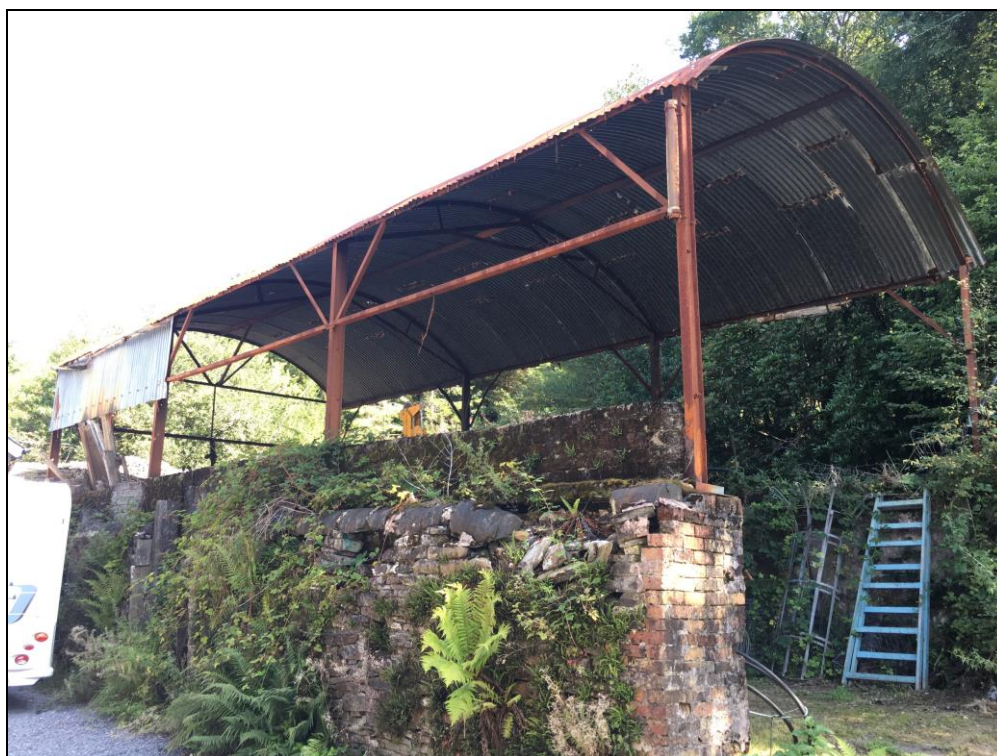
Photo 15: Dutch Barn (view looking east).
