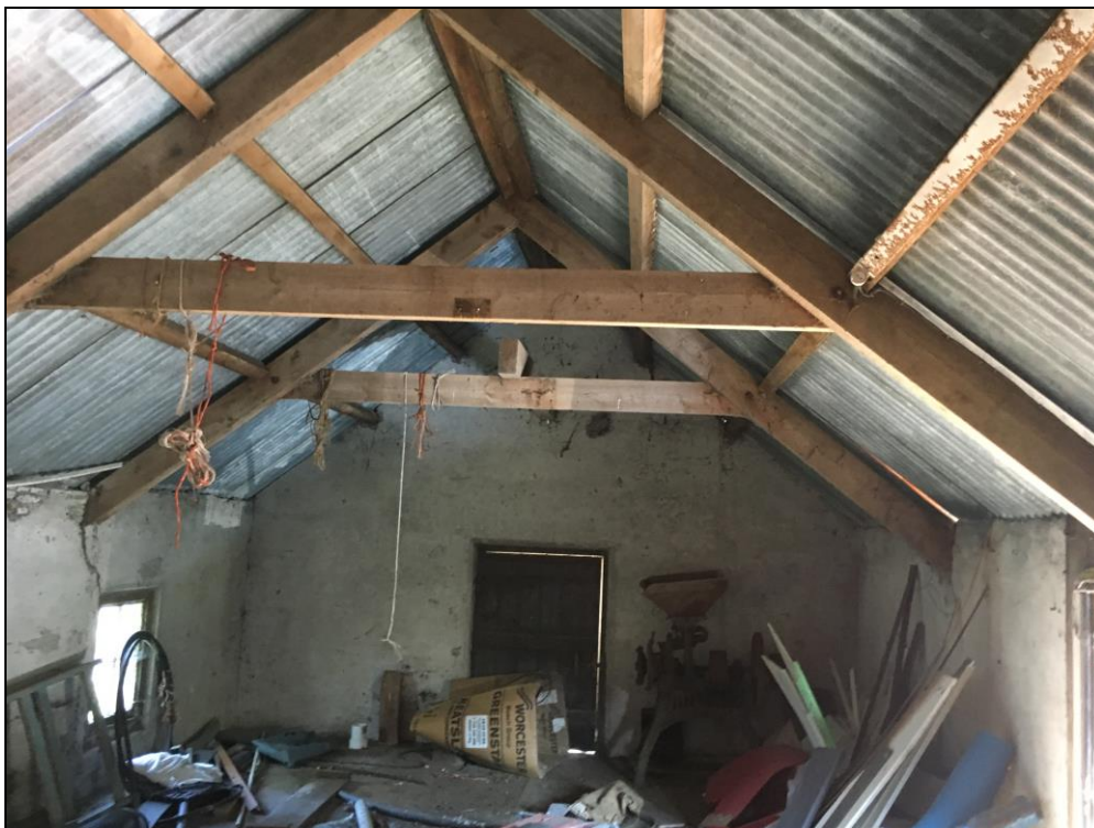
Photo 9: First floor interior (view looking north).
