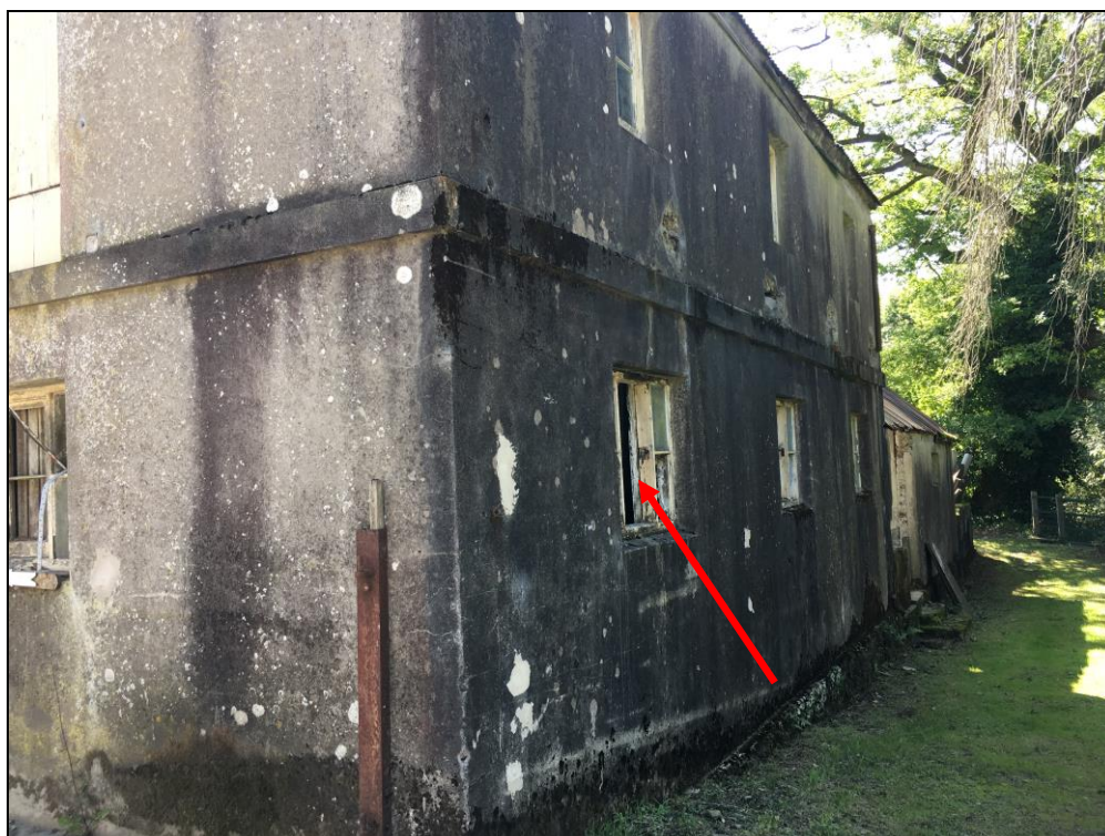
Photo 18: Emergence from open window (view looking south).
