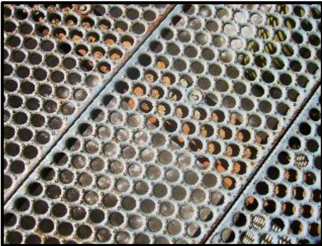
Metal grate treads fixed over existing concrete treads
