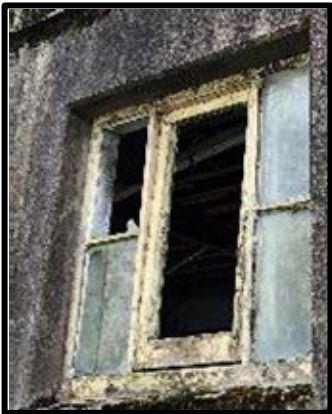
Photographs of existing typical timber windows which have deteriorated considerably and are deemed beyond reasonable repair
