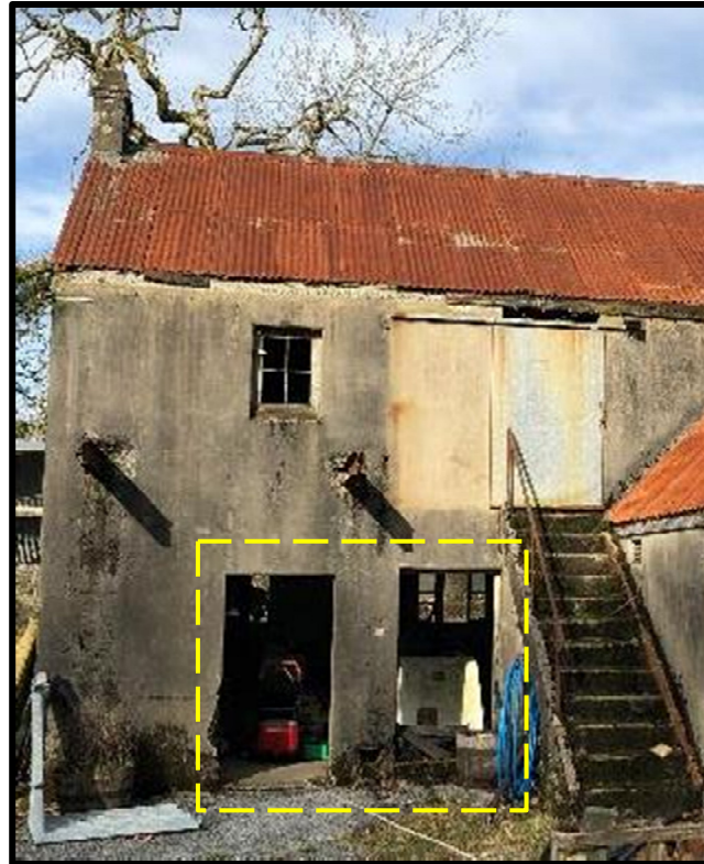
Photo of existing openings which do not currently have doors or windows within them
