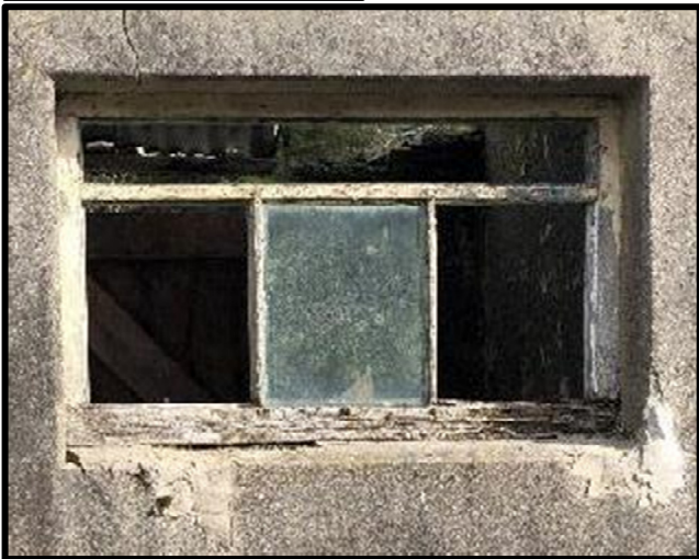
Photographs of existing typical timber windows which have deteriorated considerably and are deemed beyond reasonable repair
