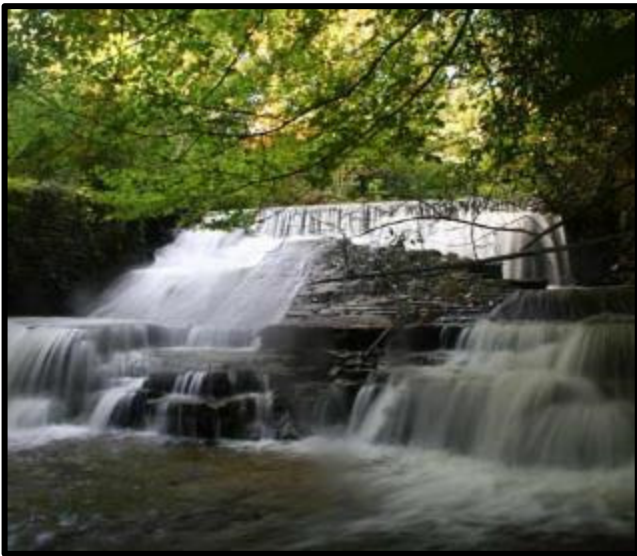
Recent photograph of the Weir at Plas Farm
