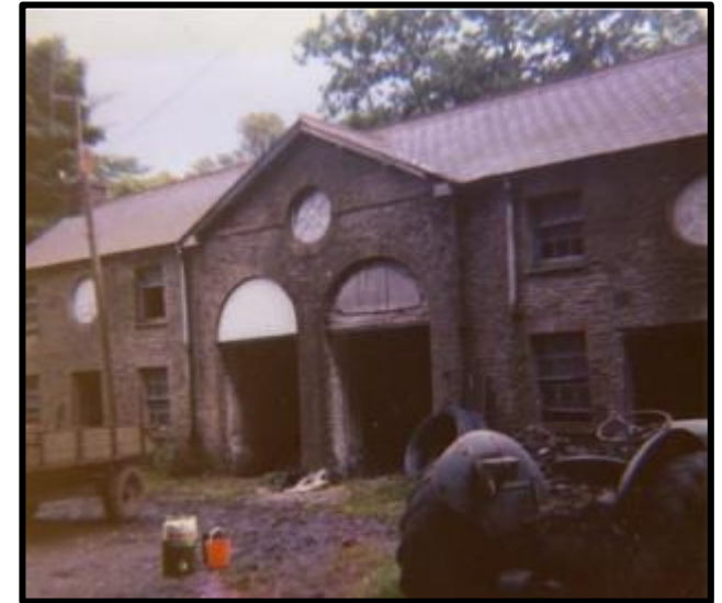
Photograph of the Georgian Coach House (now converted to 'Y Stabl' and 'Ty Cerbyd') taken in the 1960's
