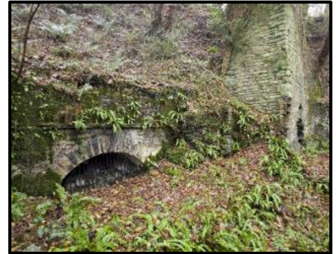
Structures that form part of Waun y Coed Colliery Branch Canal & Tramroad Incline (Scheduled Ancient Monument) Source: RCAHMW
