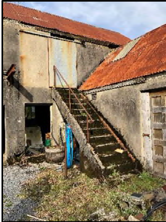
Photo of existing stair and balustrade
