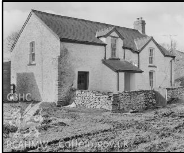
Early 20 th Century Photograph Cefn Celfi (Listed Building) prior to mid-20 th Century alterations Source: RCAHWW
