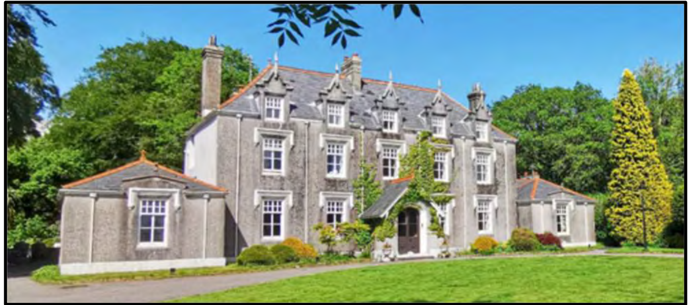
Victorian South-facing Front Elevation to Plas Cilybebyll
