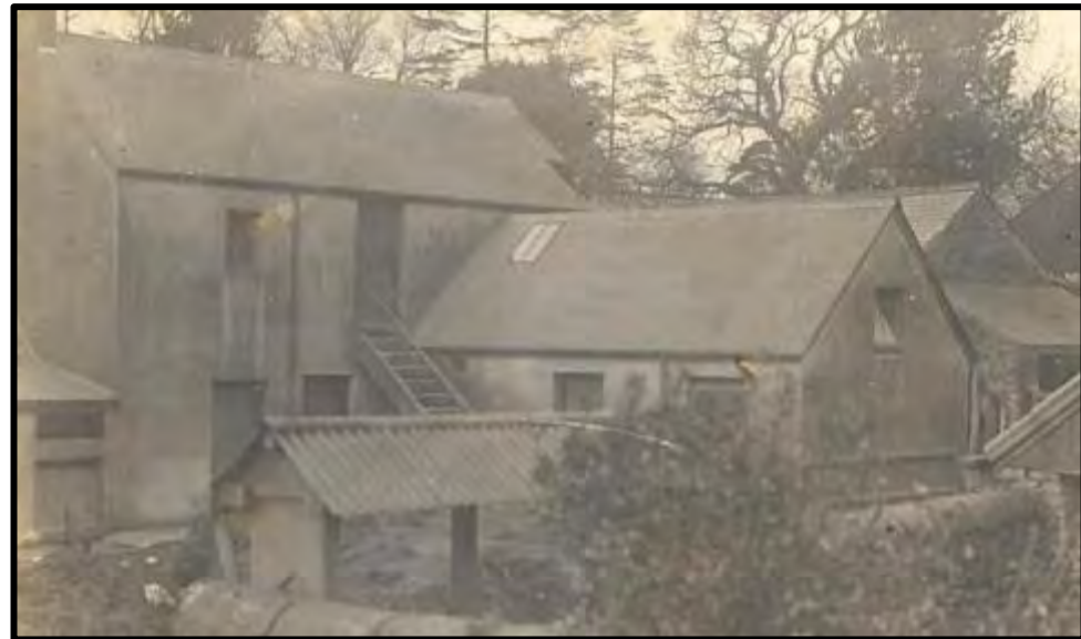
Top & Bottom Right: The building from circa 1900, demonstrating the original design and finish of the building. Mass concrete with a plain cement render, gable chimney and corrugated sheet roof. Tripart windows to ground floor, a loading door and hoist to first floor on the South gable with a projecting roof
