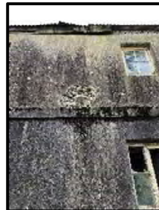
Photograph of existing typical façade to be restored highlighting necessary repair, cleaning and recoating
