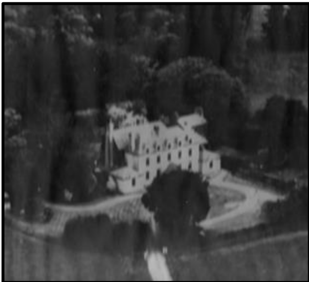
Aerial View of the 'Plas' taken from a Lancaster Bomber during a WWII training flight, clearly showing the rear wing's roof (demolished 1955)
