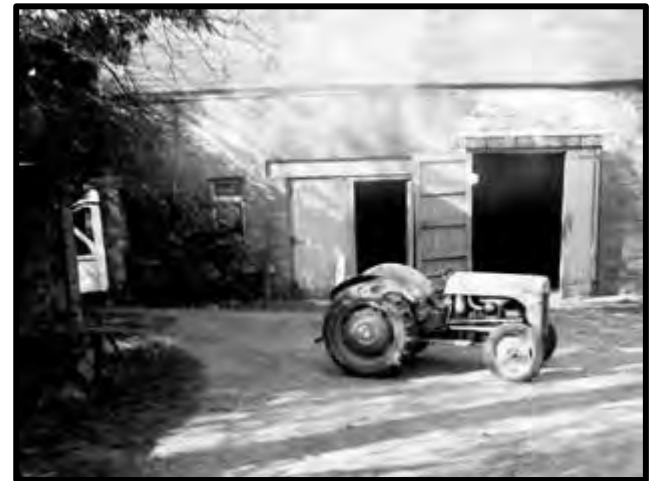
Photograph of stable taken in 1958 that has now been converted into 'Hafod y Wennol' Holiday Cottage clearly showing traditional materials used in its construction
