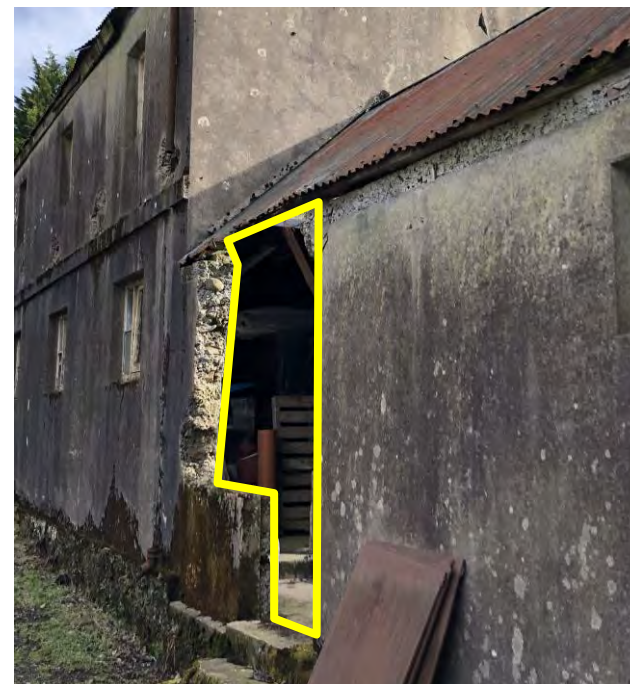
Photo of existing opening. New aluminium frame fixed window to be fixed behind and independently of the existing opening
