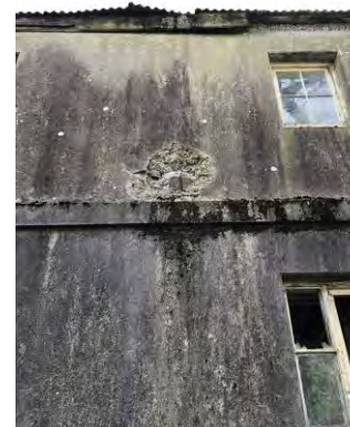
Photo of existing typical façade to be restored highlighting necessary repair, cleaning and recoating
