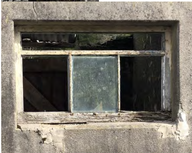
Photo of existing typical timber windows which have deteriorated considerably and are deemed beyond reasonable repair
