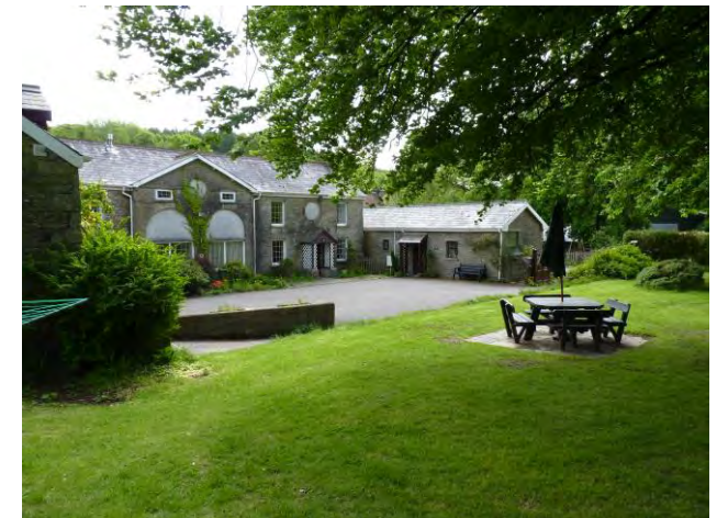
Views of the existing Plas Farm
