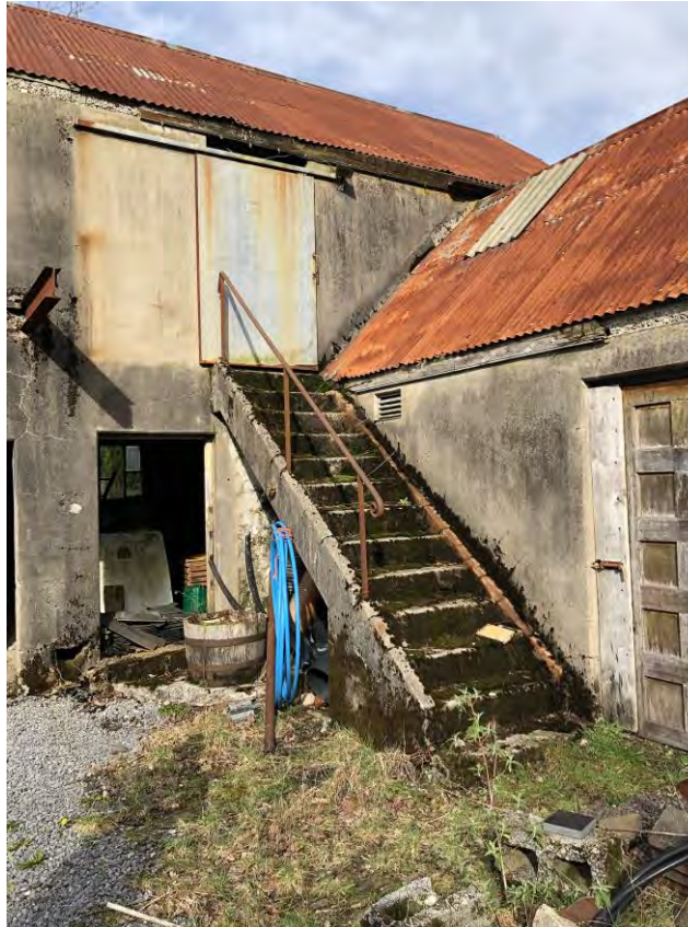
Photo of existing stair and balustrade
