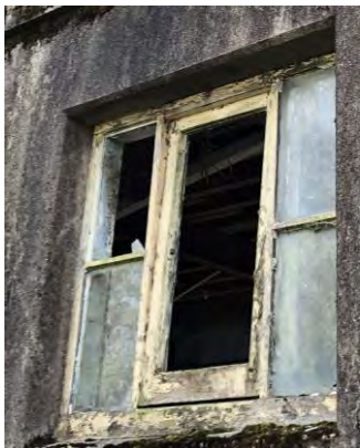
Photo of existing typical timber windows which have deteriorated considerably and are deemed beyond reasonable repair
