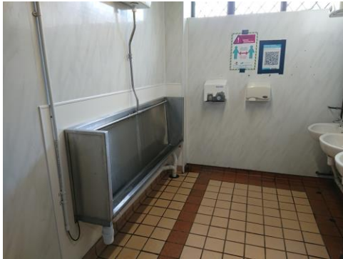
Existing Urinal and Hand Dryers
