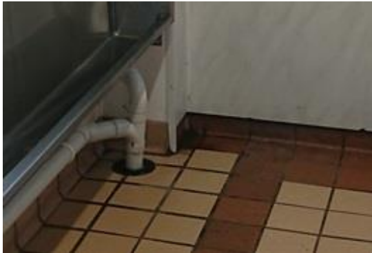
Existing Timber Waste Outlet at Floor
