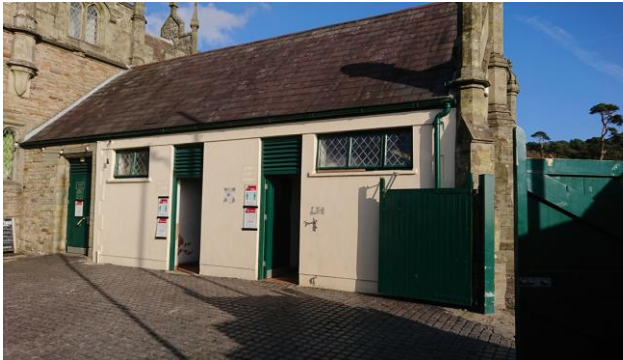
Existing Courtyard Toilets, Front Elev.
