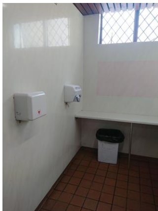
Existing Vinyl Wall Covering
