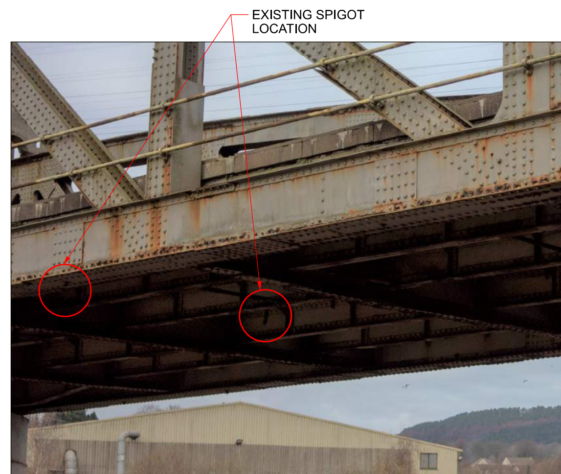
PHOTO - EXISTING SPIGOT
