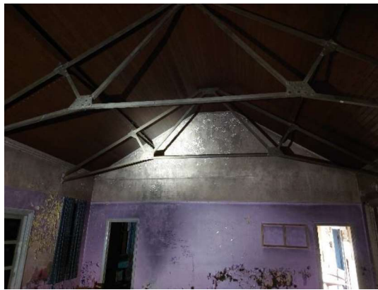
Photograph 2: Interior roof space
