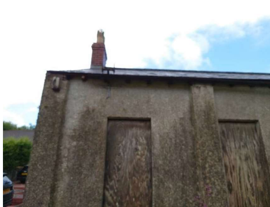
Photograph 4: Chimney on the central roof and windows boarded up.
