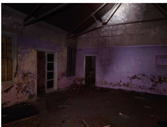
Photograph 5: Interior showing intact window frames.
