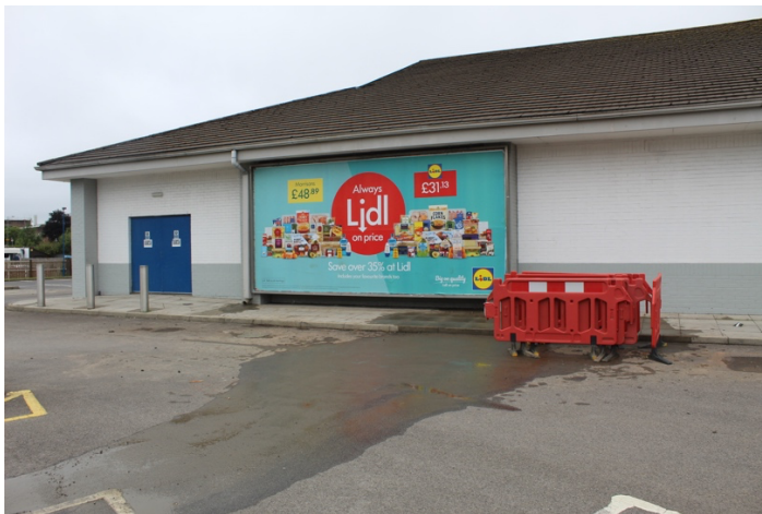
Photo 2: View westwards of the eastern façade of the existing Lidl store building in July 2020.
