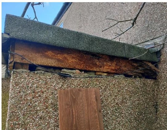
Plate 15: Missing fascia boards on flat-roofed section
