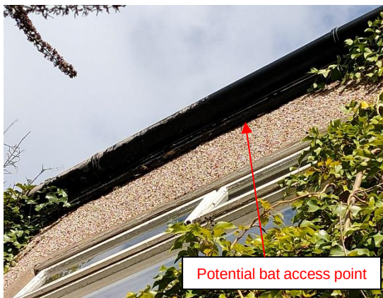
Plate 15: Missing fascia boards on flat-roofed section
