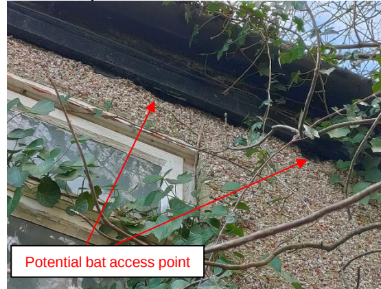
Plate 12: Gaps at barge boards on western gable 2
