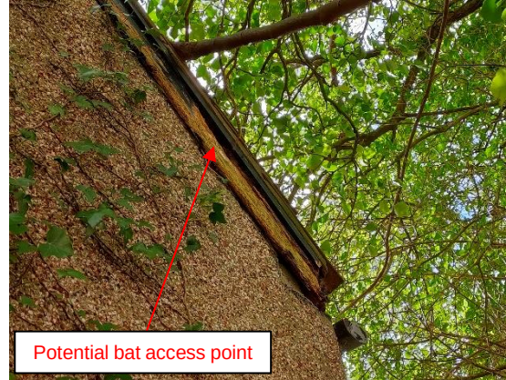
Plate 14: Holes in the flat-roofed section attached to the eastern gable
