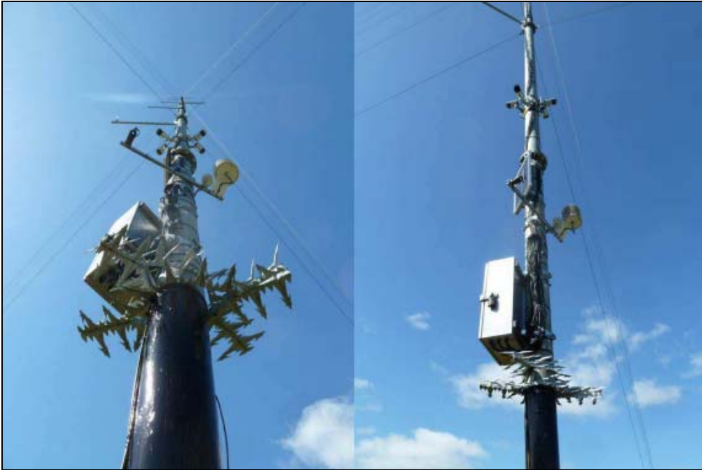
Photo 3: Security spikes, anti- climb paint and security cameras
