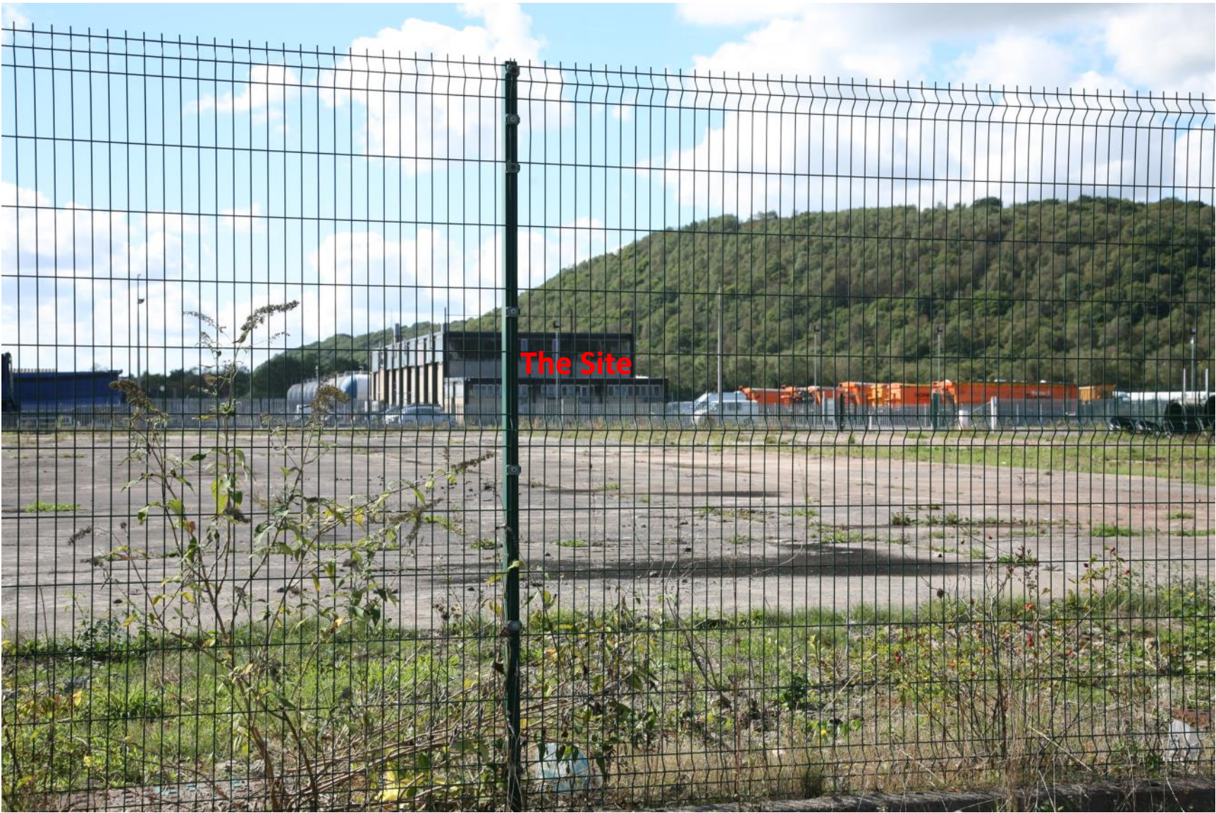
VP2 View of the proposed development site from the estate access road at the SE corner of the FE Site. The existing offices and workshop building will be retained and refurbished as part of the proposed development. Note the high wooded hills which form the backdrop to the FE Site to the W and NW between Llandarcy and Jersey Marine
