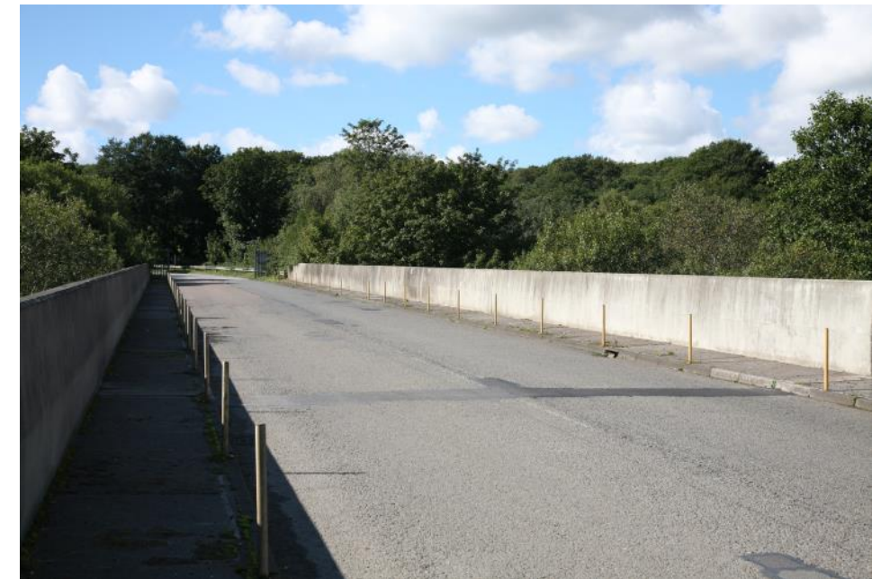
View NW from the access road bridge leading into the FE Site showing the wooded high ground of the Gelli-Bwch Hills between Llandarcy and Jersey Marine
