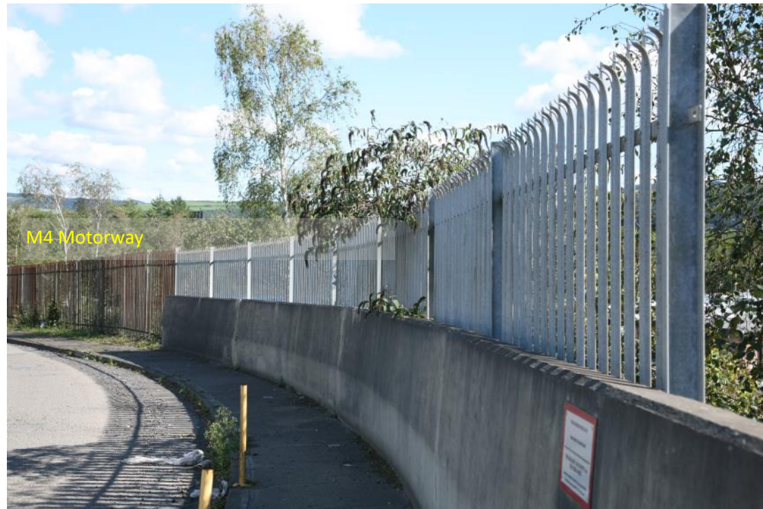
View to the left, showing the FE Site perimeter security fence. Part of the wooded embankment of the M4 Motorway can be seen in the left hand middle ground
