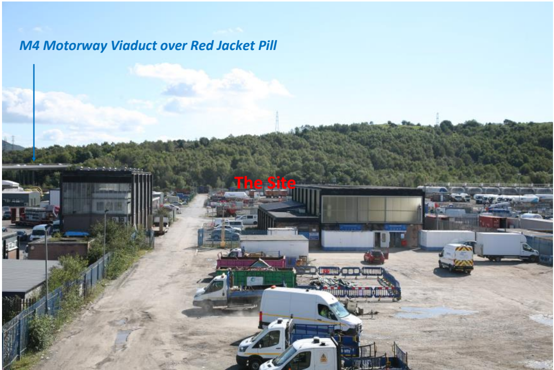
View S into the FE Site from the eastern end of the access road bridge over the Tenant Canal and the railways. The M4 Motorway viaduct over Red Jacket Pill can be seen in the far left hand middle ground of this view. The large above-ground gas storage tanks in the SW section of the FE Site are seen in the far right hand middle ground. The existing offices and workshops building within the proposed development site is obscured by the intervening building in the centre right of this view
