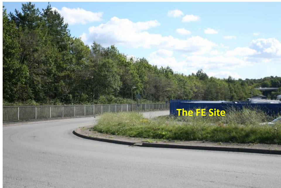
M4 Motorway embankment adjacent to the NW boundary of the FE Site
