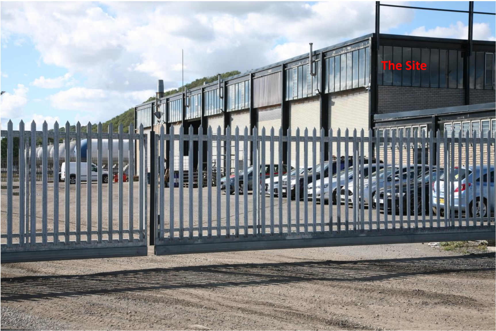
VP1 View of the existing offices and workshops building from the adjacent estate access road. This will be retained and refurbished as part of the proposed development. The very large above-ground gas storage tanks located in the SW section of the FE Site can be seen in the left middle ground of this view, beyond the proposed development site boundary fence
