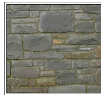
Example of pennant stone cladding to highlighted elevations
