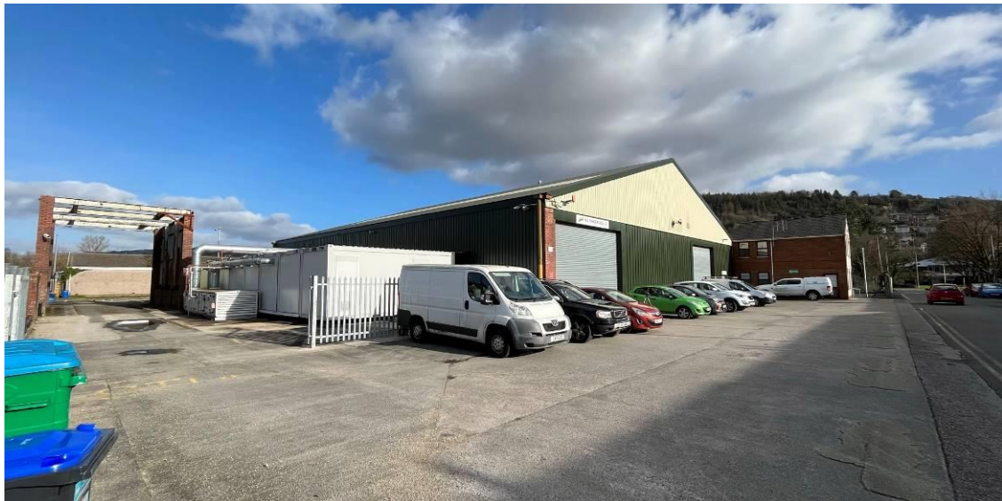
Figure 6.2 – Brother Engineering Site
