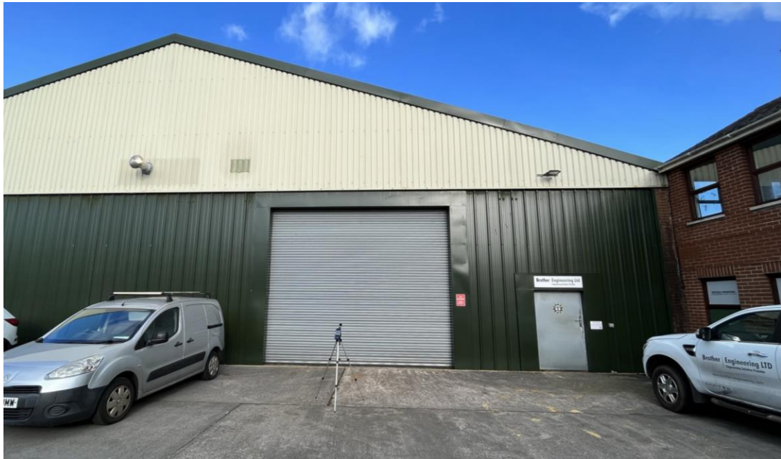
Figure 6.3 – Front SW Façade – Critical Roller-Shutter Door
