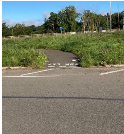
Photo 2-12 - Uncontrolled crossing point across B4290 leading to Coed Darcy business park
