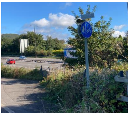
Photo 2-36 - First indication of path status - segregated route signage half-way along link (shared signage is on the reverse)
