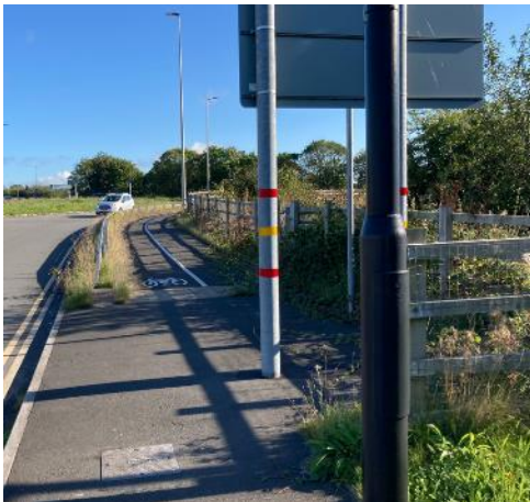
Photo 2-7 - Shared/segregated connection hampered by alignment issues and street furniture
