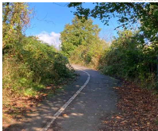
Photo 2-37 - Windy and steep section of the segregated route. There is poor visibility on the bend due to overgrown vegetation
