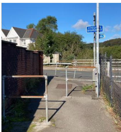
Photo 2-38 - Staggered barrier at the Heol Crymlyn end of the link (cyclist dismount/direction signage partially blocked by lamp column)
