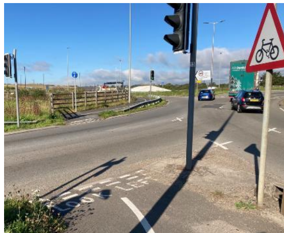
Photo 2-17 - Uncontrolled crossing across M4 J43 westbound off-slip (looking south)
