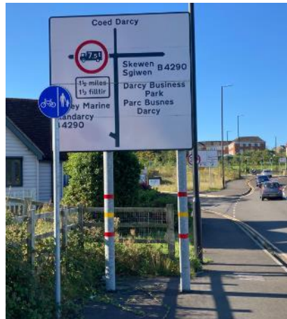
Photo 2-8 - Incorrect signage indicating wrong footway type
