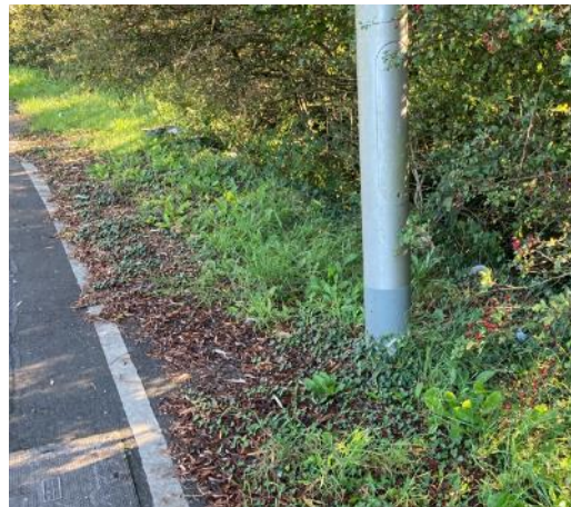
Photo 2-21 - Verge creep blocks pedestrian side of segregated provision and a lighting column is also placed in the centre of it
