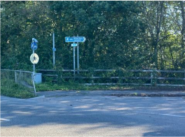
Photo 2-24 - Signage on the northern side of the M4 Junction 43 eastbound on-slip includes a segregated provision sign facing the wrong direction
