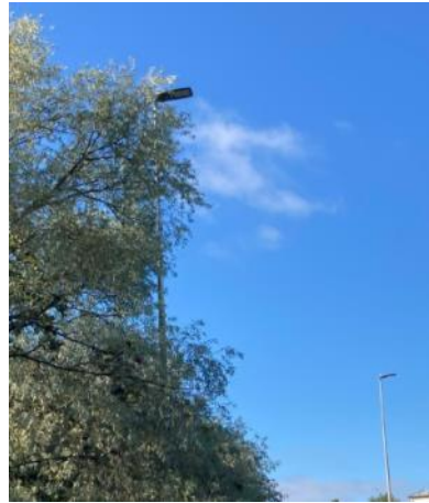
Photo 2-25 - Vegetation blocking existing lighting column above segregated provision
