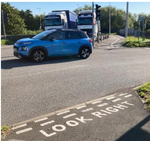
Photo 2-16 - Uncontrolled crossing across M4 J43 westbound off-slip (looking north)
