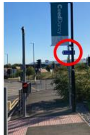
Photo 2-4 - Shared facility pinch point and partially blocked signage due to street furniture
