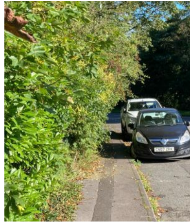
Photo 2-31 - Narrow footway (approx. 0.5m) due to vegetation, which also housed a swarm of insects
