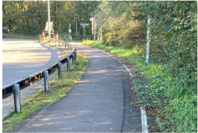
Photo 2-19 - Verge creep completely blocks pedestrian side of segregated path
