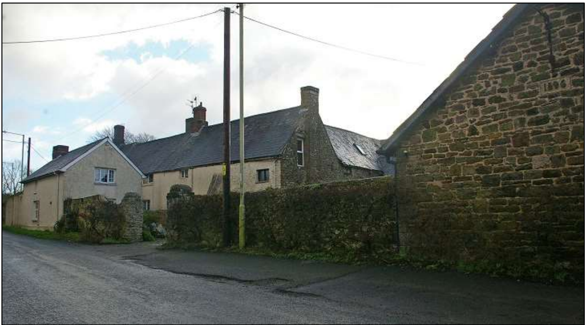
FIGURE 15: MARLAS HOUSE, WITH 19 TH CENTURY FARM BUILDINGS TO RIGHT. VIEWED FROM THE NORTH-WEST.
