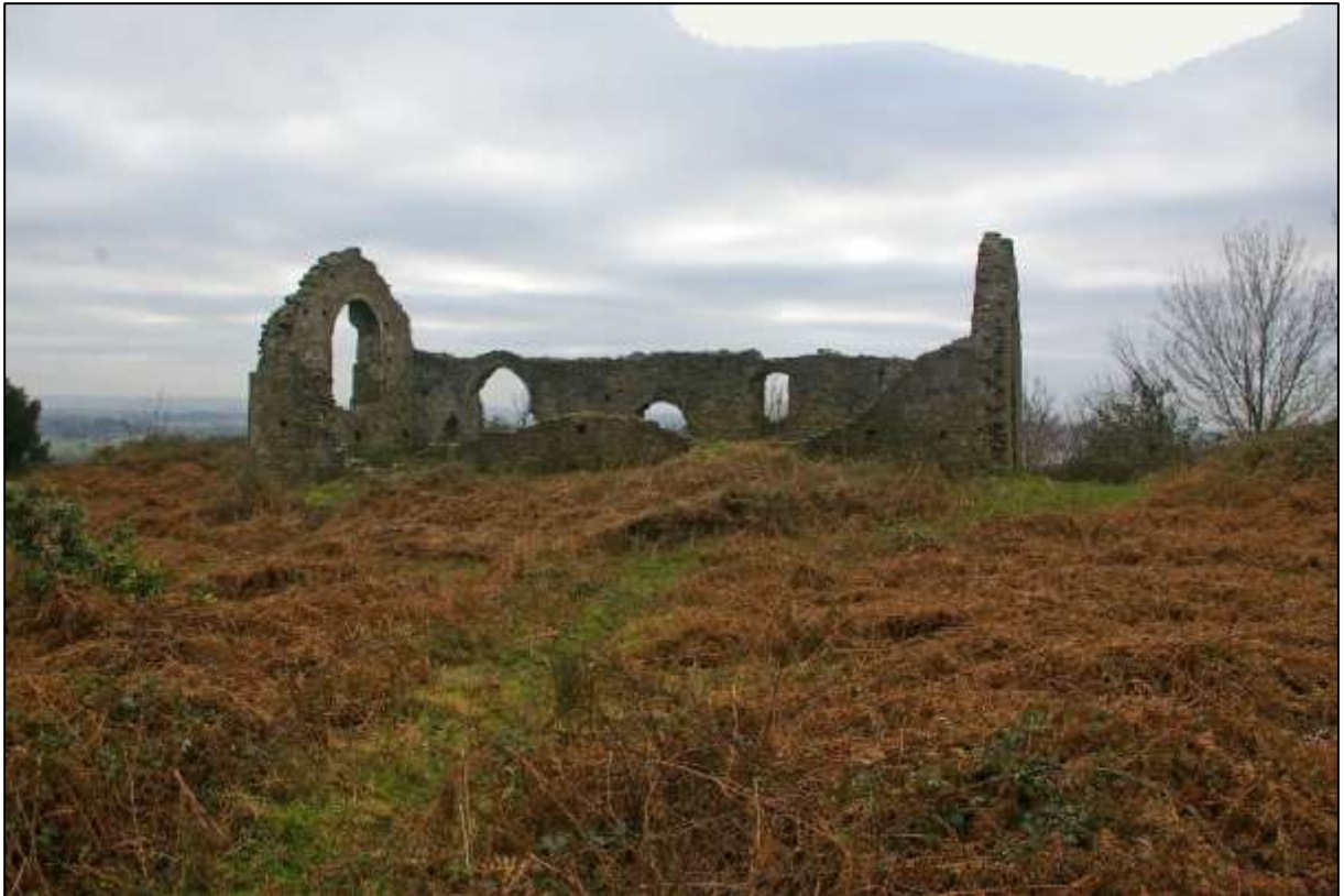
9. CAPEL MAIR, LOCATED ON AN OPEN MID-SLOPE PROMONTORY ABOVE MARGAM PARK; VIEWED FROM THE NORTH-WEST.
