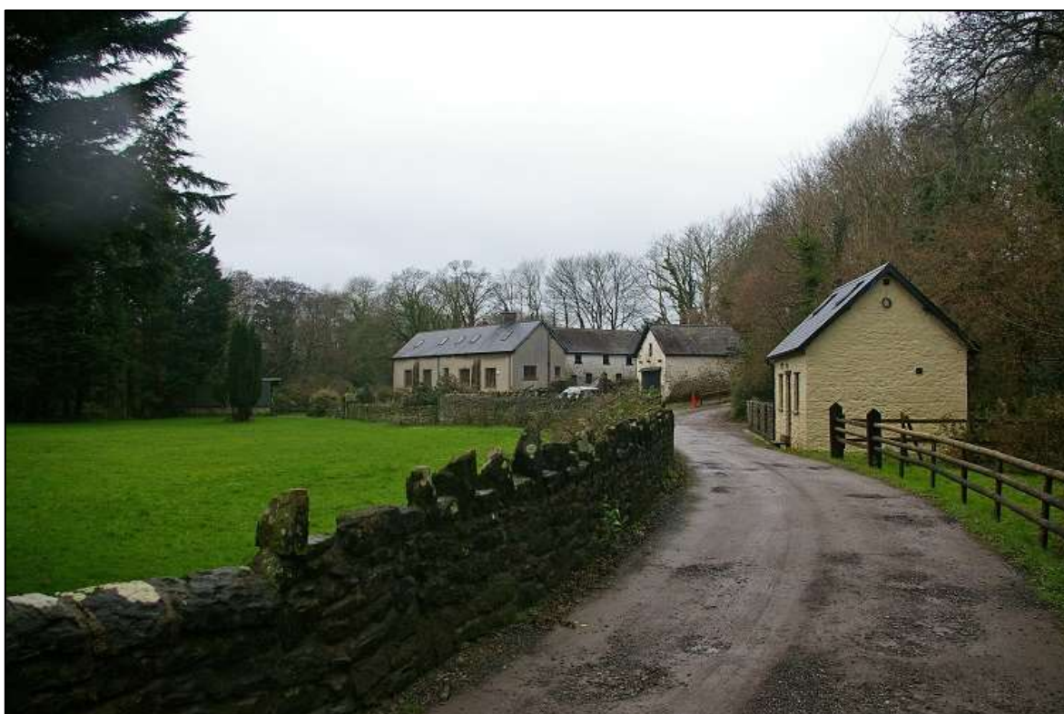
FIGURE 16: LANMIHANGEL MILL, LEAT AND DAM; VIEWED FROM THE SOUTH-EAST.
