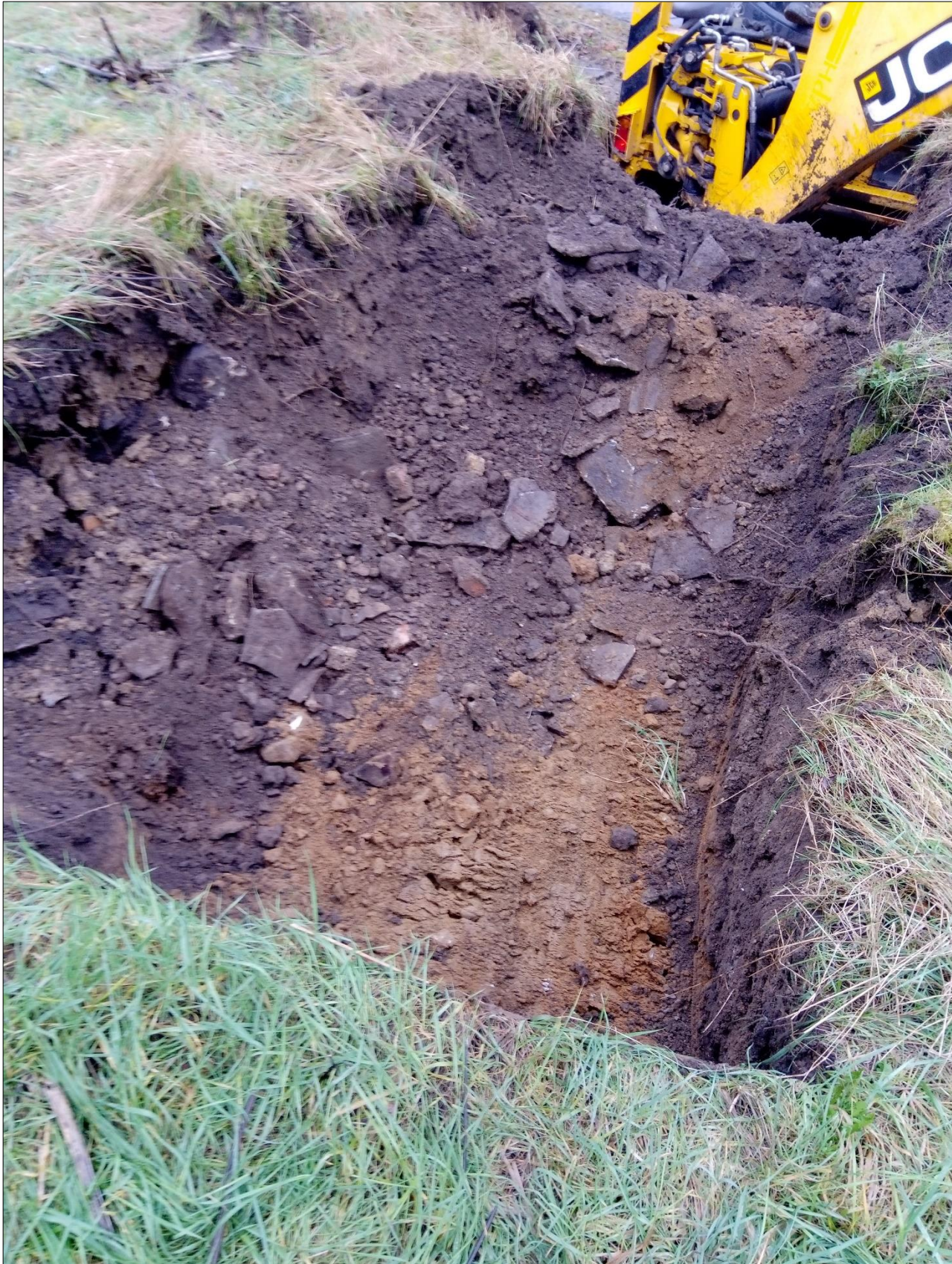
Figure 11. Excavation works, 1 m down. Feature not visible. Residual natural mottled orangish brown sandy gravelly CL:AY visible at base of pit. Boulders and cobbles present in brown topsoil/made ground above possibly from head of well.
