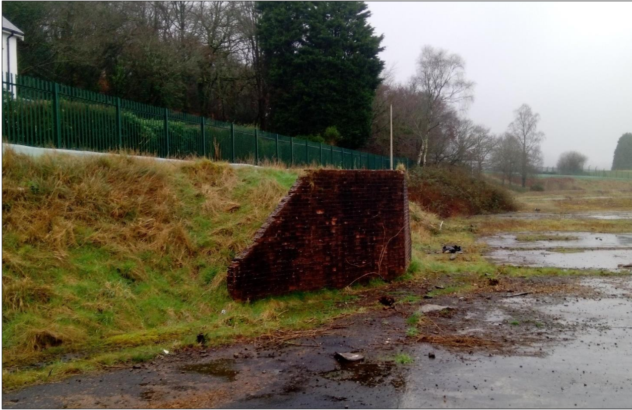
Figure 9. View of wind-retaining wall structure along the western site boundary
