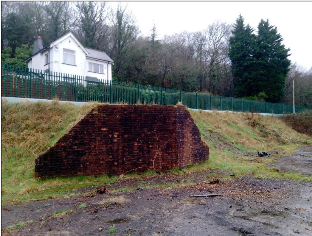
Figure 2. View looking north at estimate location of well/mine entry (behind the winged retaining wall an underneath earth embankment).
