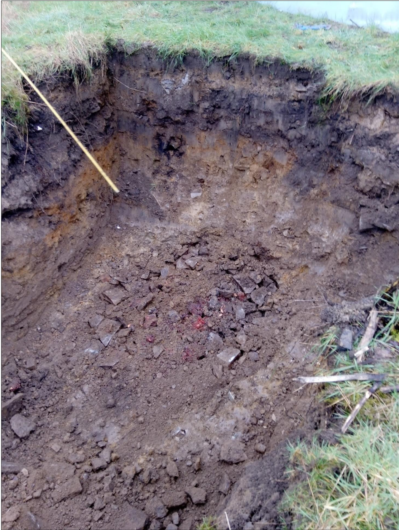
Figure 12. Photograph of excavation at 1.9 m depth, with feature perimeter blockwork observed and clinker backfill with voids present.
