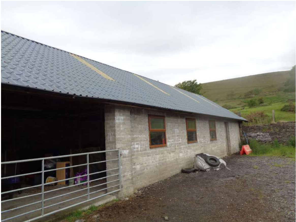
Photograph 1 – Front elevation, viewed from the south-east corner.
