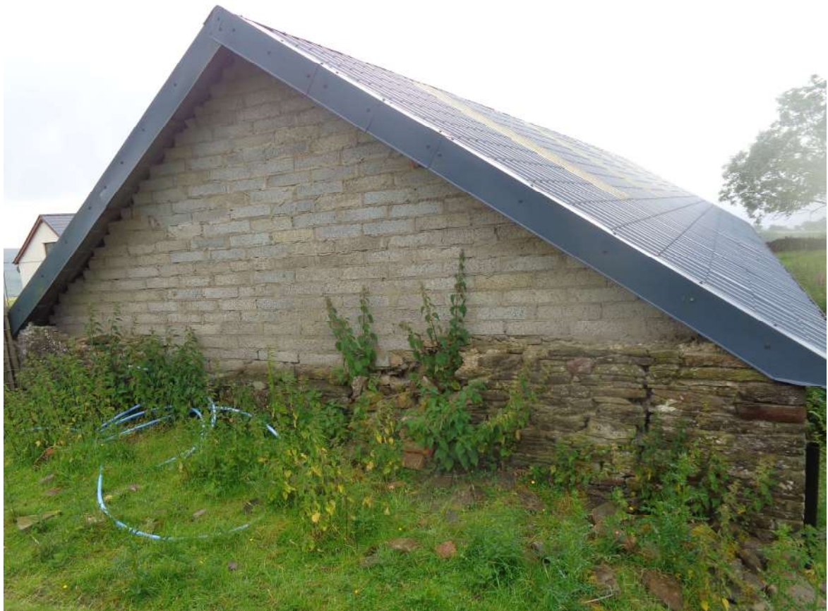
Photograph 5 – North-facing gable elevation.
