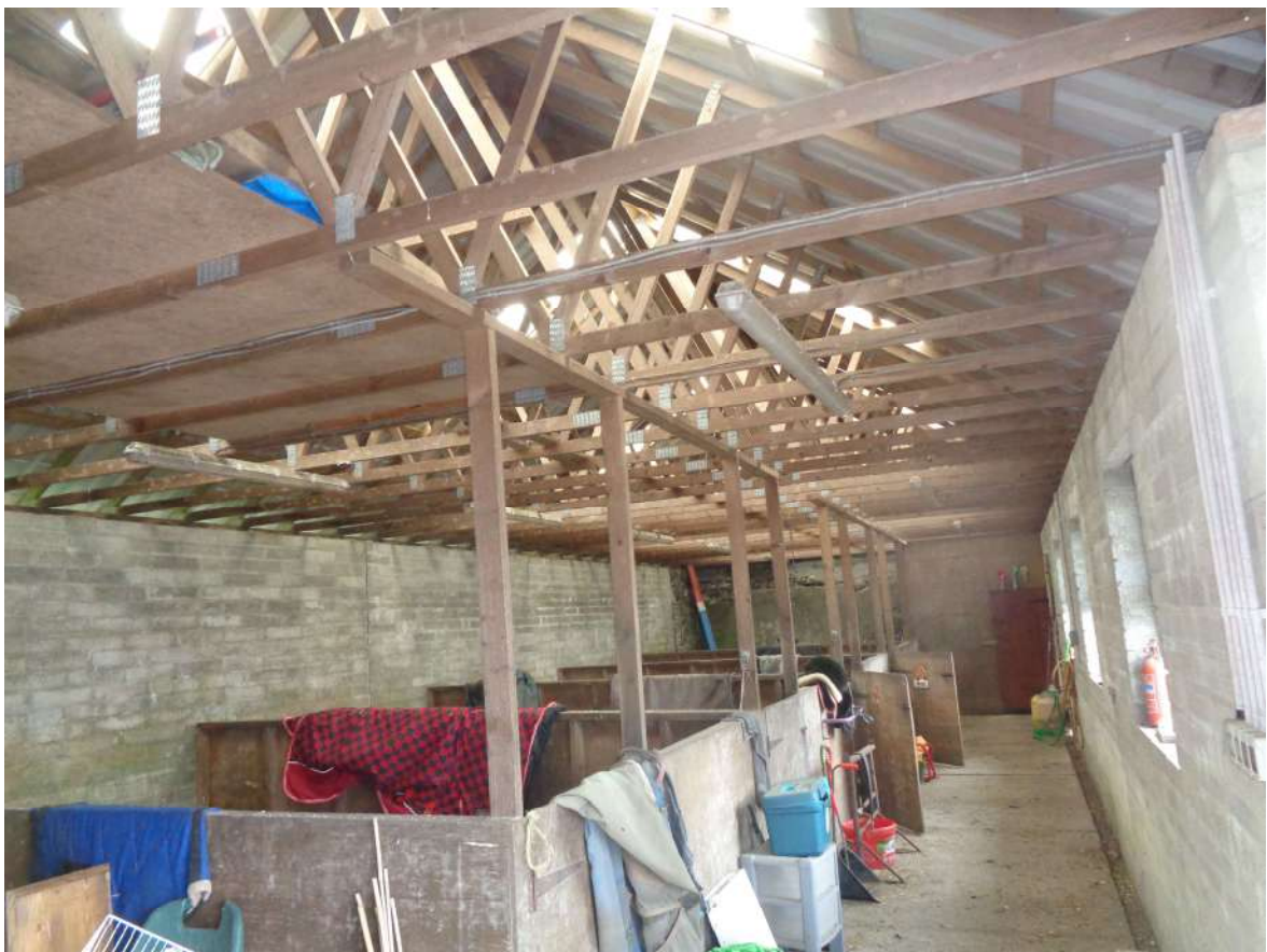
Photograph 6 – Internal view of building, facing northwards.
