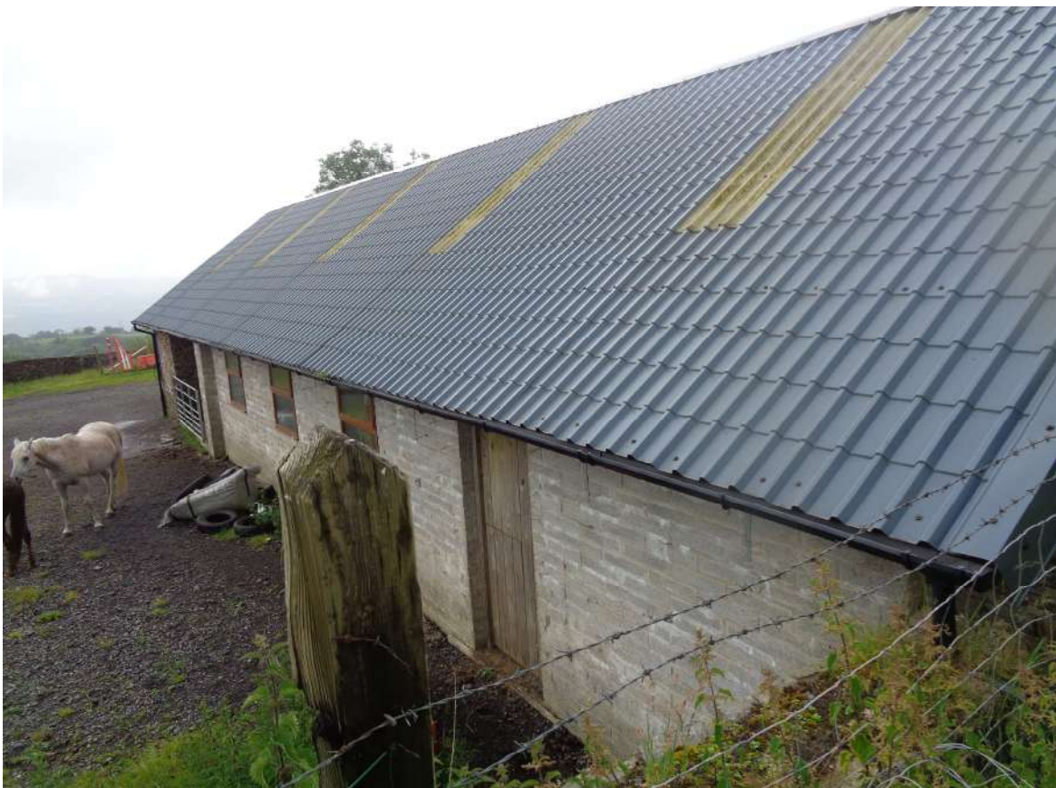
Photograph 2 – Front elevation, viewed from the north-east corner.
