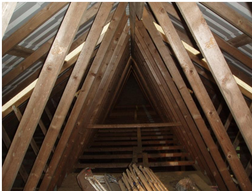
New truss roof structure
