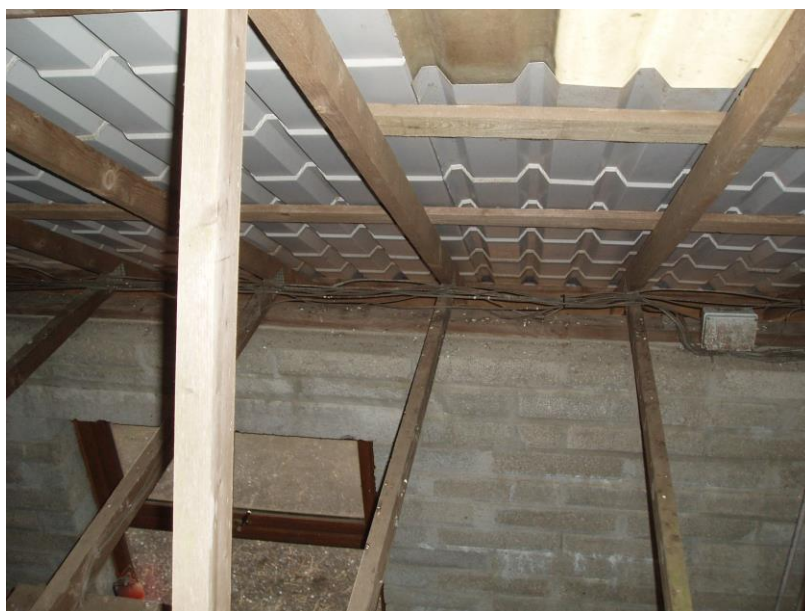
Metal profile roof showing polycarbonate light
