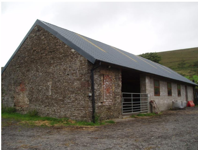
The south east gable and eastern elevation.
