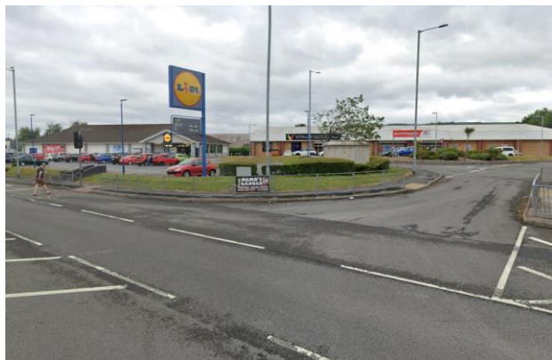
View looking towards the site (from the East)
