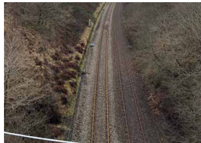
RAIL LINE BISECTING SITE
