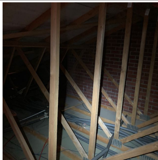
Figure 9. Loft space above single storey section to the north.
