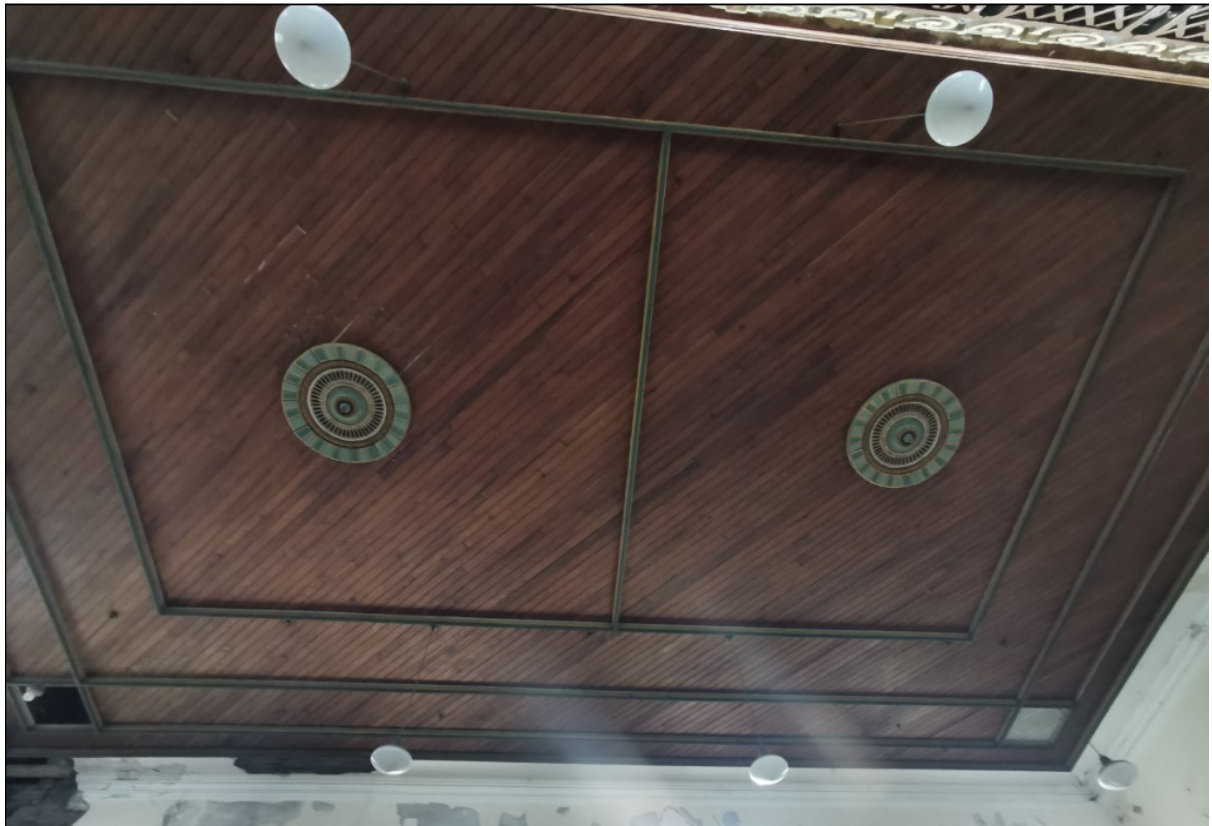
Figure 13 - Decorative, pitch pine planked ceiling, complete with two large ceiling roses
