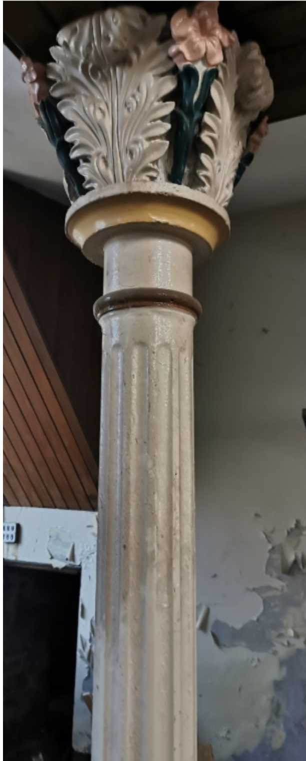
Figure 15 – One of the nine decorative, supportive cast-iron columns...
