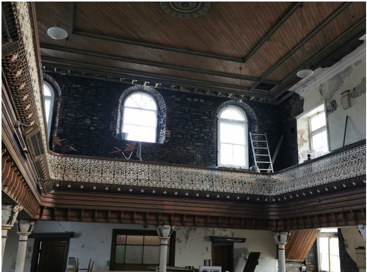
Figure 12 - Decorative, cast-iron handrails and ceiling
