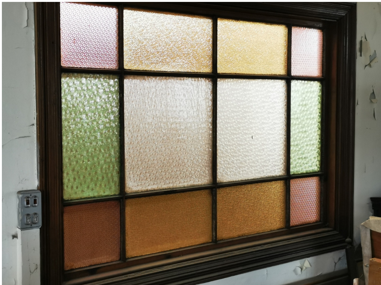
Figure 14 - Decorative, stained-glass window divider, between foyer and chapel
