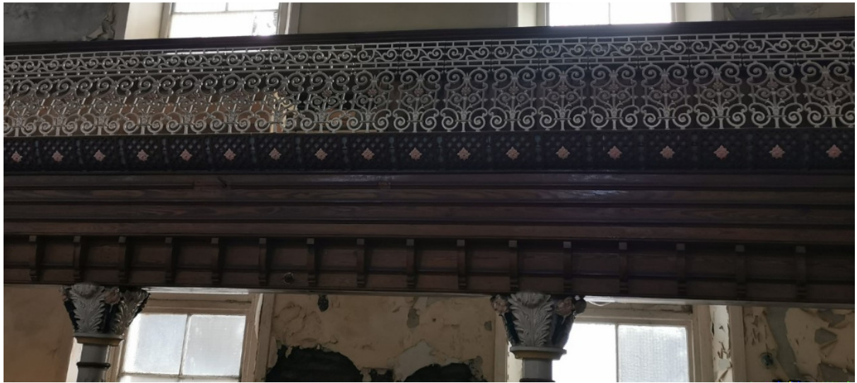
Figure 11 - Decorative, cast-iron handrails around the upper gallery of Bethel
