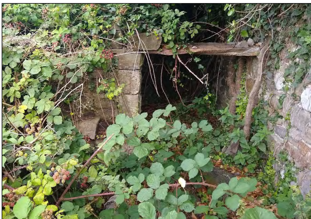
Photo 6: Image of storage structure, looking north
