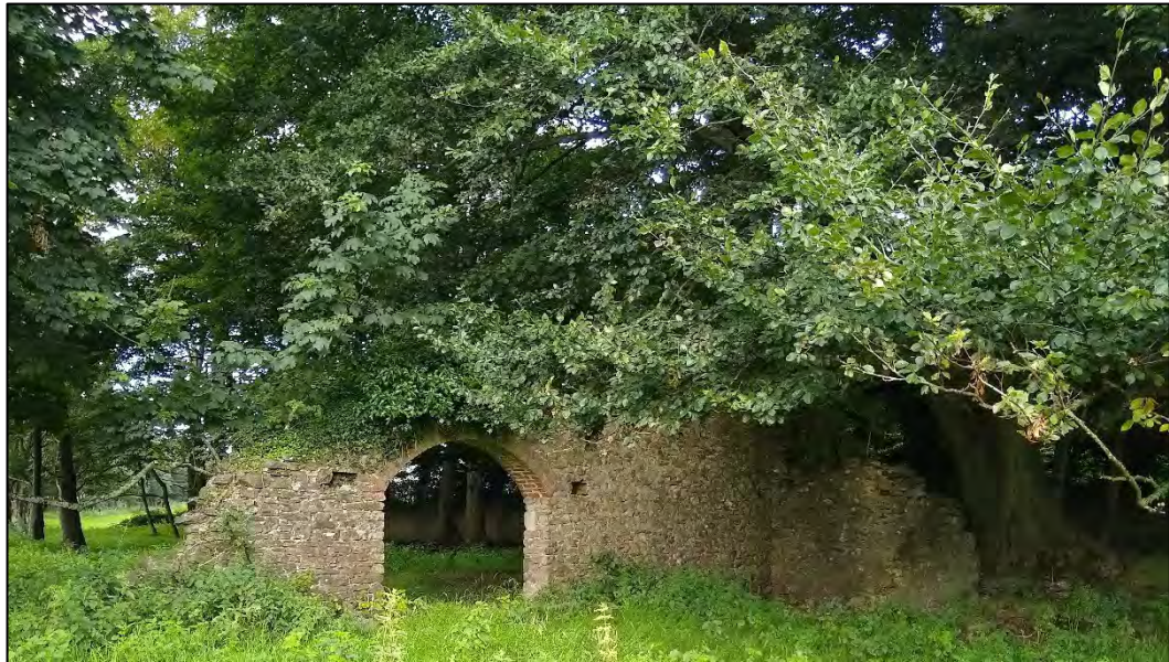
Photo 5: Image of surviving eastern wall, looking west
