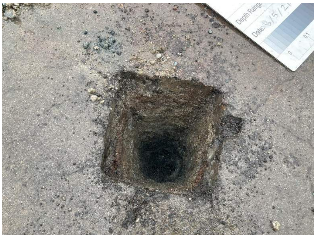
Plate 22 WS202 Inspection pit
