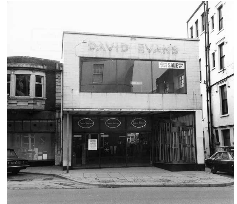
The Picturedrome then Capitol, High Street, Port Talbot (after conversion to a David Evans store) (source: cinematreasures.org)
