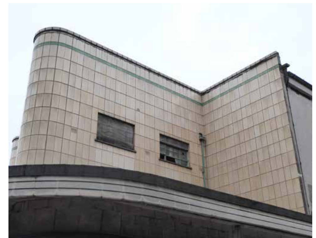
A recent photo of the Plaza frontage shows that, despite its dereliction, it retains the iconic Art Deco forms, lines & features
