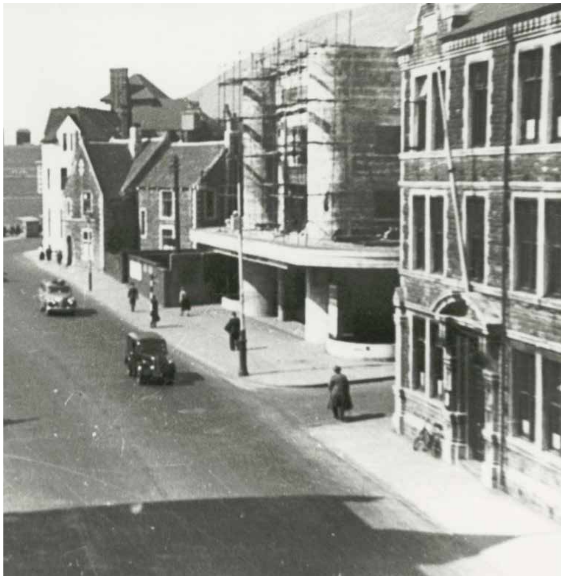
Plaza exterior approx 1950 - building receiving sign, tiles and windows 10 years after opening (source: Port Talbot Historical Society)
