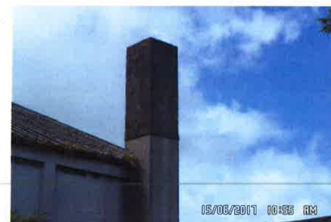
Rear Chimney cracked and leaning (June 2017) Top portion of chimney removed (July 2017)
