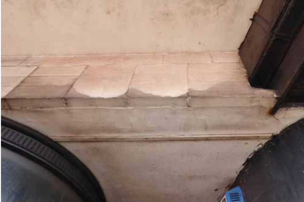
M Stone Cladding above openings
