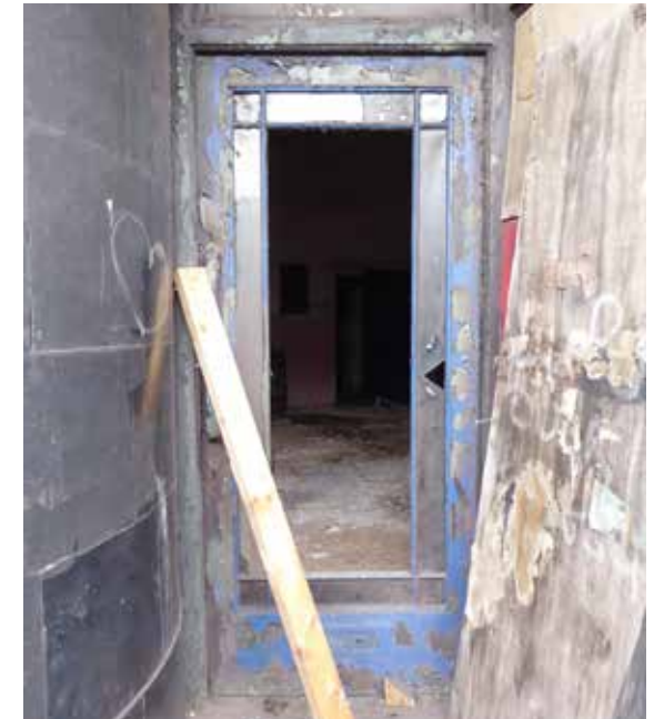
H Timber-framed Shop Doors to be Retained & Restored
