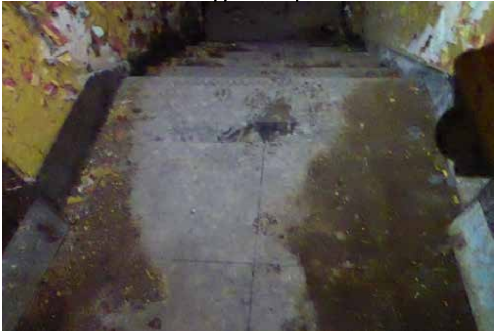
V Existing Steps to be Repaired
