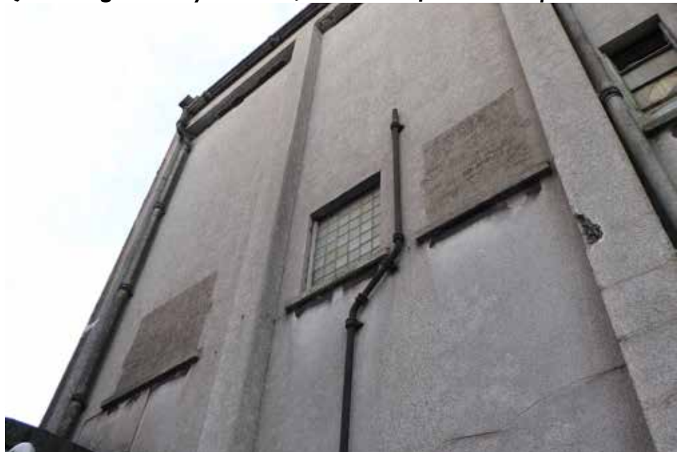
R Existing Masonry Infills to be Replaced
