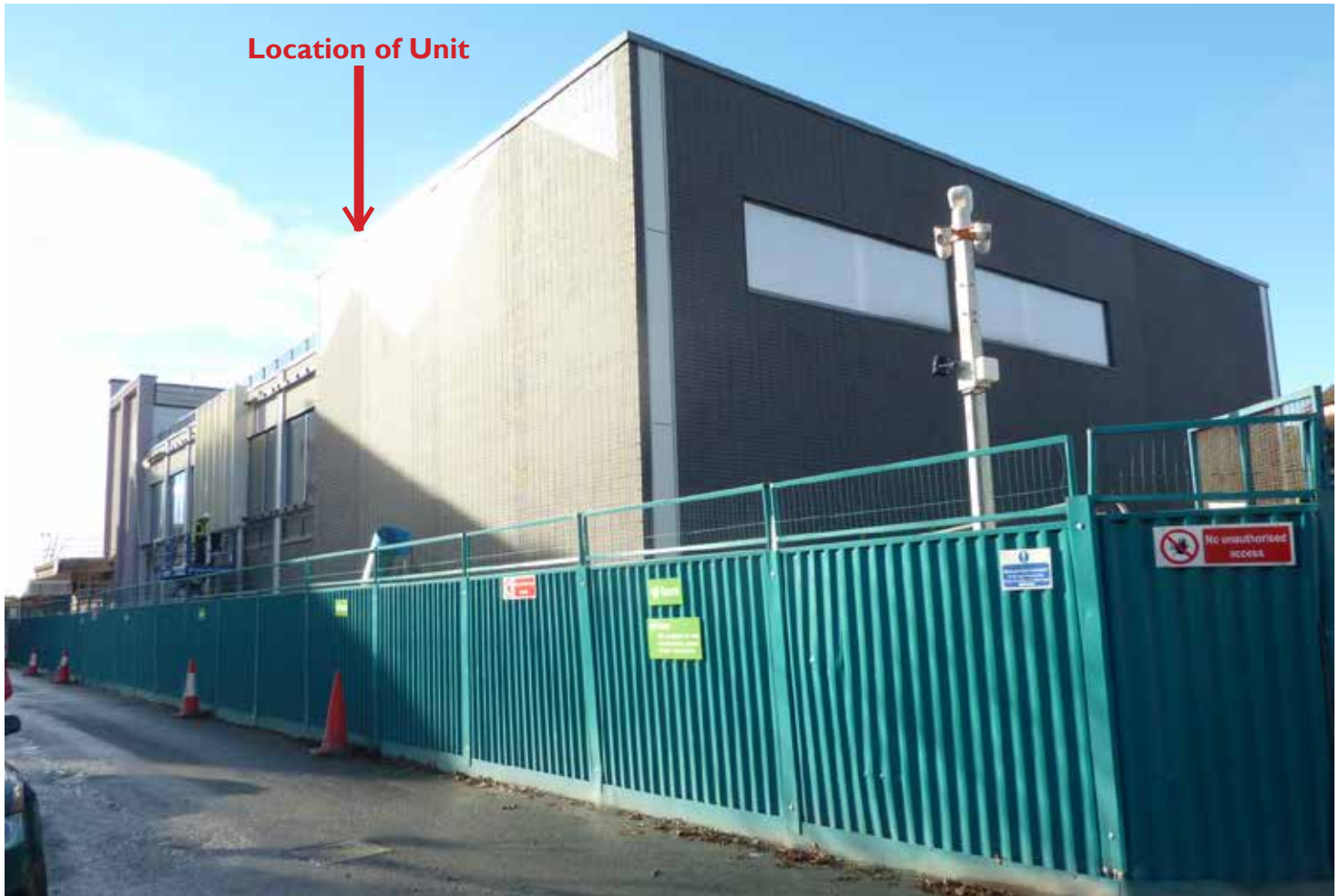
View from Eagle Street to North East of building
