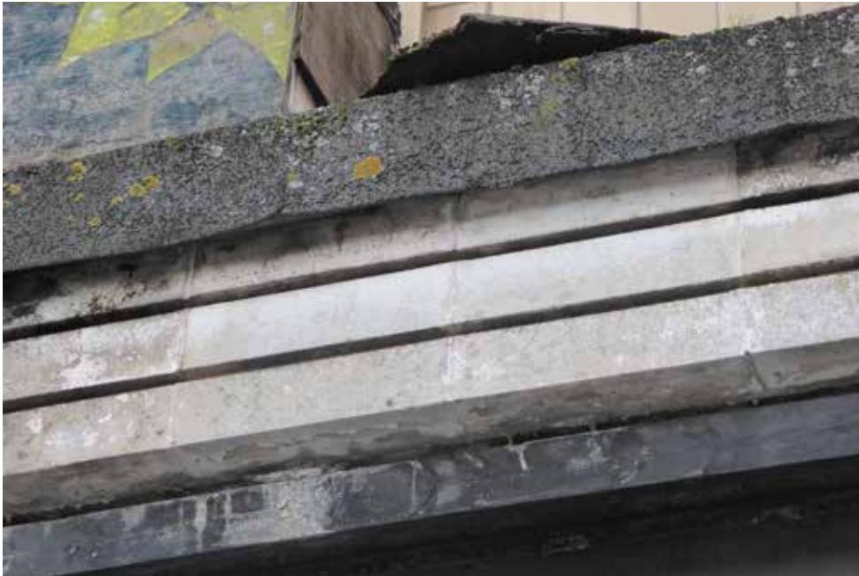
T Reconstituted Stone Profiled Fascia to Canopy with felt dressed
