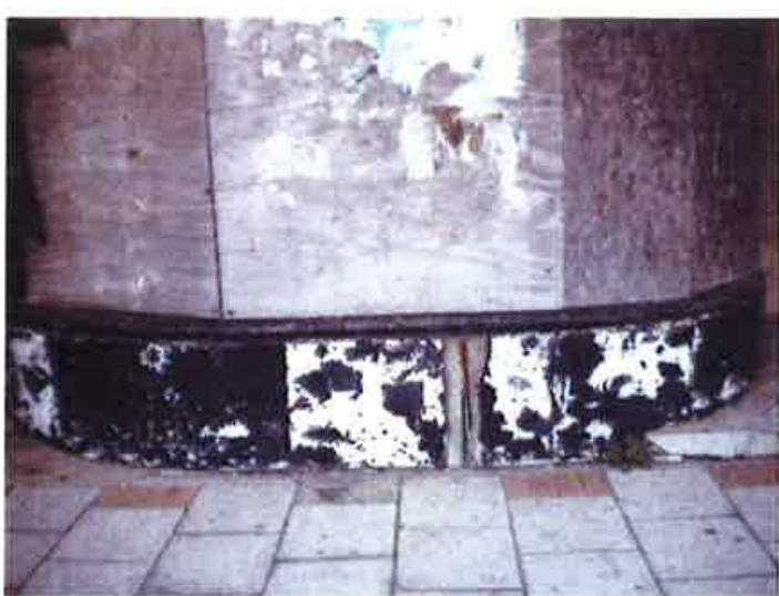
Cladding panels below window 2012
