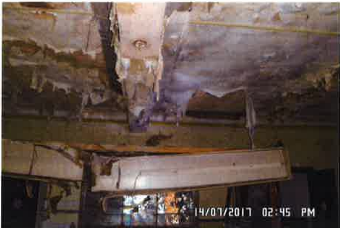
Foyer area ceiling, July 2017
