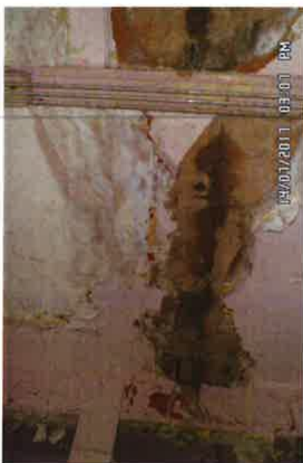
July 2017 indicates clear evidence of water penetration through hairline cracks
