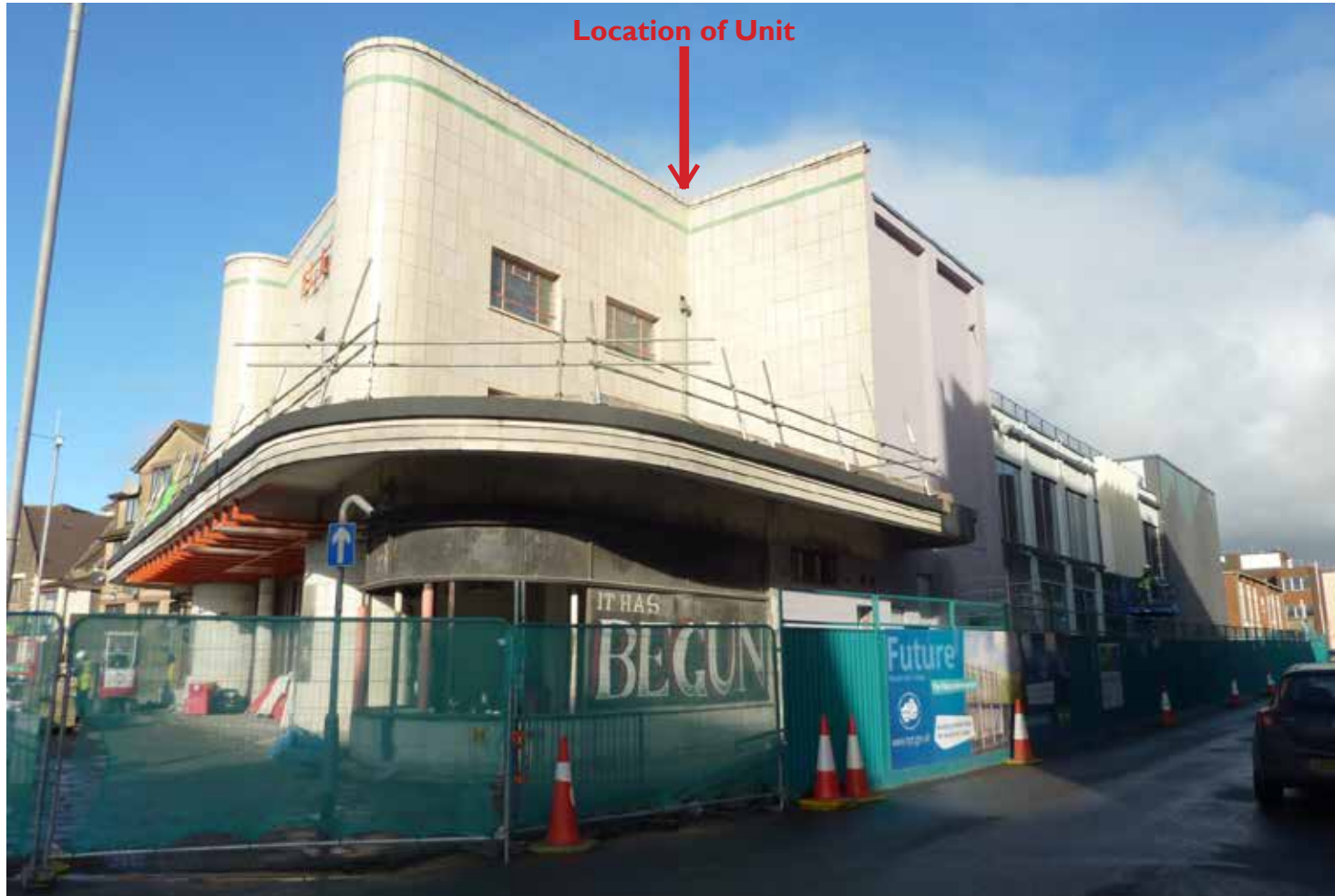
View from Talbot Road / Eagle Street junction to South of building
