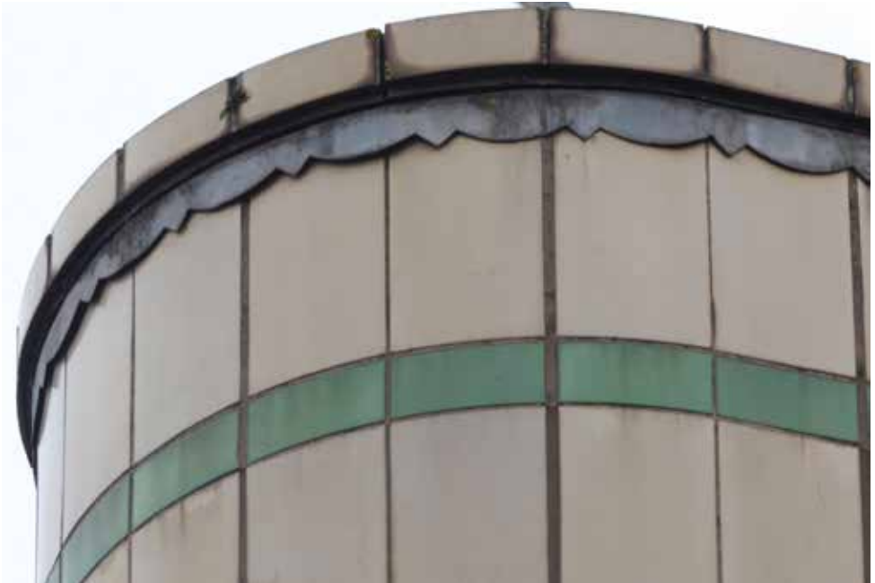
W Scalloped Lead Flashing at head of faience tiling
