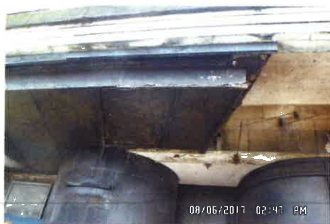
Loose/corroded metal soffit panels (June 2017) Pavement hoarded off below (July 2017)
