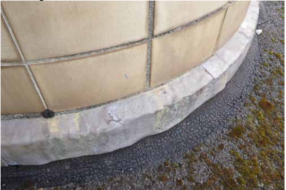
Y Lead Flashing at base of faience tiling
