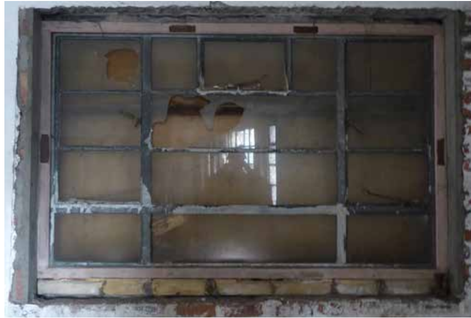
C Crittall Window to be Retained & Restored - Window S2
