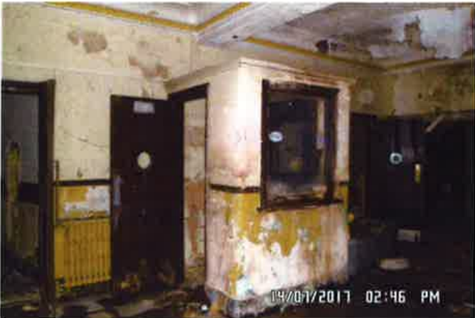
Foyer area ticket booth, July 2017
