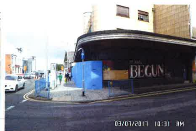
Loose/corroded metal soffit panels (June 2017) Pavement hoarded off below (July 2017)
