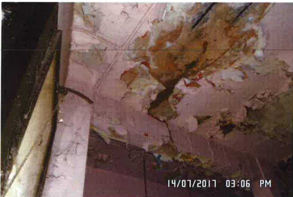
July 2017 indicates clear evidence of water penetration through hairline cracks
