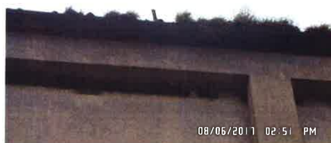
Overgrowth in high level gutters (June 2017) Overgrowth removed via MEWP (July 2017)
