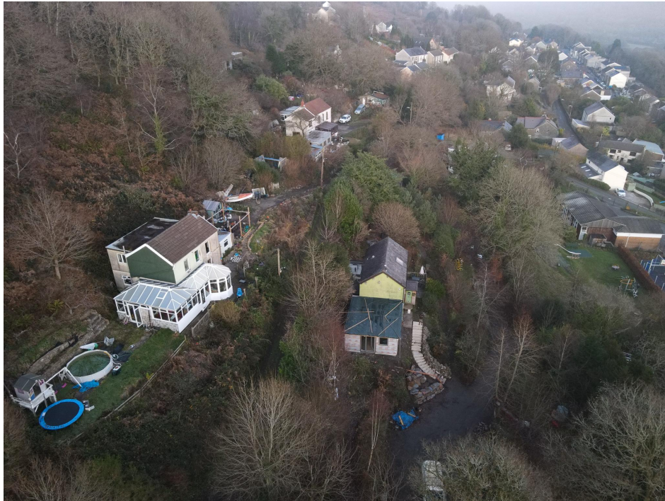
Existing dwelling with part complete single storey extension.
