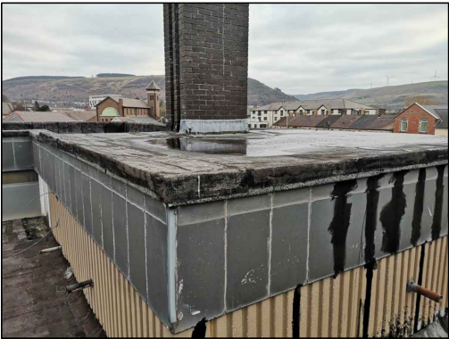
FLAT ROOF PHOTO 3
