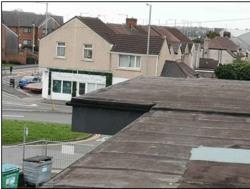
FLAT ROOF PHOTO 2
