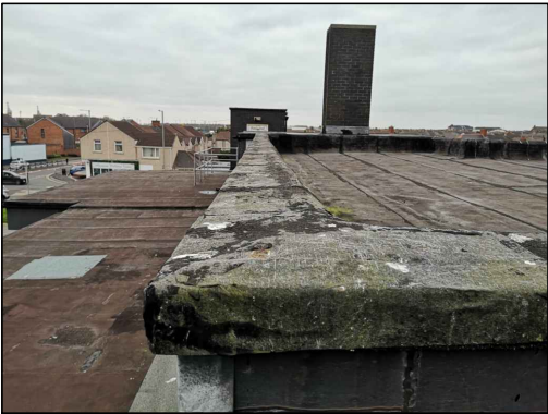
PARAPET ROOF PHOTO 1
