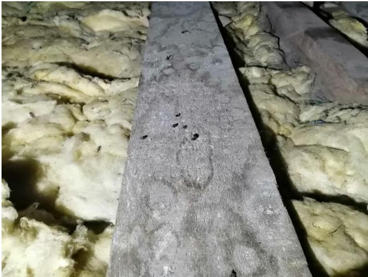
Photo 15 – Indications of Vermin (Main Roof Profile)
