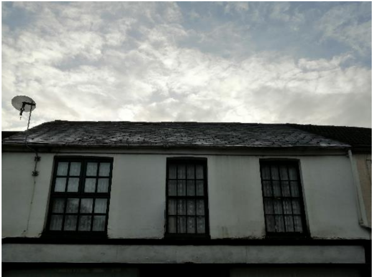
Photo 1 – Front Roof Profile
