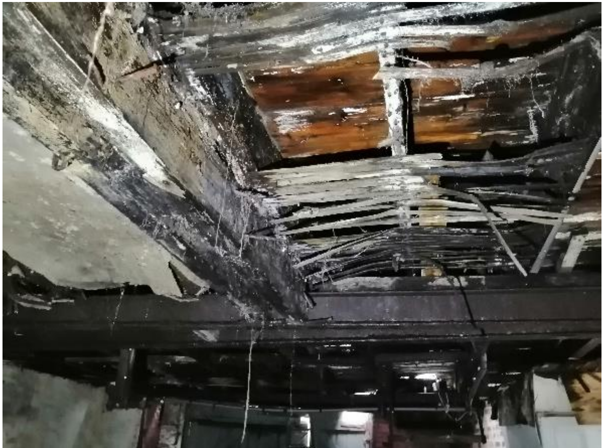
Photo 77 – Timber Structure Floor
