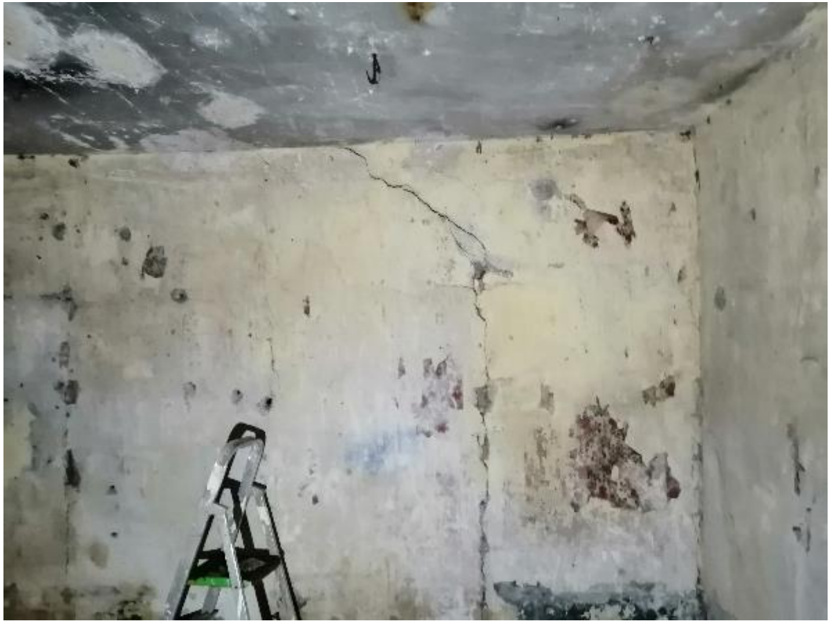
Photo 60 – Crack to Internal Wall (Basement Room 2)
