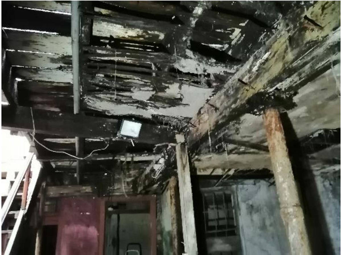
Photo 76 – Timber Structure Floor
