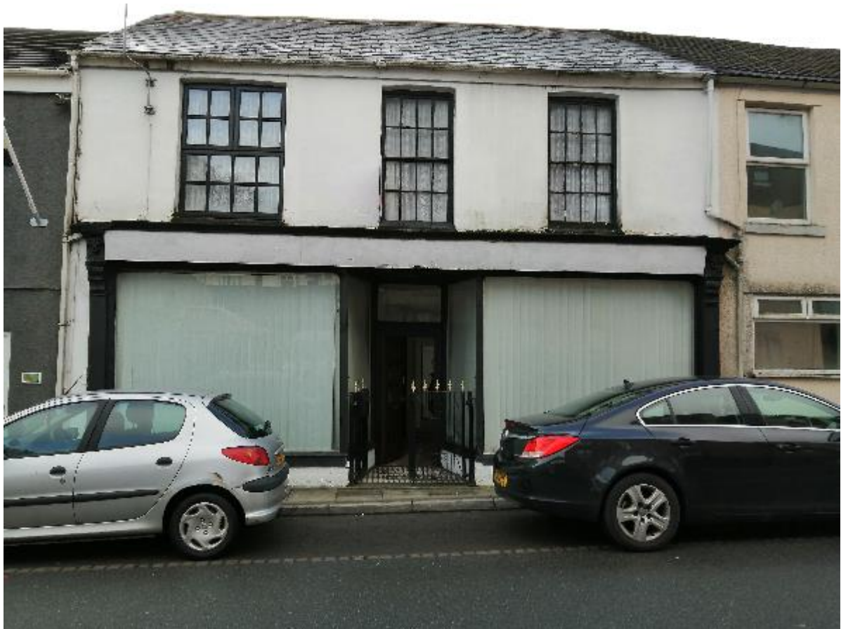
Photo 5 – Front Wall Elevation
