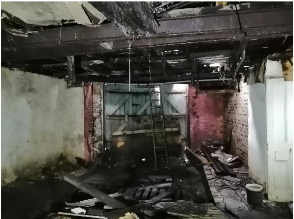
Photo 73 – Timber Structure Basement
