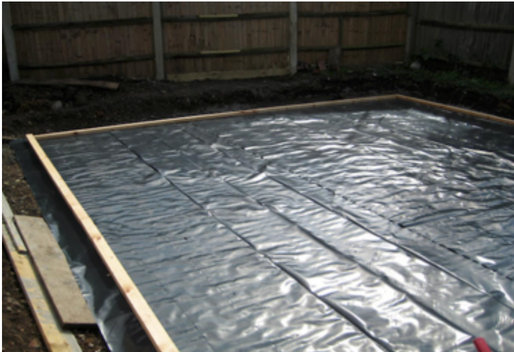
Example of a Damp Proof Membrane being installed before placement of concrete slab
