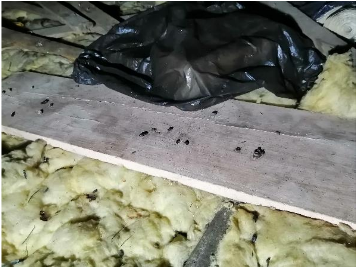
Photo 14 – Indications of Vermin (Main Roof Profile)
