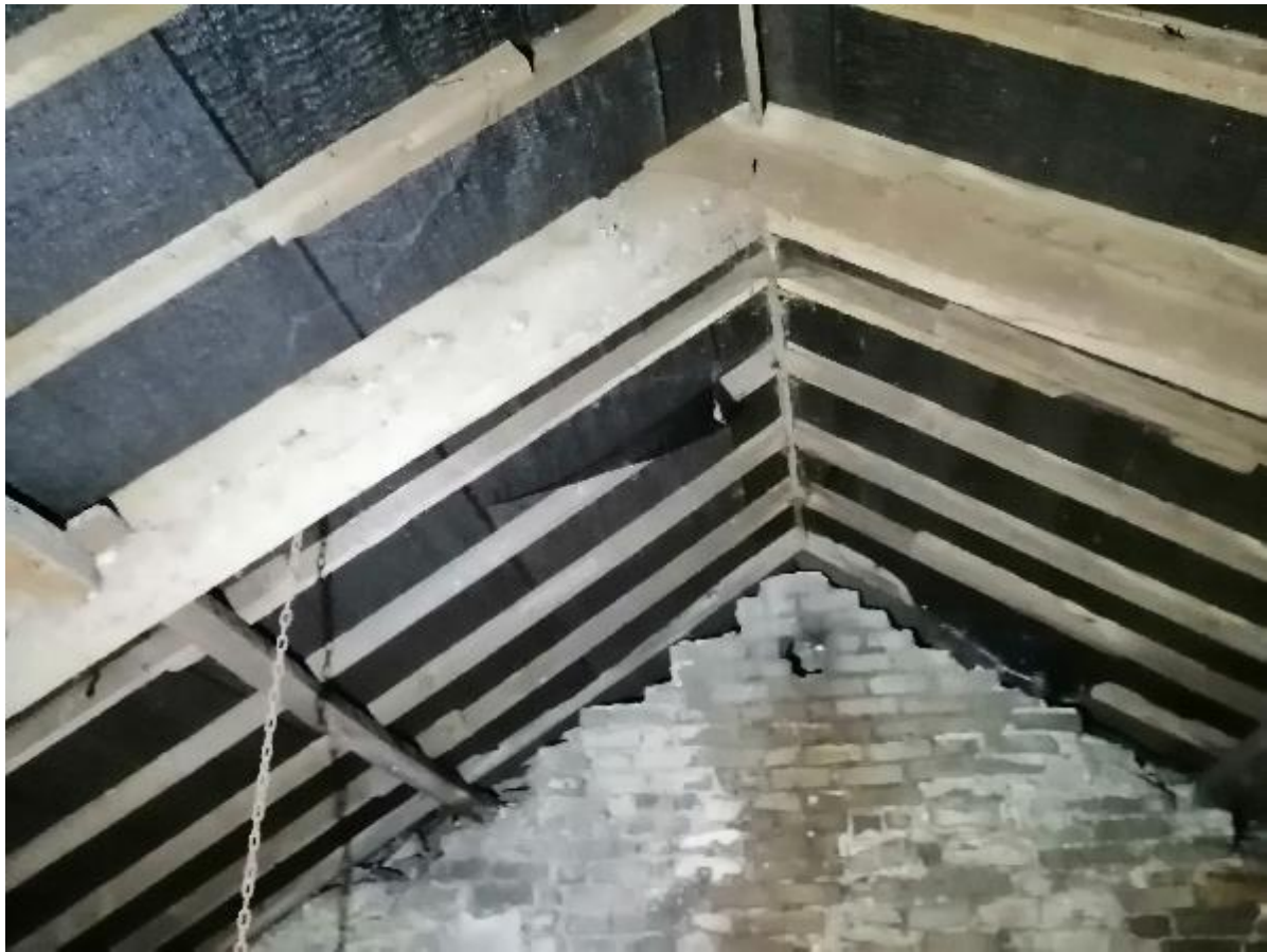
Photo 13 – Timber Roof Frameworks
