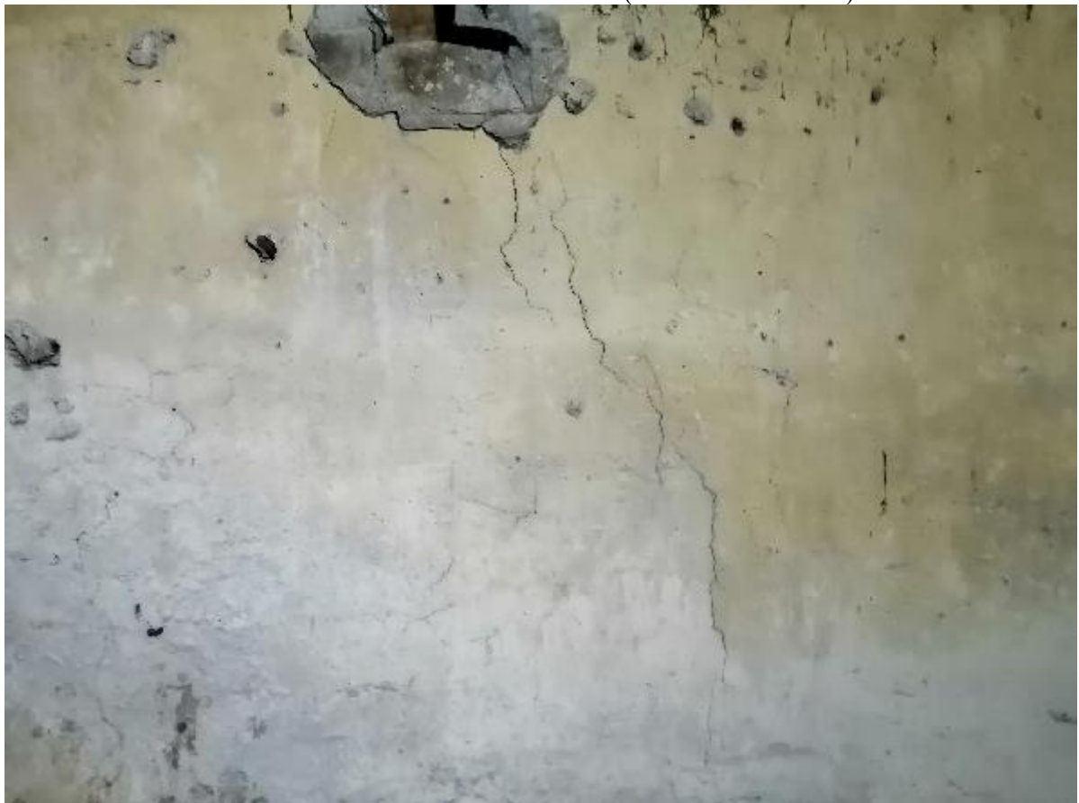
Photo 60 – Crack to Internal Wall (Basement Room 2)
