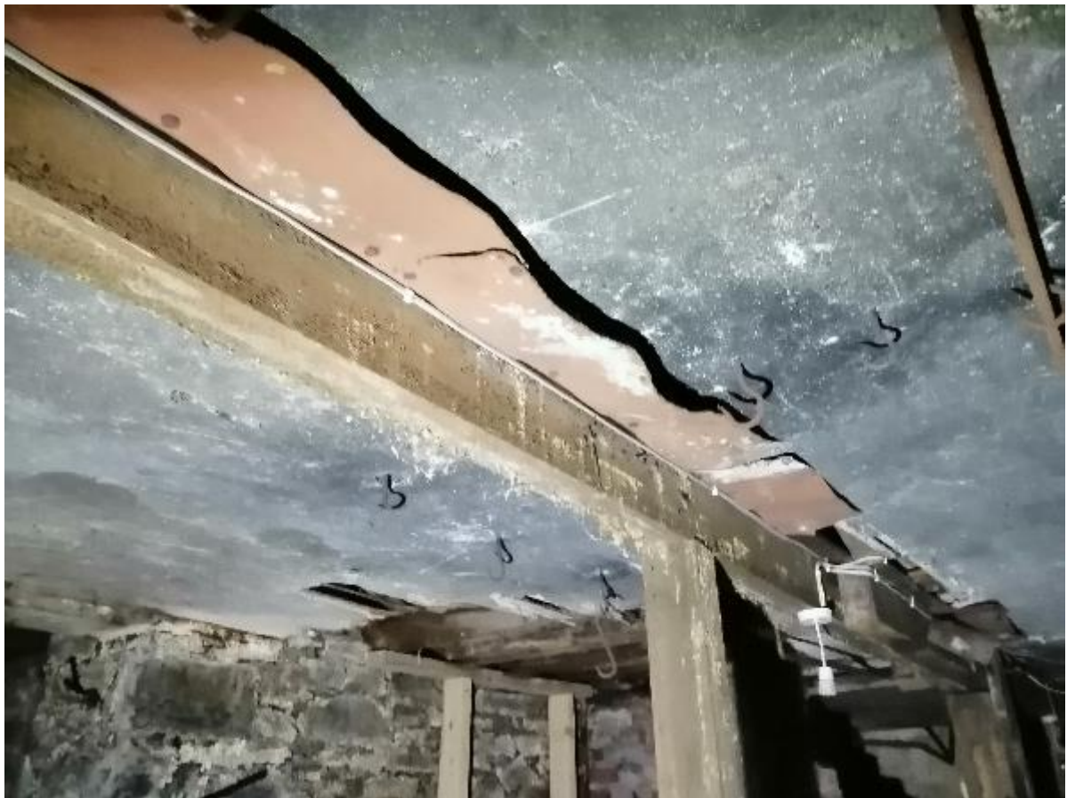
Photo 78 – Timber Column and Beam (Basement Room 4)
