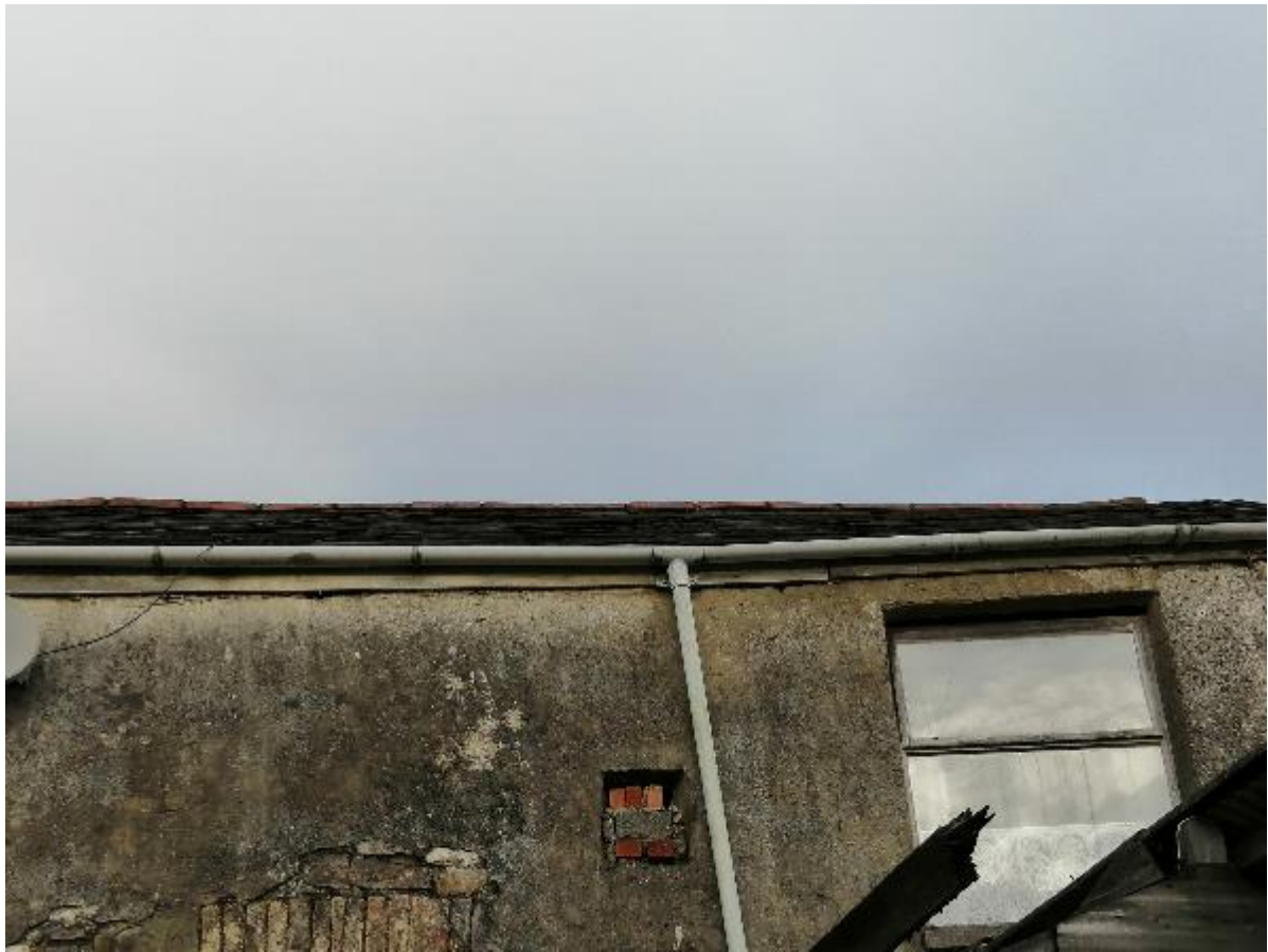
Photo 2 – Rear Roof Profile
