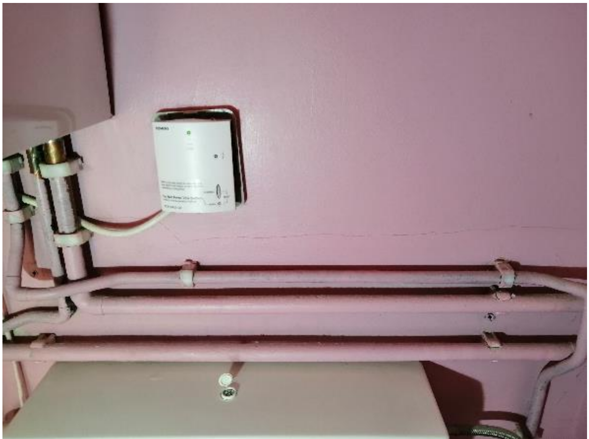
Photo 29 – Wall Plaster Crack (Bathroom)
