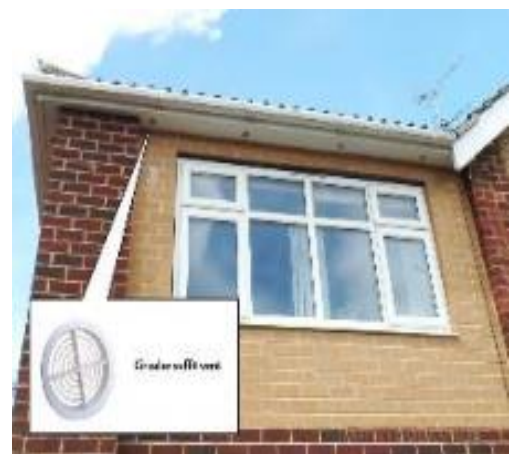
Figure 4 : Ventilation Soffit Boards
