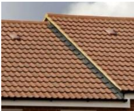
Figure 3 : Ventilation Roof Tiles
