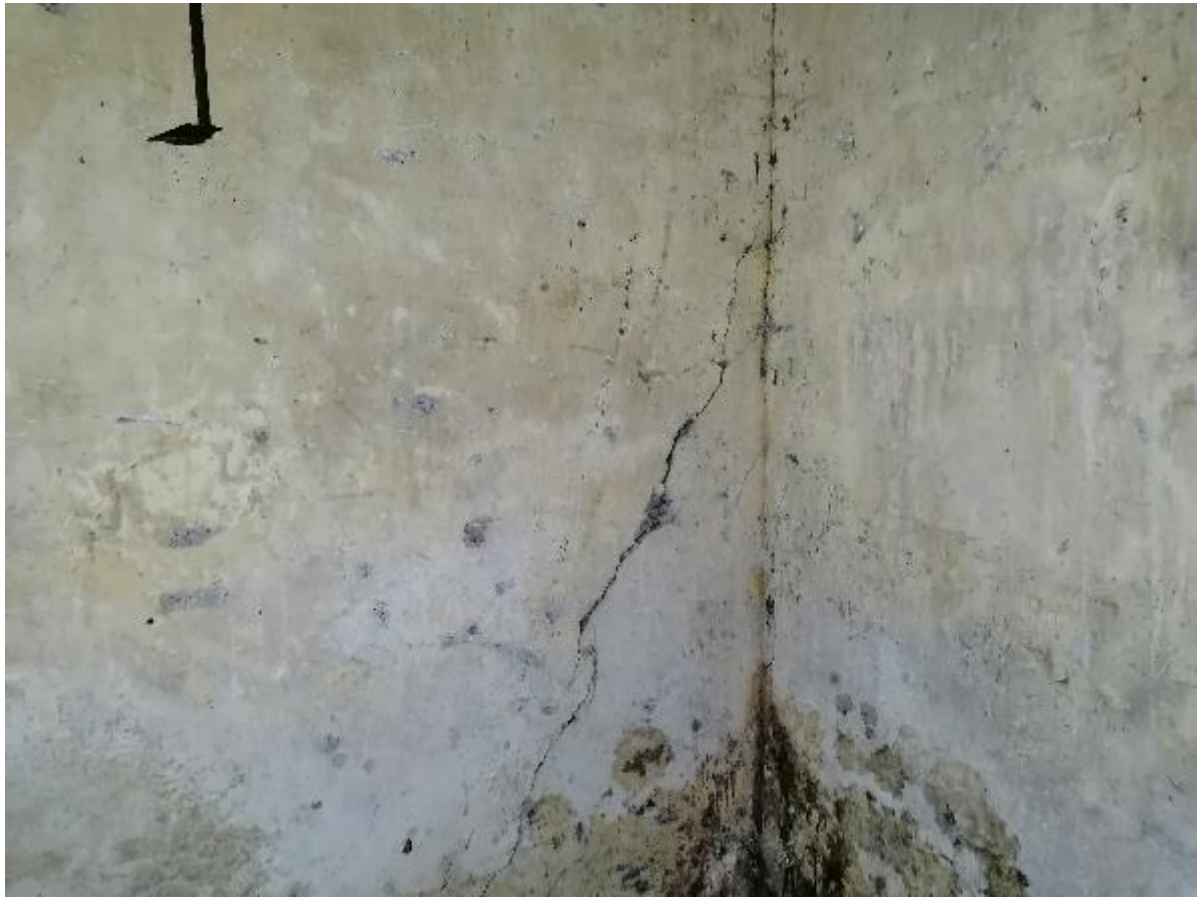
Photo 62 – Crack to External Wall (Basement Room 3)
