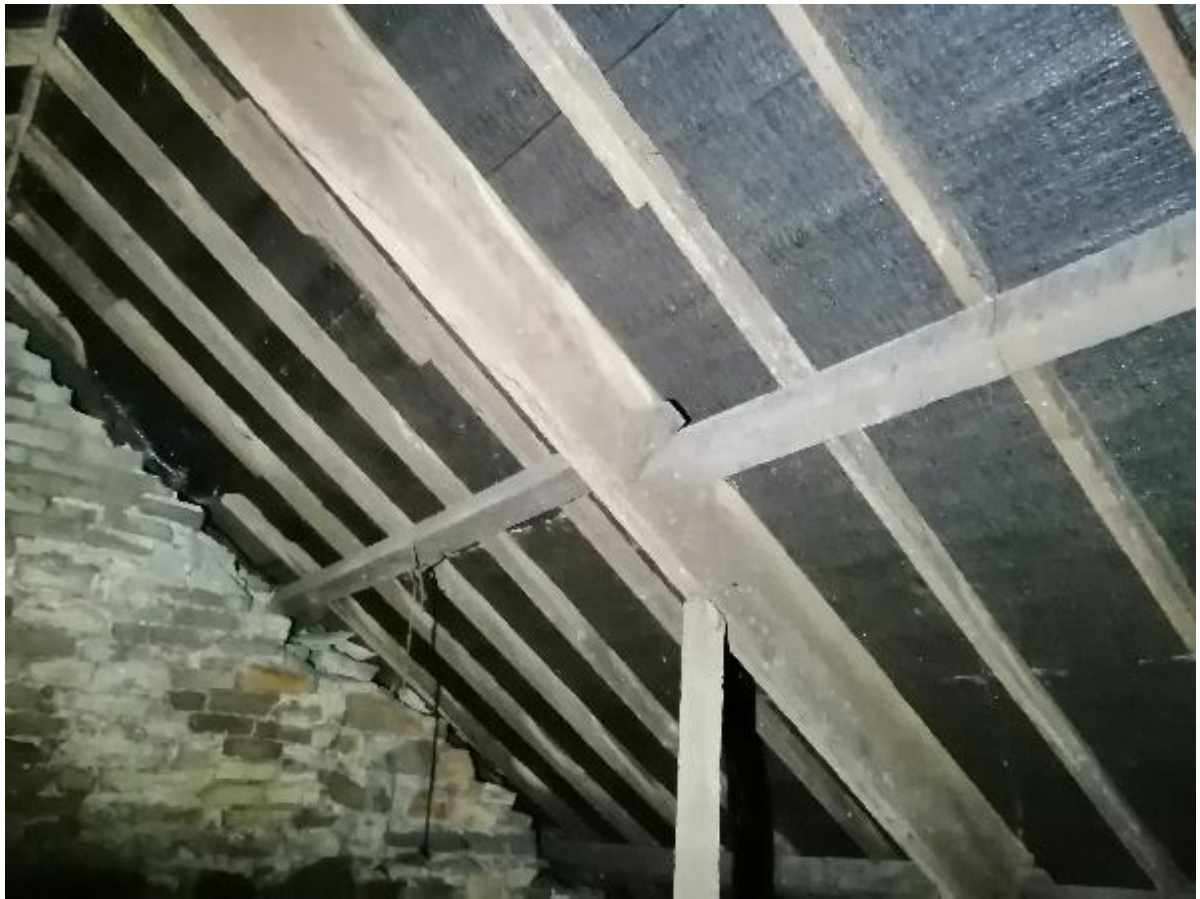
Photo 11 – Timber Roof Frameworks
