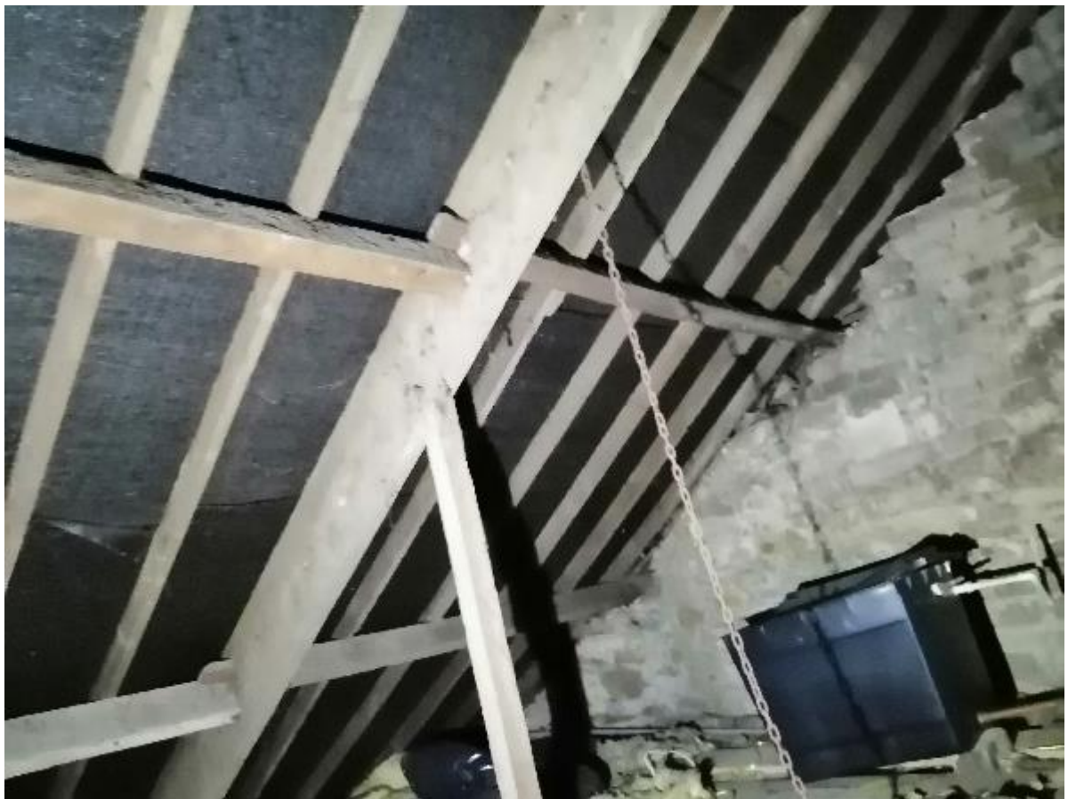
Photo 12 – Timber Roof Frameworks
