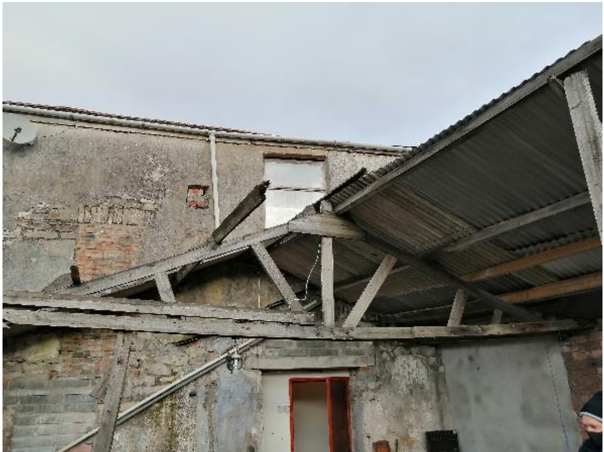
Photo 72 – Timber Structure Roof
