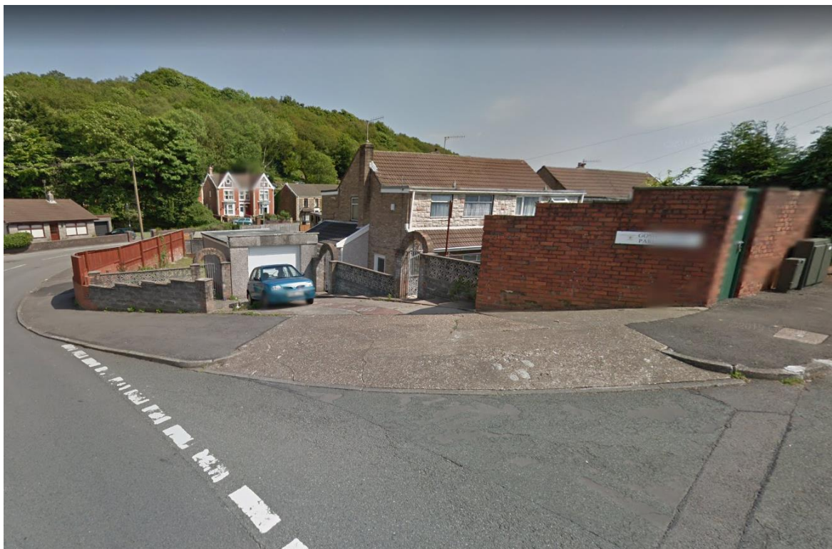
Photograph 3 – View towards the east from Drumau Road prior to demolition of the previous garage and boundary treatment
