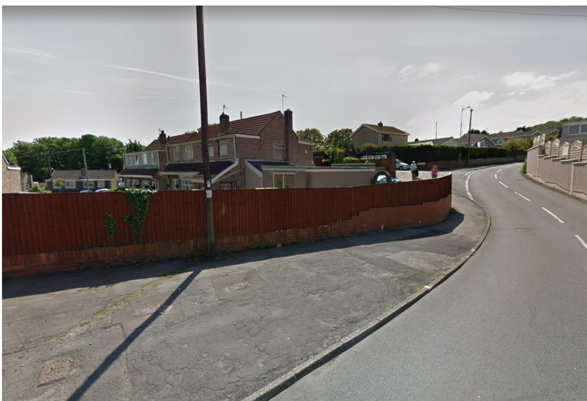
Photograph 4 – View towards the south west from Drumau Road prior to demolition of the previous garage and boundary treatment
