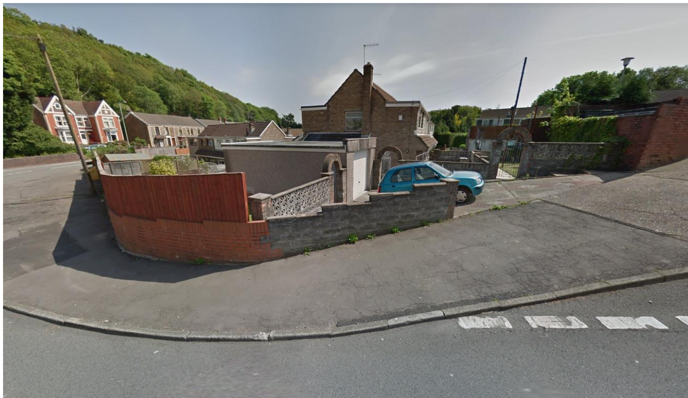
Photograph 5 – View towards the south from Drumau Road prior to demolition of the previous garage and boundary treatment
