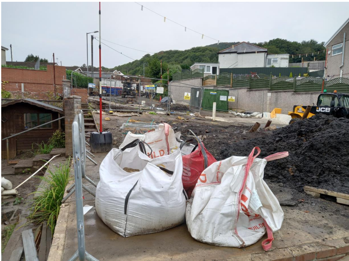
Photograph 2 – Further present view towards the west from Drumau Road
