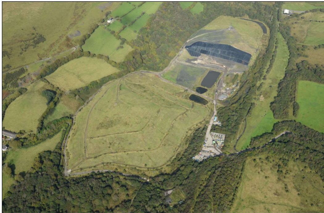
Figure 2.1: Aerial Image of Tip 890 looking north
