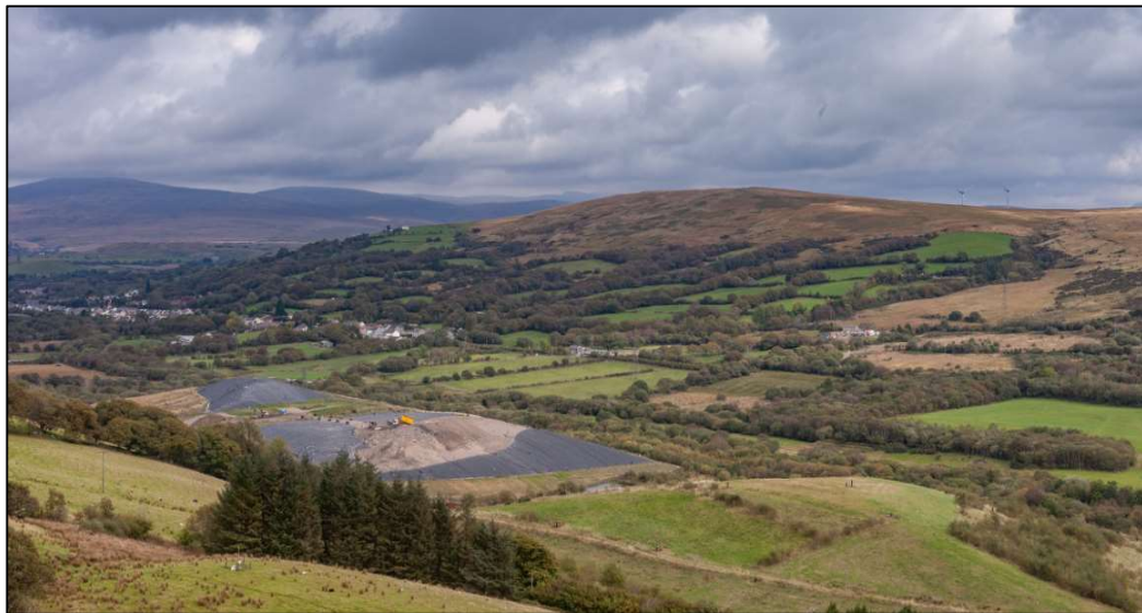
Figure 2.2: View of Tip 890 looking north-east
