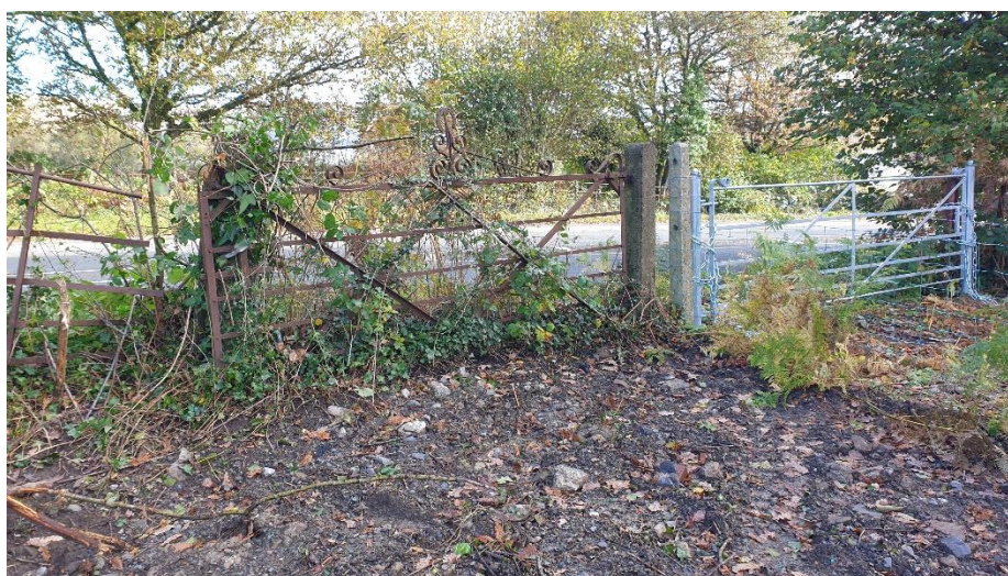
Photograph 22: Existing gated access to the south-east of the wider site
