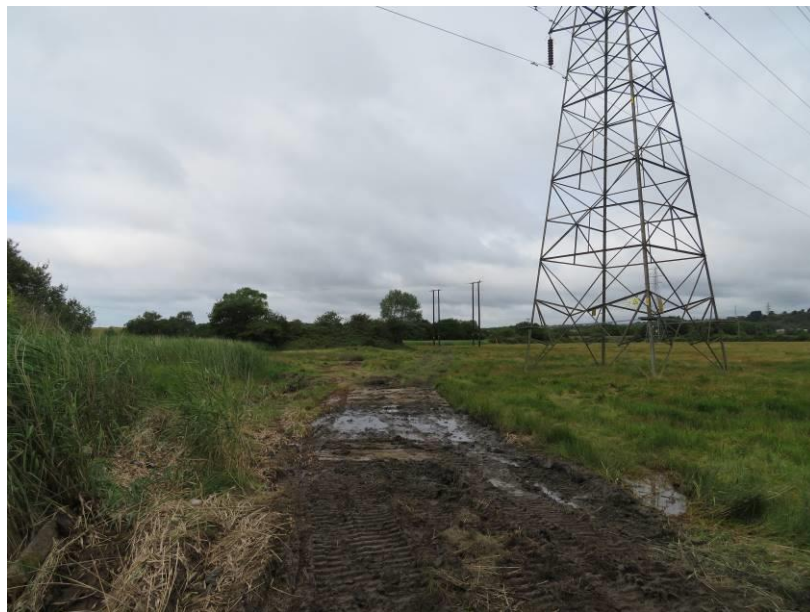
Figure 3: showing the start of the tracked area which will be used (and is) to gain access to repair the pylons.
