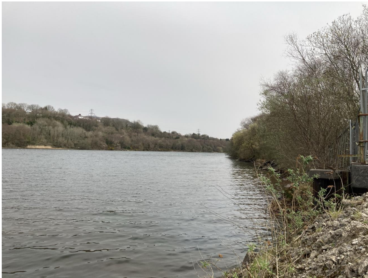
9 – North Site Reservoir facing E
