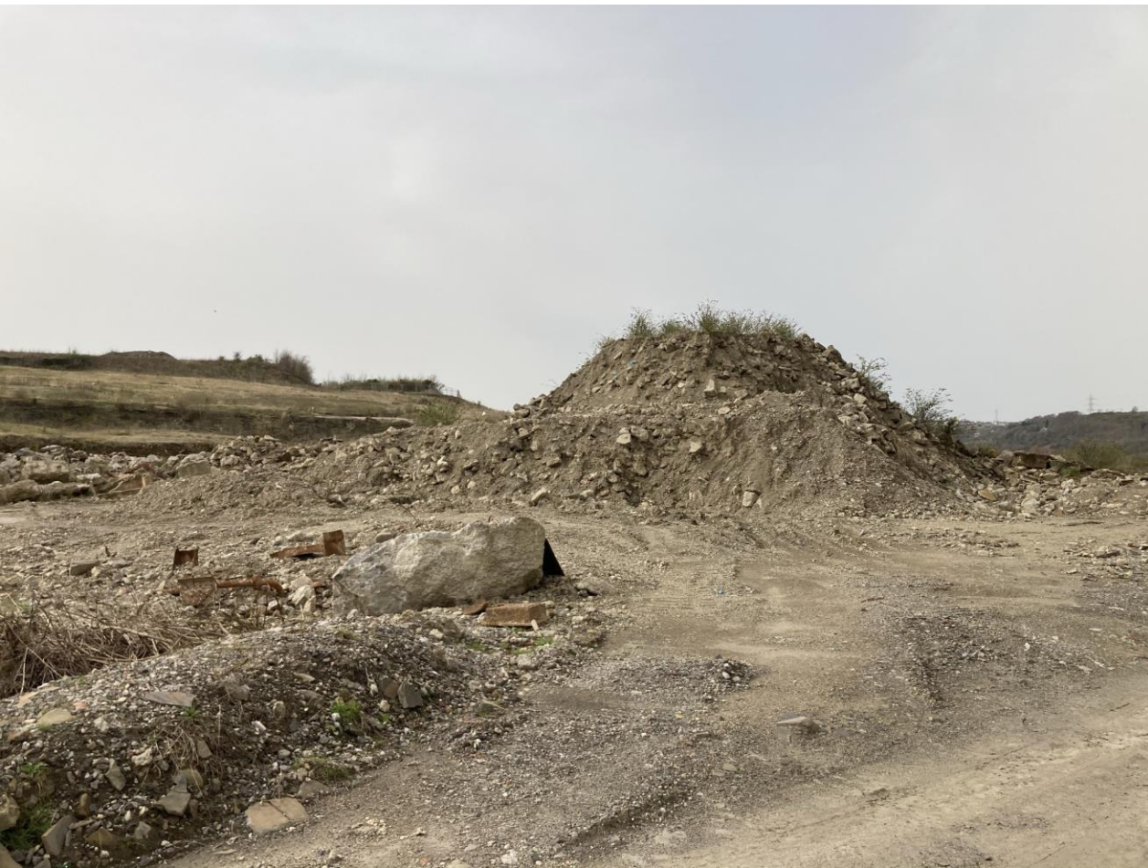
5 – Aggregate Piles in RG4
