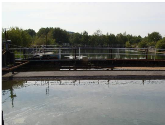
API Separators pre-remediation 3 September 2010
