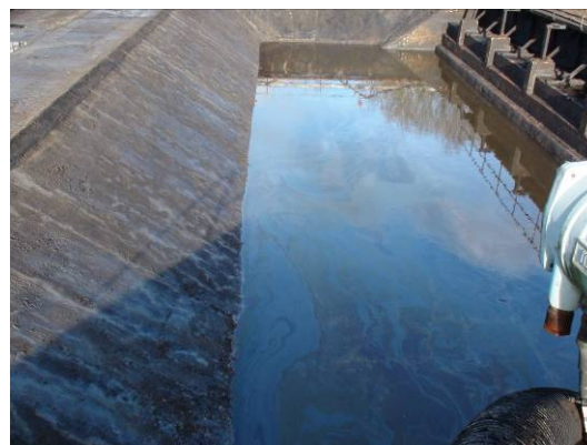
Dewatering – note hydrocarbon sheens 14 February 2011
