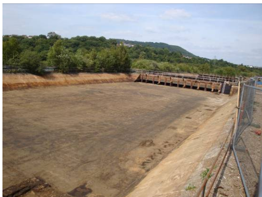
API Separators following completion of the works 4 July 2011
