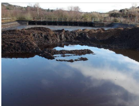
Addition of wood chippings to stabilise sludge 14 February 2011
