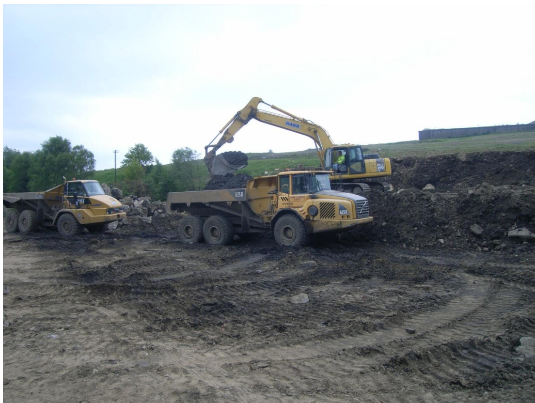
Photograph 3: Preparation of Treatment pad
