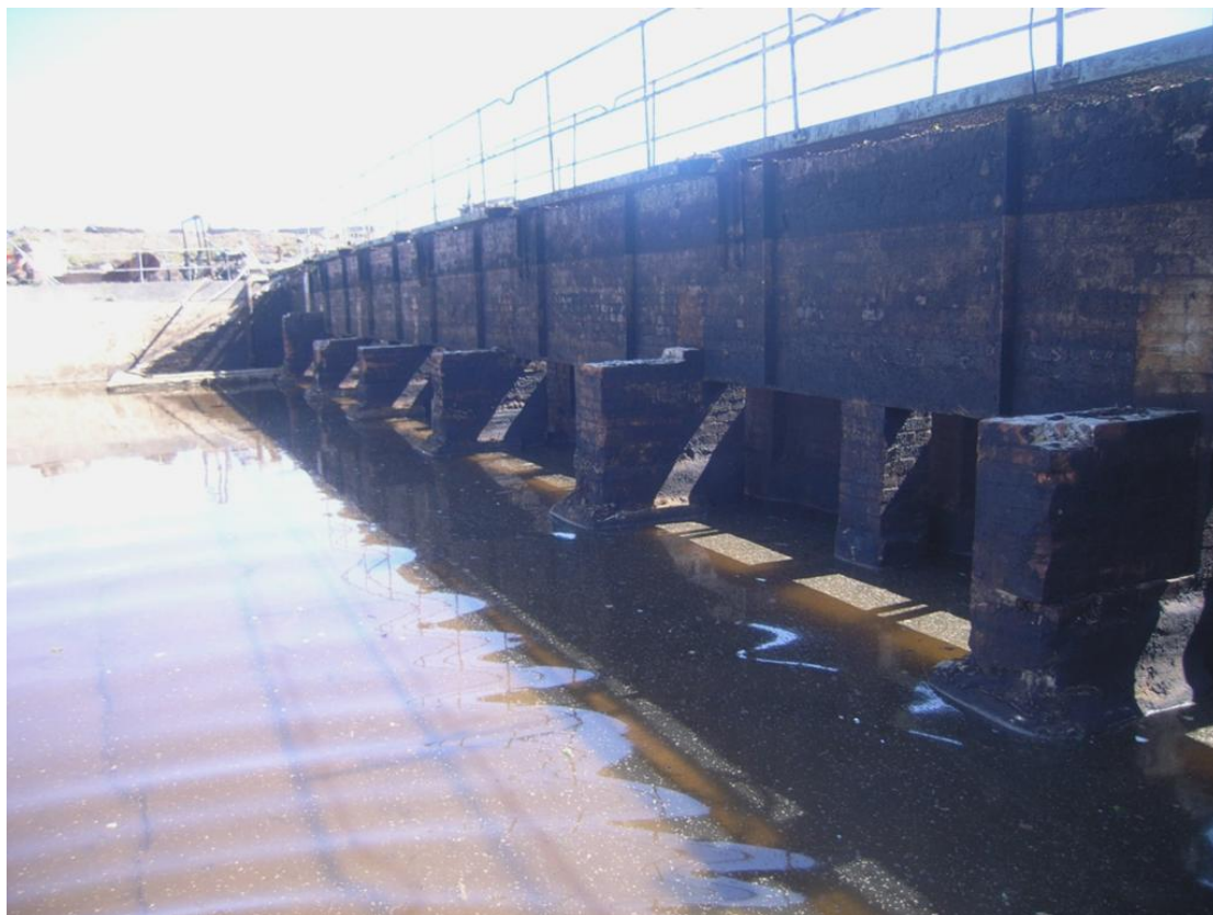
Photograph 11: Chamber 4 – Post remediation
