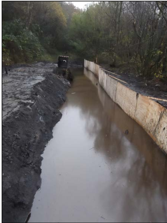
Photograph 1 – Completed trench showing boards to north (facing west)
