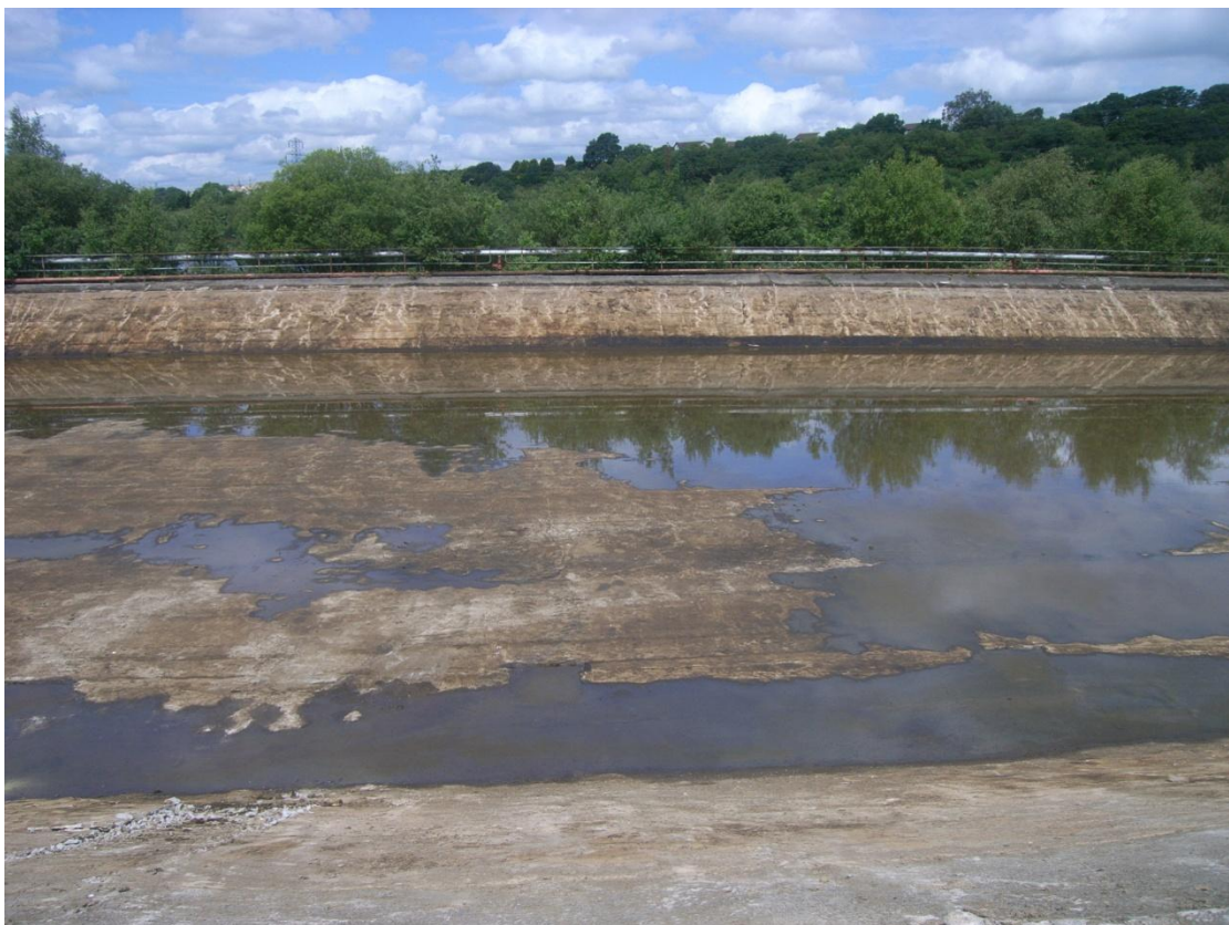
Photograph 10: Chamber 4 – Post remediation
