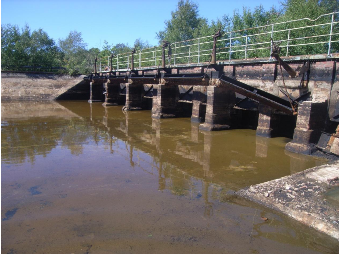
Photograph 13: Chamber 4 – Post remediation
