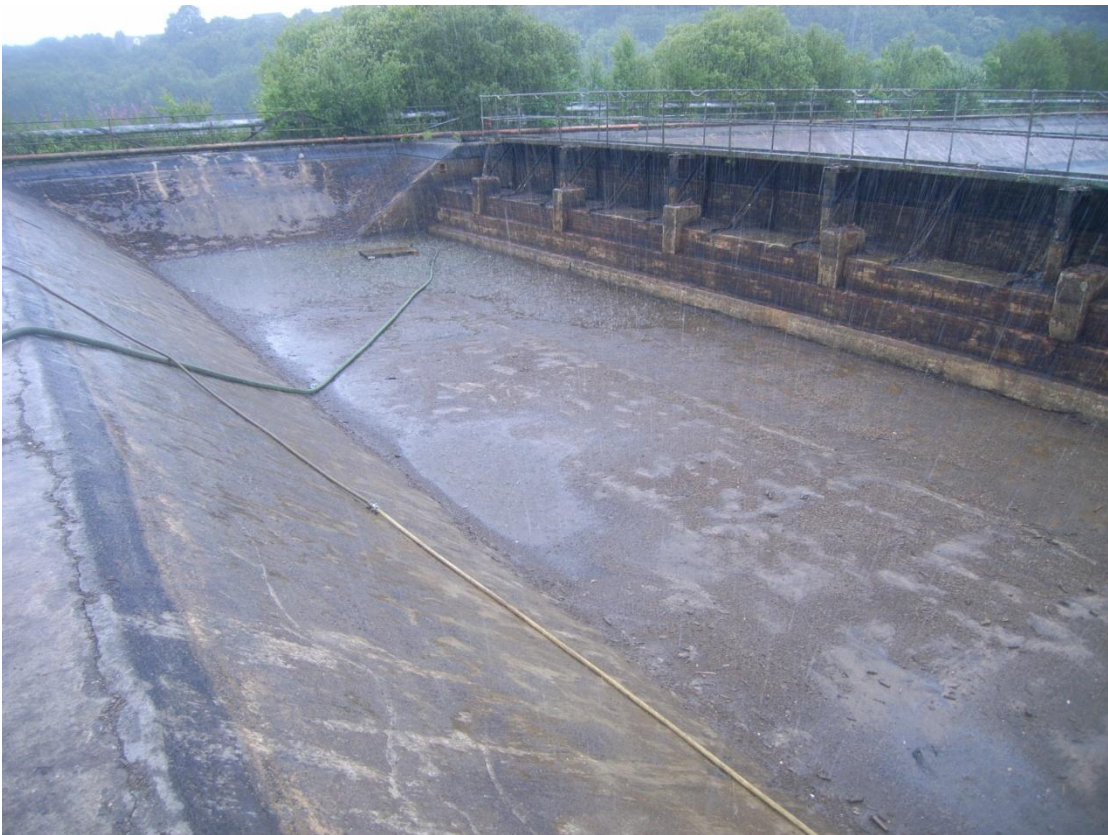
Photograph 7: Chamber 3 - Post sludge removal undergoing jet washing
