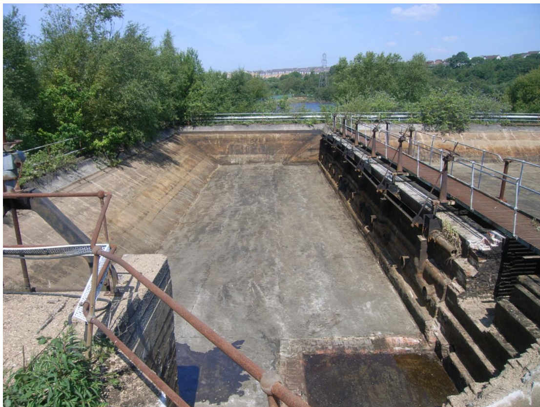
Photograph 1. Chamber 1 – Post Remediation
