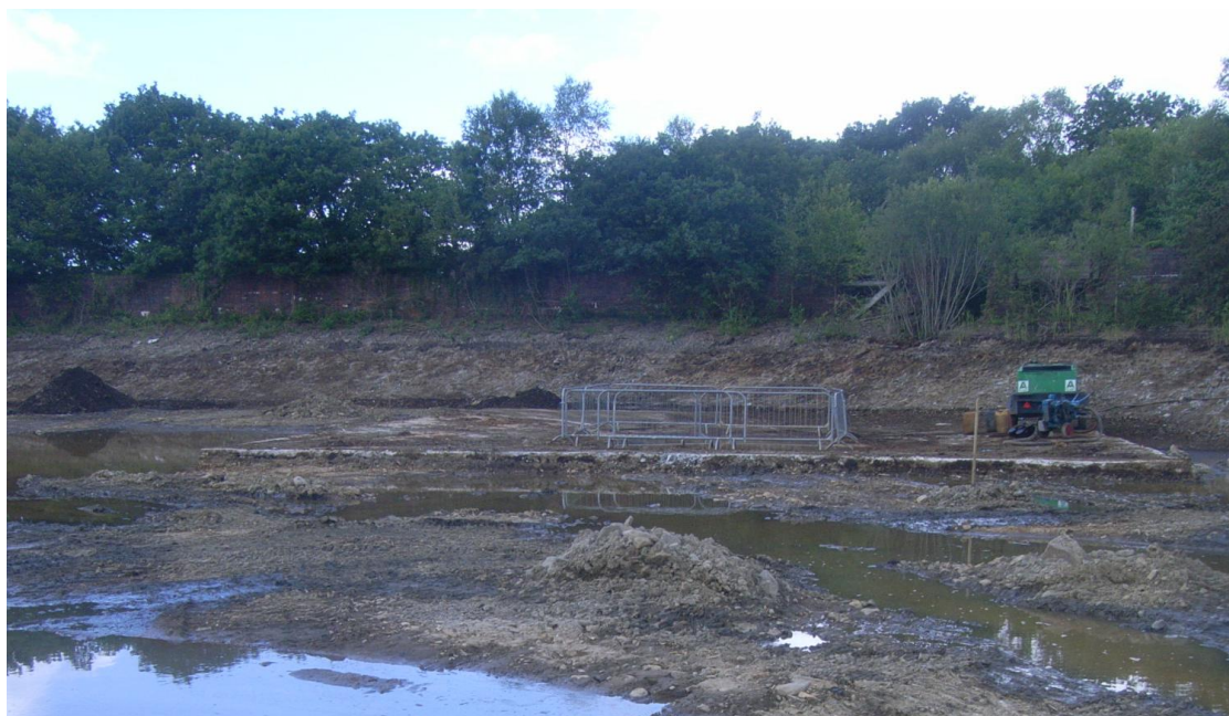
Photograph 7: Emergency draw down valve plinth
