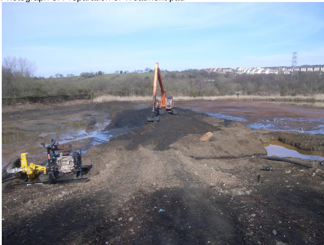
Photograph 4: Hydrocarbon impacted Sludge Stabilisation & Removal
