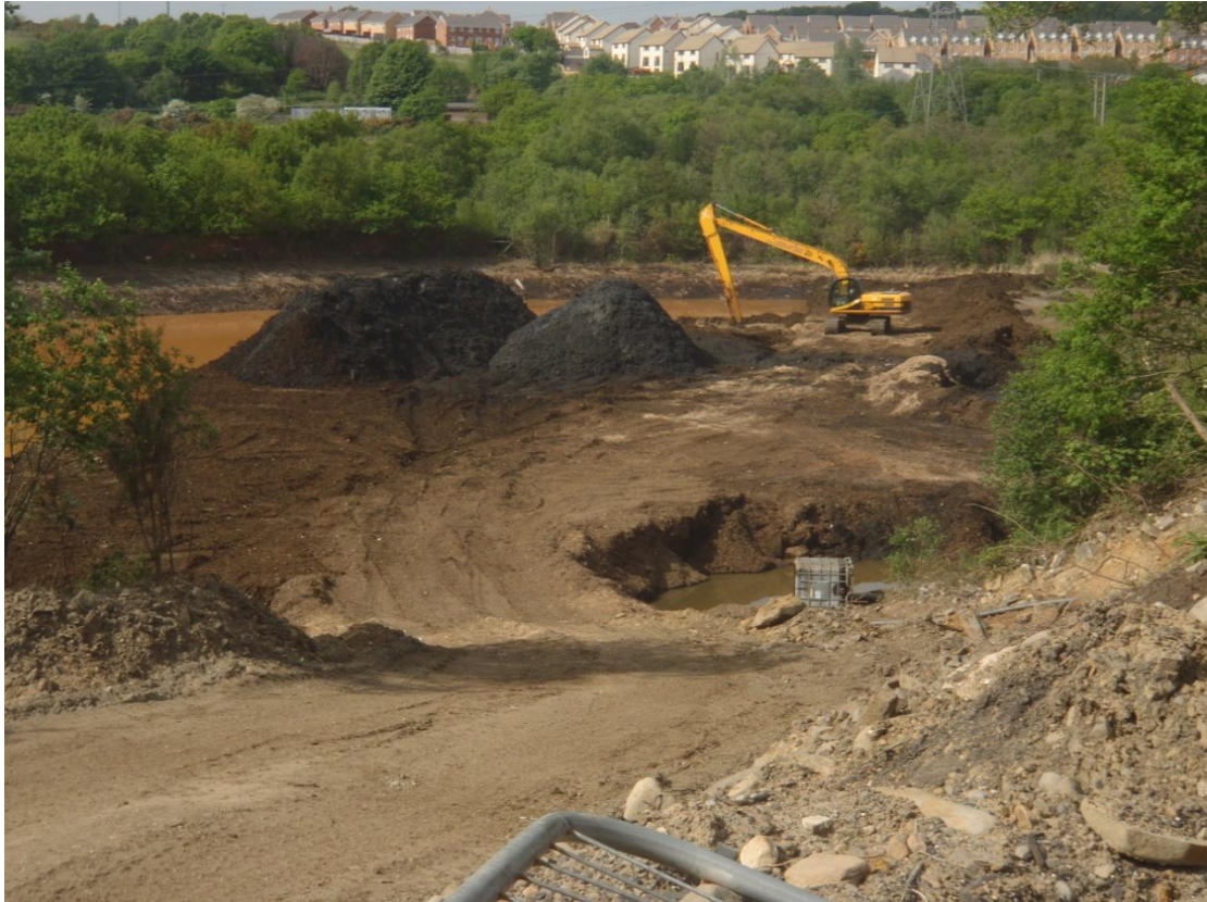
Photograph 5: Hydrocarbon impacted sludge removal
