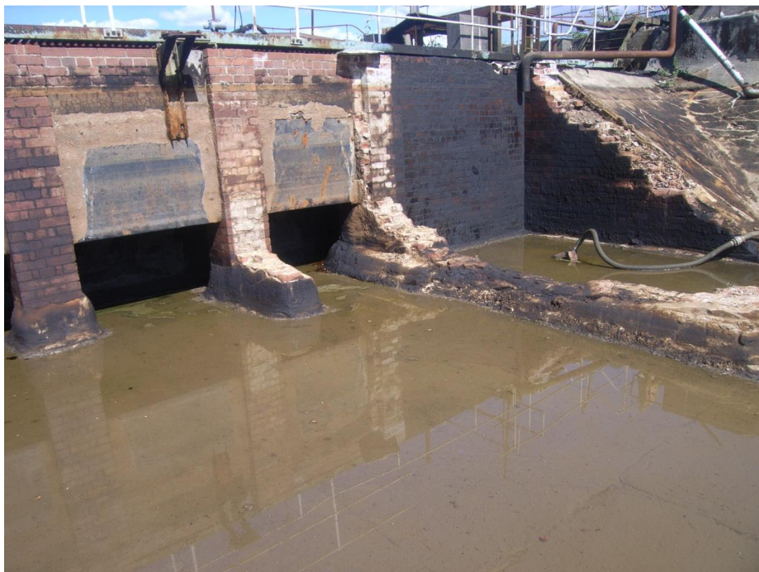
Photograph 5. Chamber 2. Post remediation with heavier staining on former oil collection sump
