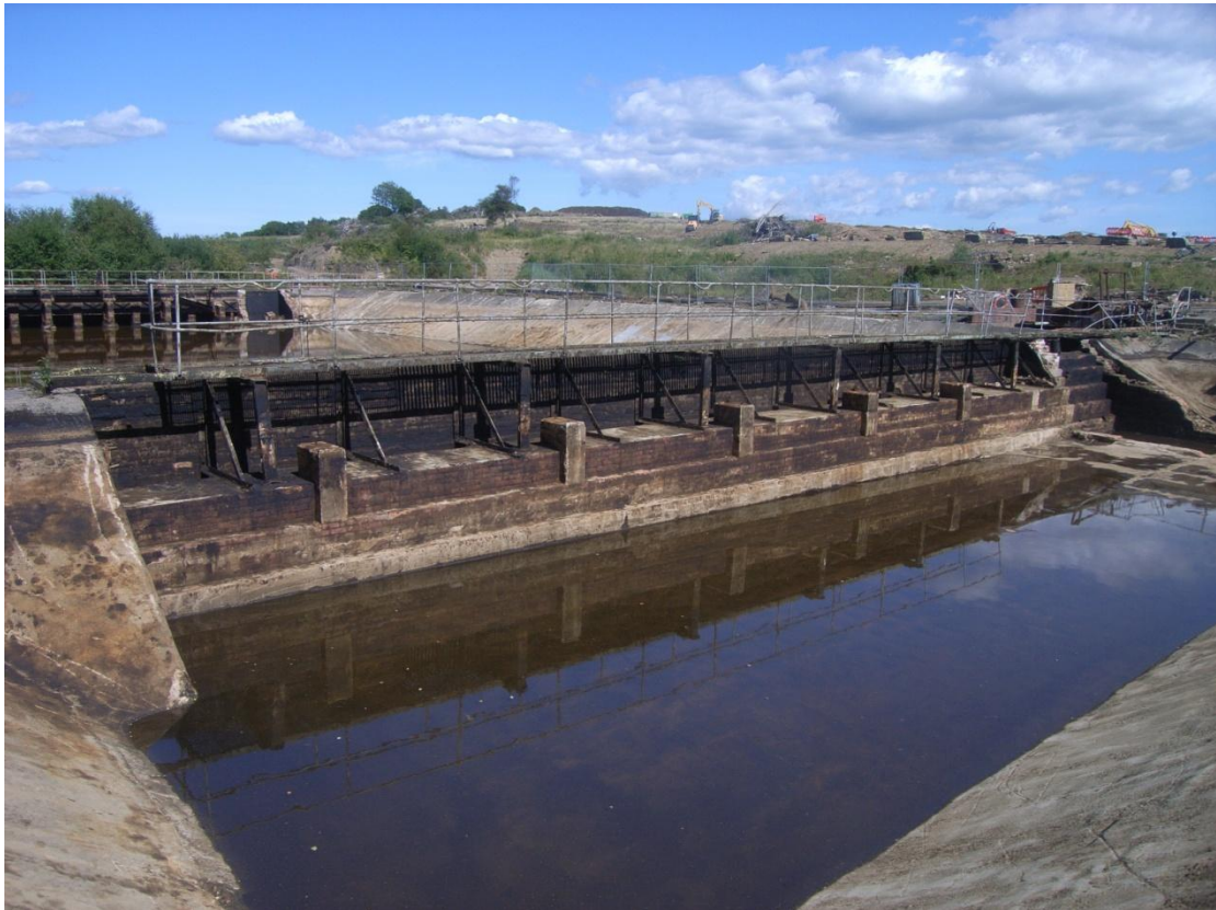
Photograph 9: Chamber 3. Post Remediation
