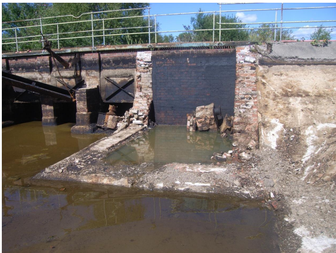
Photograph 12: Chamber 4 – Post remediation, some staining within former oil collection sump
