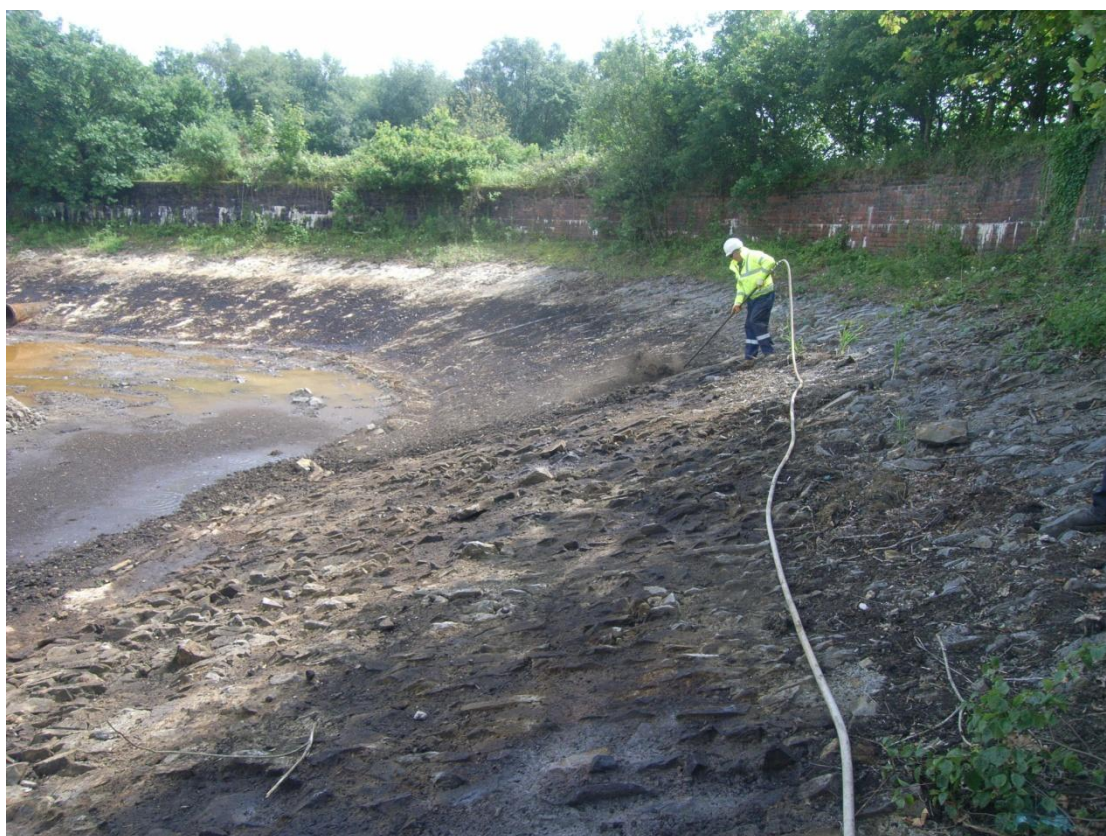
Photograph 8: Pressurised air being used to remove oil tide mark from walls
