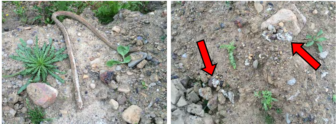
Figure Suspected AC observed within phase comprising suspected asbestos rope left and suspected fragments of asbestos right
