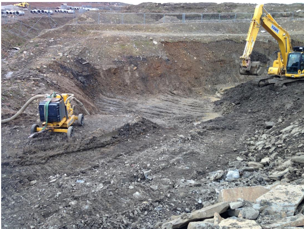
Photograph 11 – Excavation of 'Dust Lagoon'
