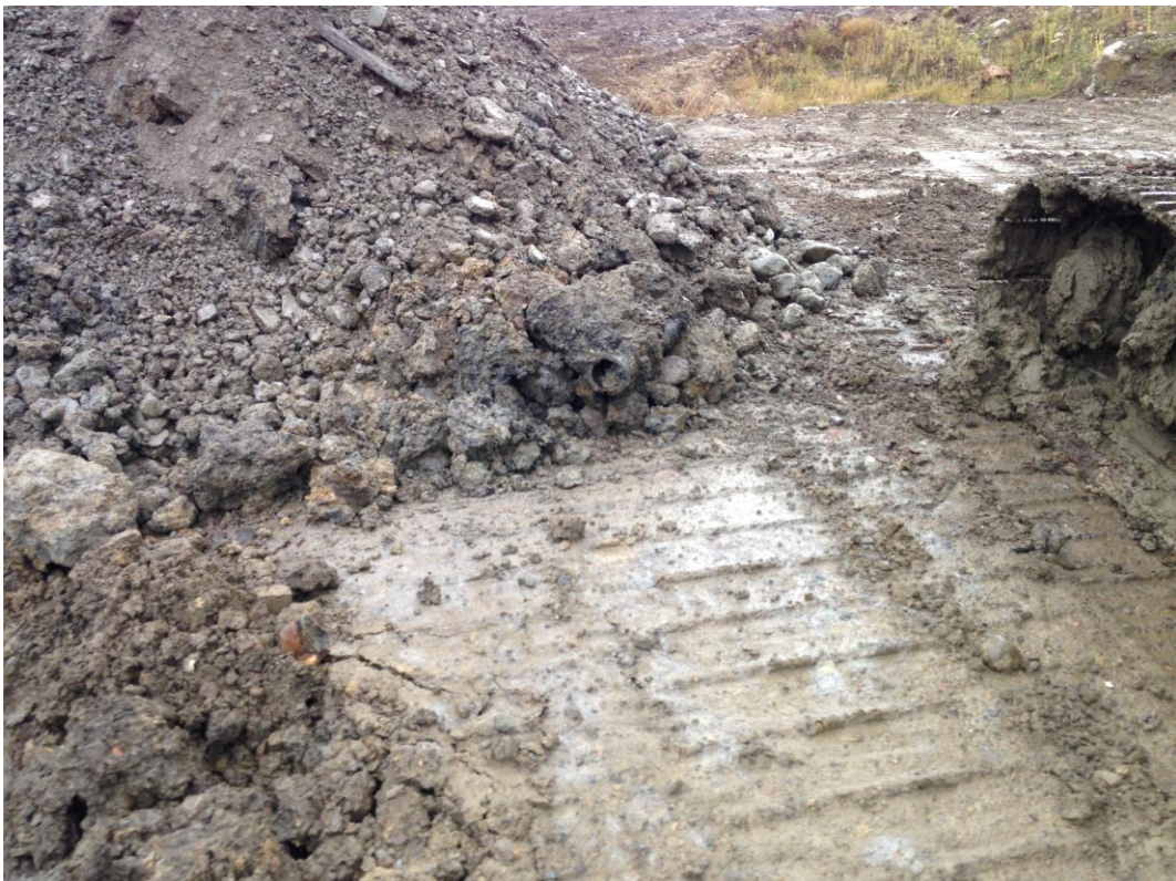
Photograph 8 – Section of pipe removed from additional excavation at IP3997
