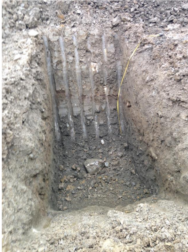
Photograph 9 – Additional excavation for VO inspection at Ip4038
