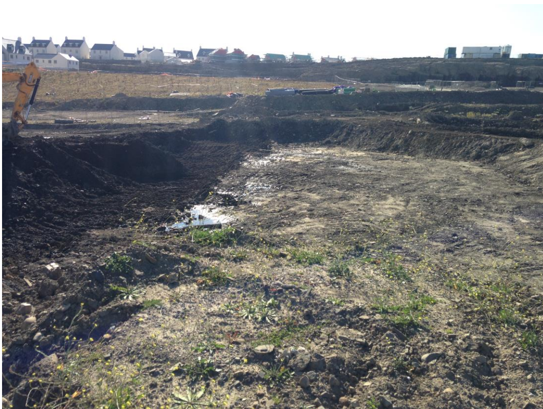
Photograph 12 – Backfill of 'Dust Lagoon'
