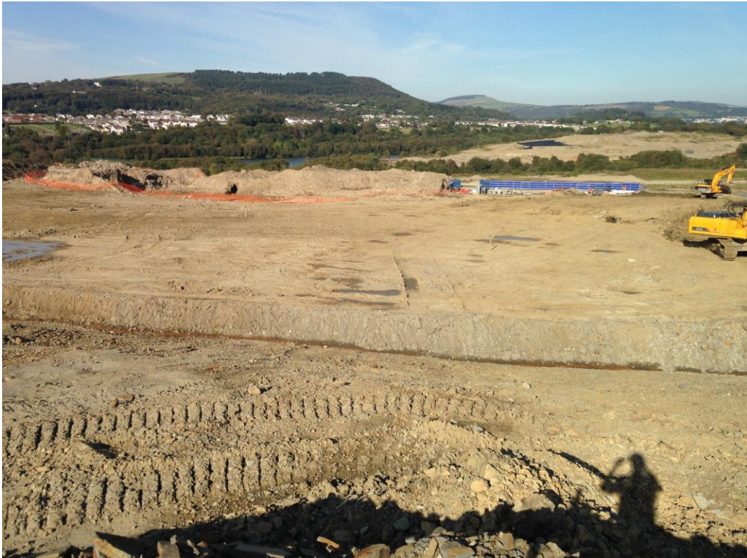
Photograph 7 – Finished levels across north west part of MP70
