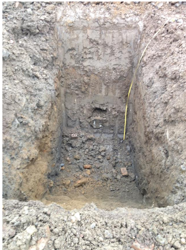
Photograph 10 – Additional excavation for VO inspection at TPE3714
