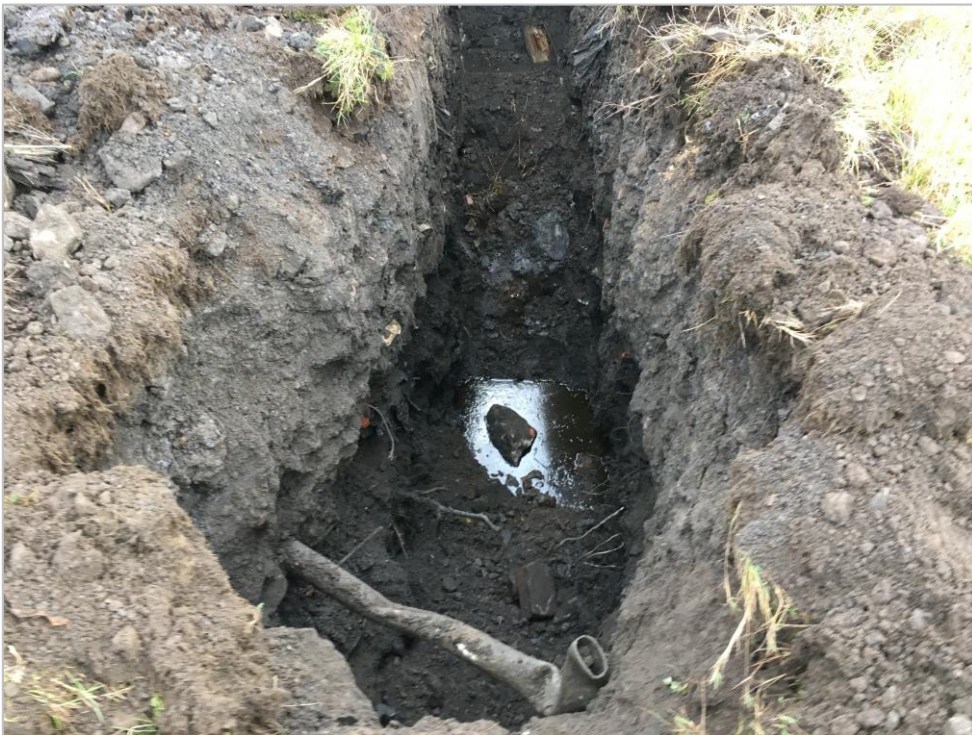
Photograph 12: TP06 excavation with visible pipework and water at base
