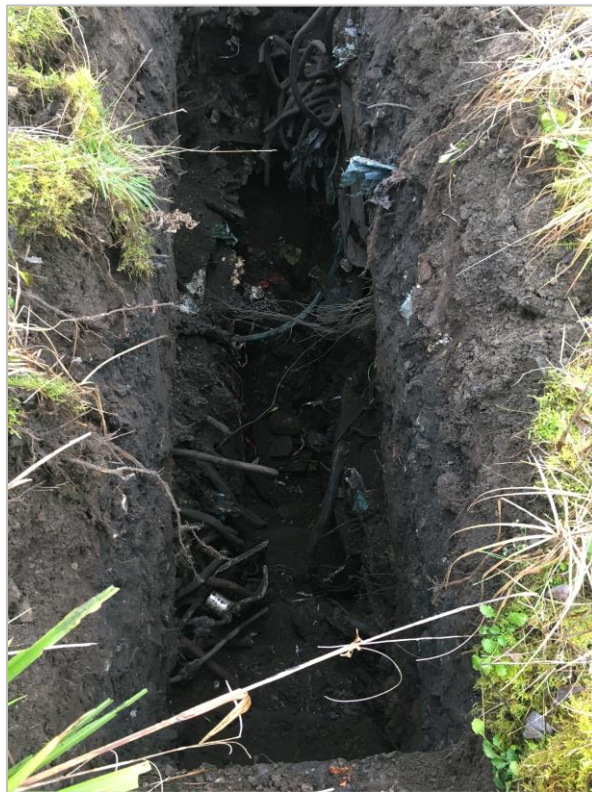
Photograph 4: TP02 Excavation with cables and pipes visible
