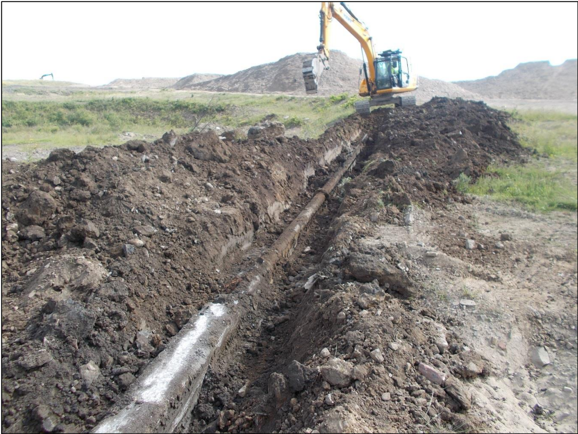
Photograph 5 TPE1254 – Part of pipe network encountered and removed from Monitor Phase 58
