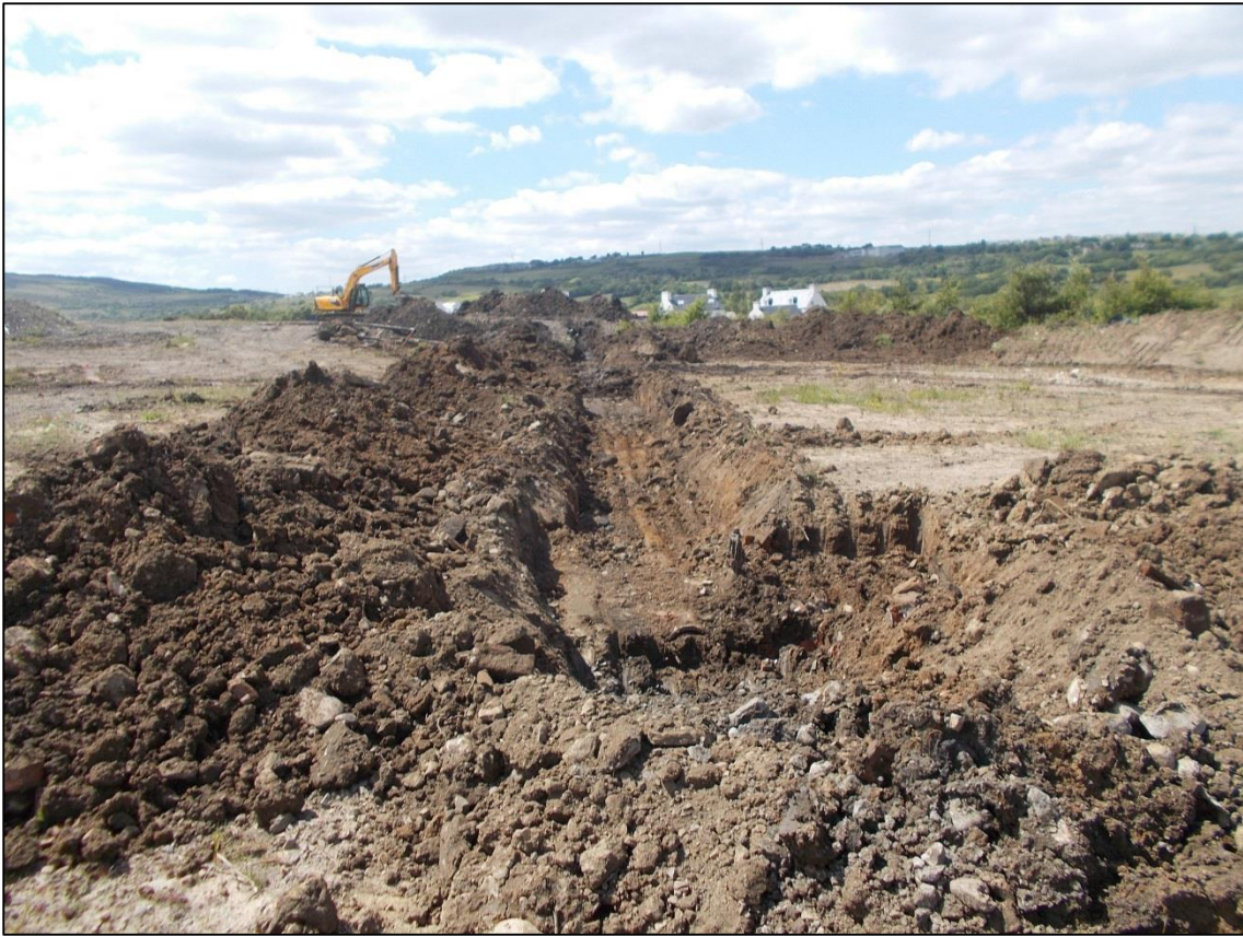
Photograph 3 IP2501 – Part of pipe network encountered and removed from Monitor Phase 58
