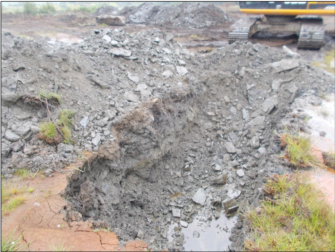
Photograph 2 IP2404 – No evidence of free product in excavation
