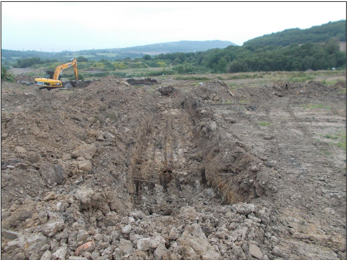
Photograph 4 TPE1175 – Part of pipe network encountered and removed from Monitor Phase 58
