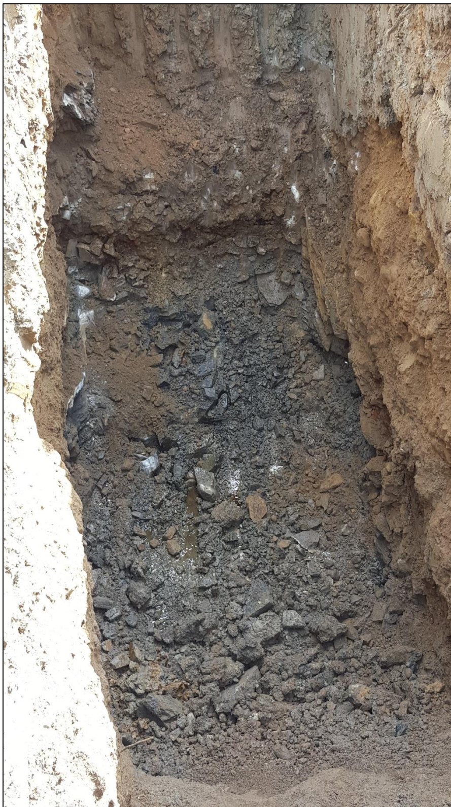
Photograph 1 TPE2687 – Minor free product at base of trial pit
