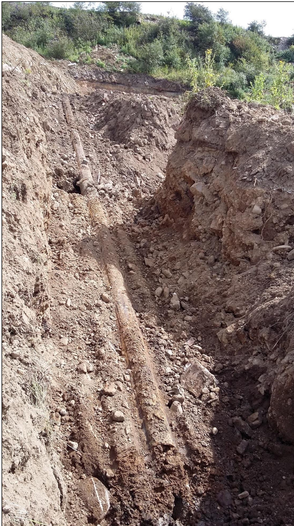
Photograph 5 TPE2676 – Section of pipework to be removed from excavation
