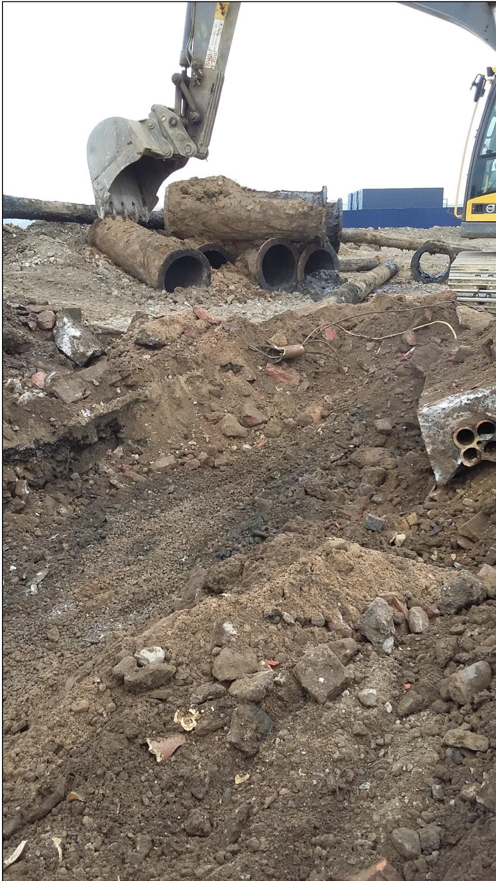
Photograph 6 TPE2820 – Metal and clay pipework removed from excavation
