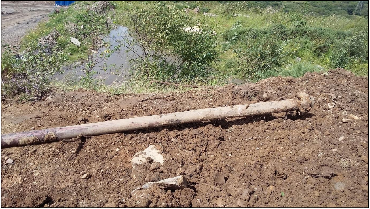
Photograph 7 TPE2999 – Section of metal pipe removed from excavation
